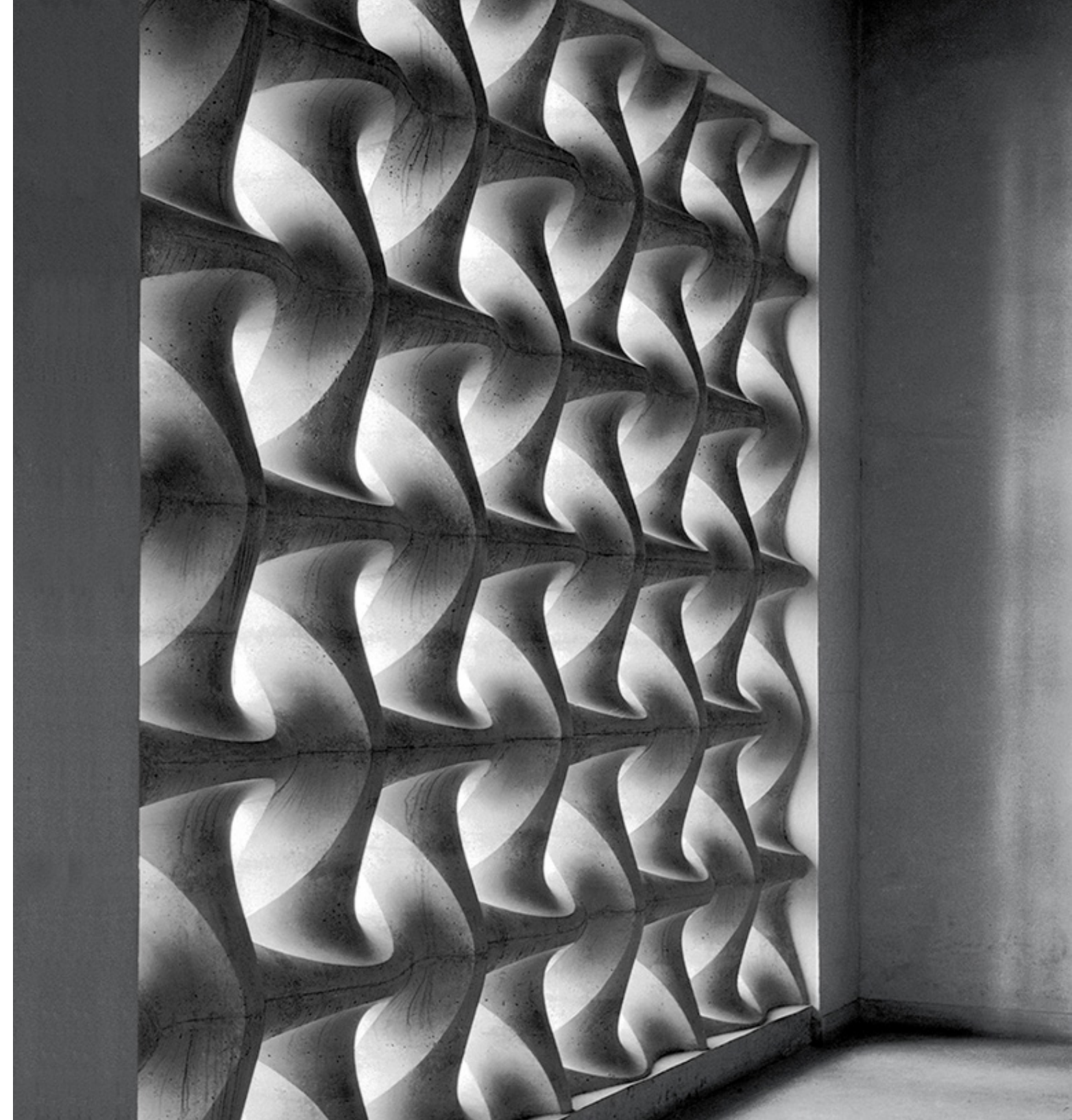
Figure 2.4.1 ‘Continua’ Screen, ‘Design 2’ by Erwin Hauer. Cast Hydrostone. Pfarre Liesing Church, Austria, 1951.
