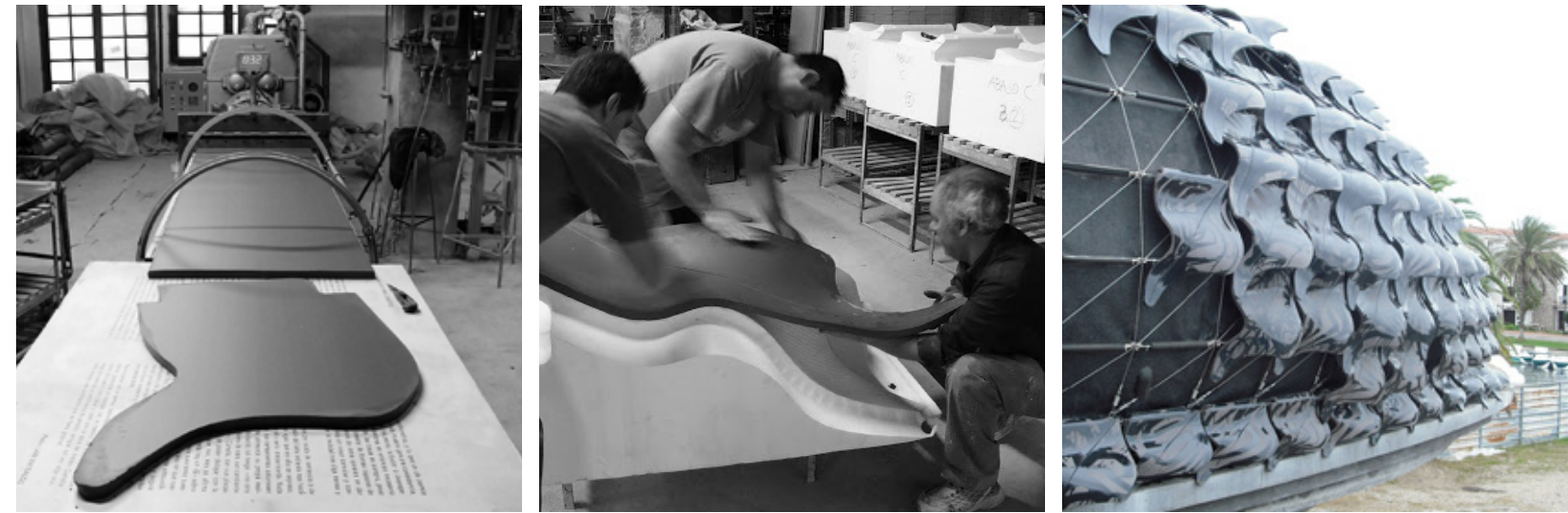
Figure 2.3.1 Slump moulded building system at Villa Nurbs by CLOUD 9.
