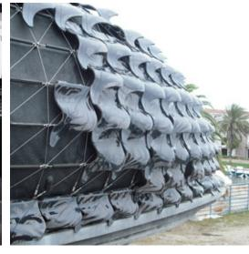
Figure 2.3.1 Slump moulded building system at Villa Nurbs by CLOUD 9.
