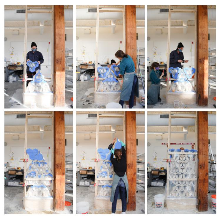
Figure 5.3.2 HIVE prototype assembly process.
