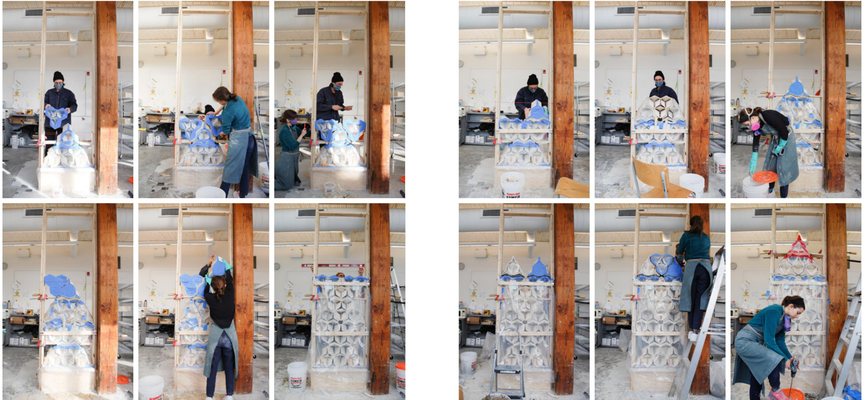
Figure 5.3.2 HIVE prototype assembly process.
