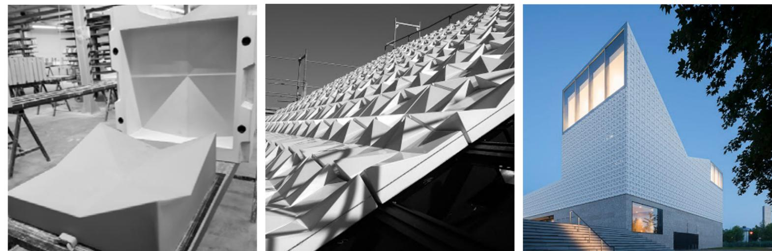
Figure 2.3.3 Slip cast building system at Saint Rupert Church by Meck Arkitekten.
