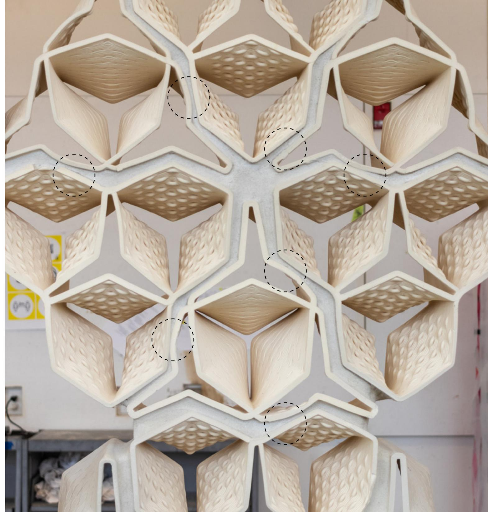
**Figure 5.3.4** Detail of HIVE prototype highlighting dimensional inconsistencies across mortar joints.
