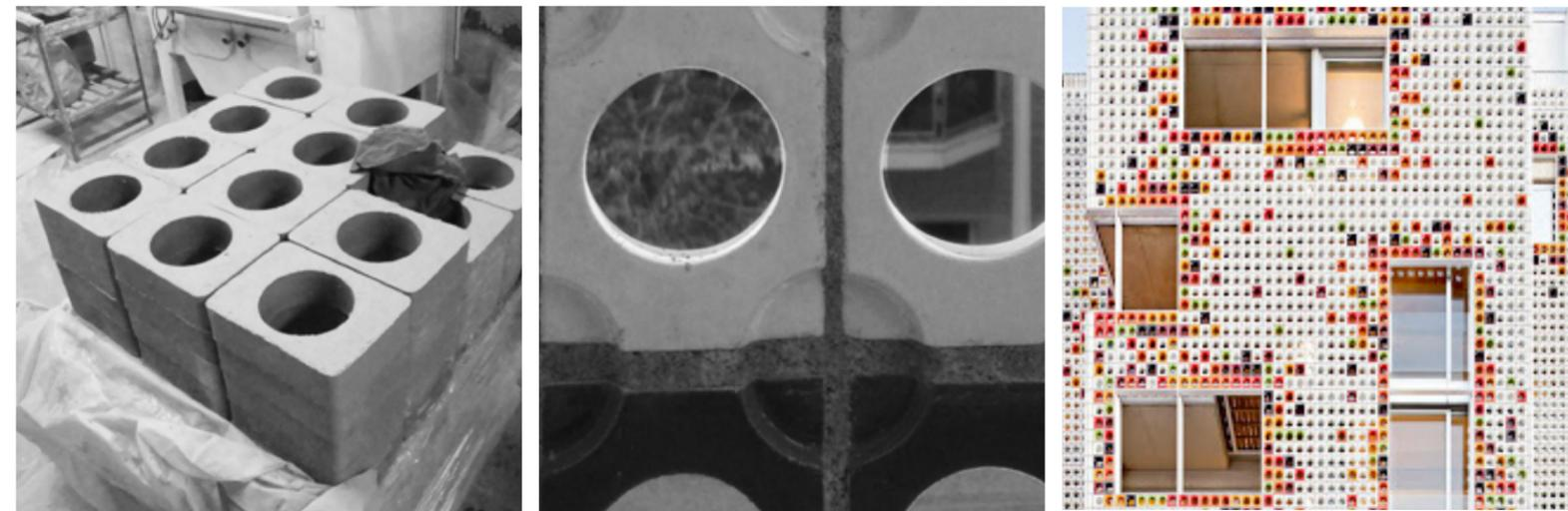
Figure 2.3.2 Plastic pressed building system at Badalona Apartments by Lagula Architects.
