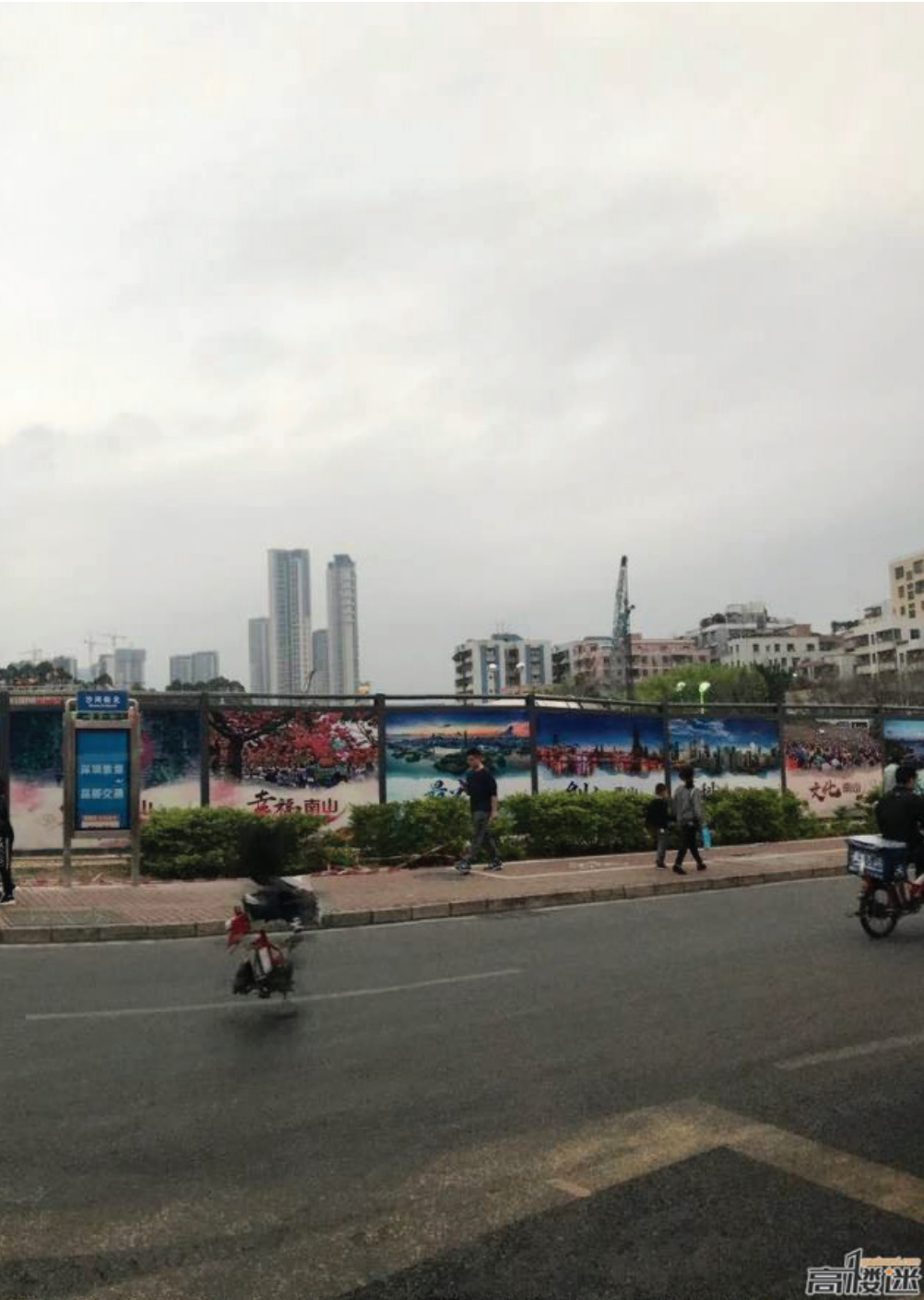
Fig.3.4 | Construction Site at Baishizhou
