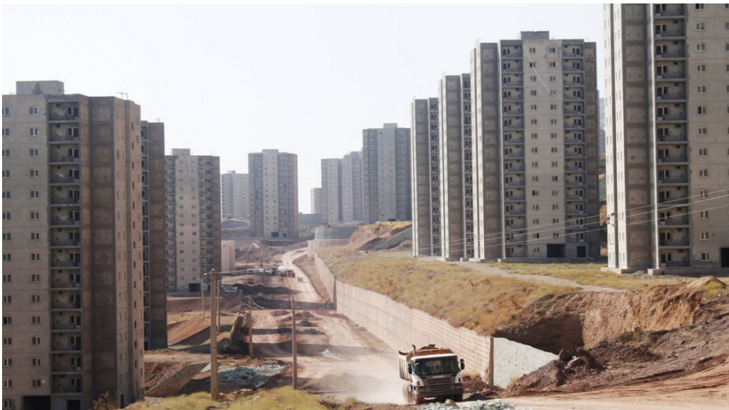
Fig. 1.24 Long retaining walls along the neighborhood
