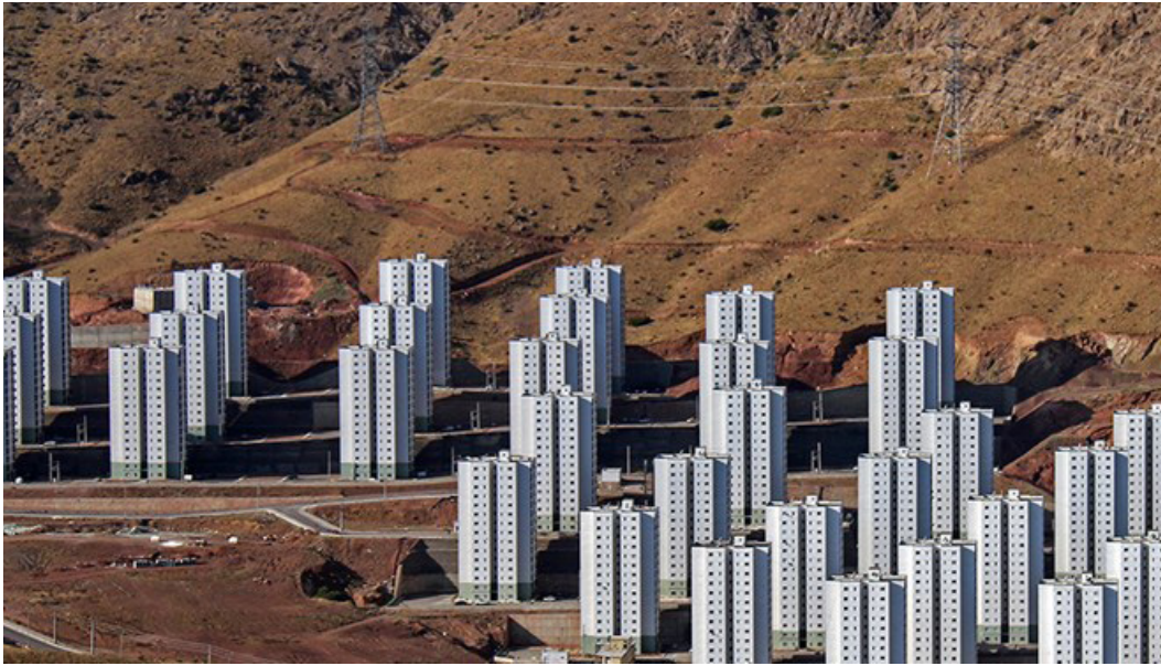
Fig. 1.22 Residential towers in phase 11 under construction
