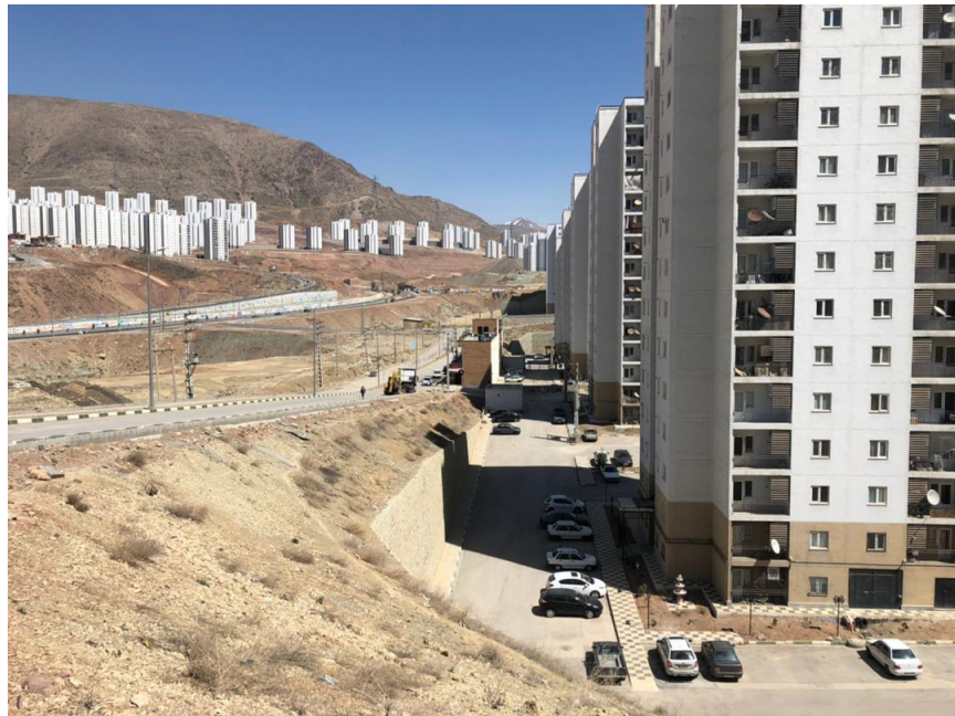
Fig. 3.12 Dangerous shortcut made to reach the main street
