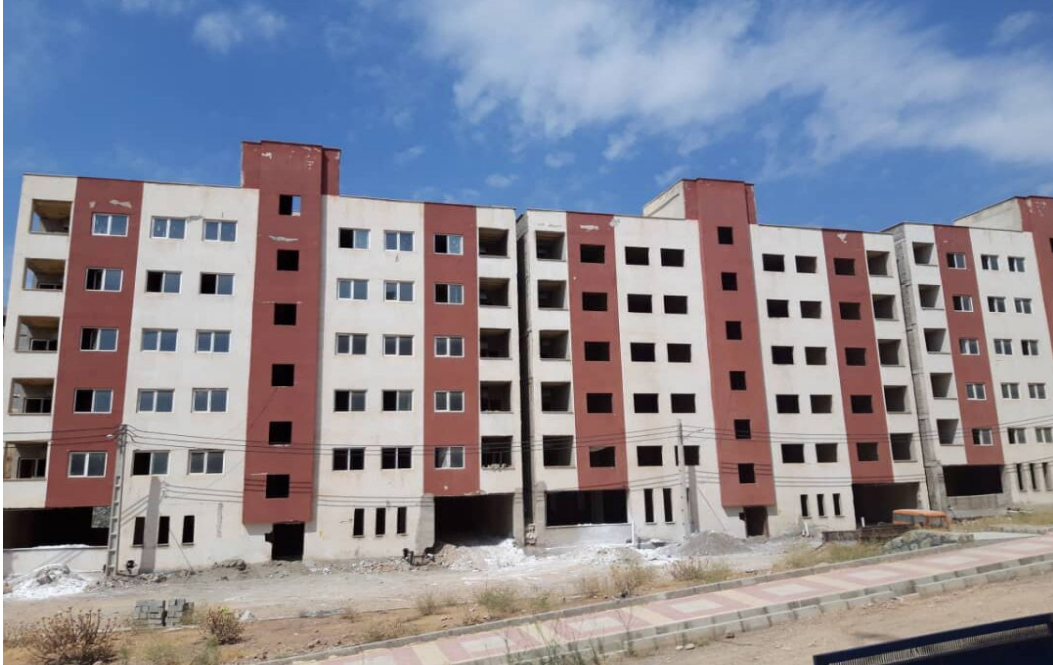
Fig. 1.16 Mehr housing in Hashgerd new town
