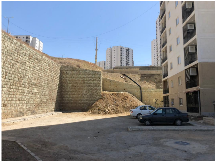
Fig. 3.9 9-meter high retaining wall
