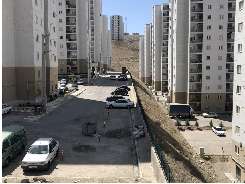
Fig. 3.8 Retaining wall along the site
