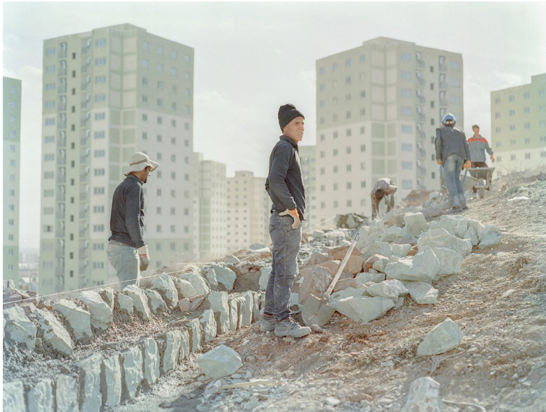
Fig. 1.28 Laborers in Pardis construction
