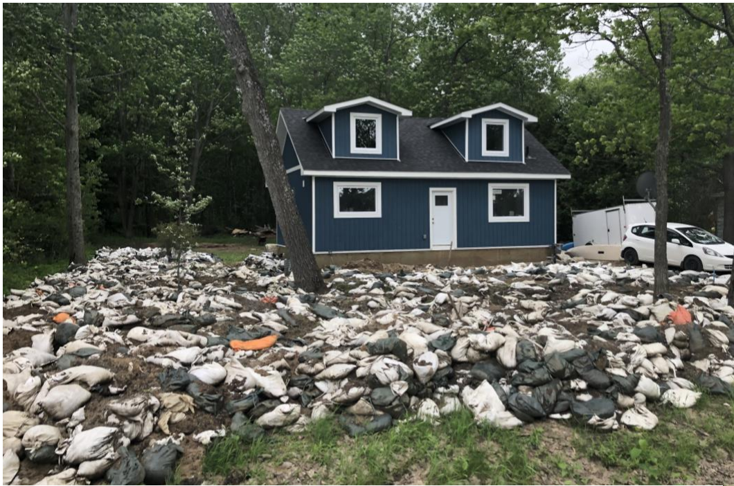
Figure 4: A property in Constance Bay, ON is surrounded by sandbags to protect it from the flooded banks of the Ottawa River (Cottar, 2019).
