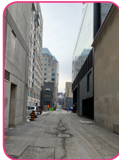
Fig. 33 - Mixed-Use/Commercial Laneway; 2019, photo
