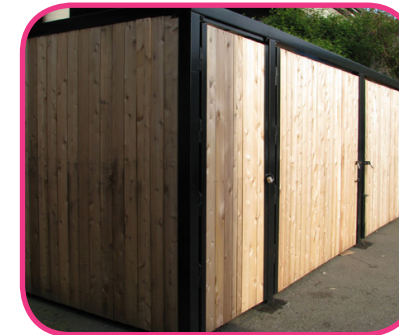
Fig. 182 - Garbage Enclosure, photo
