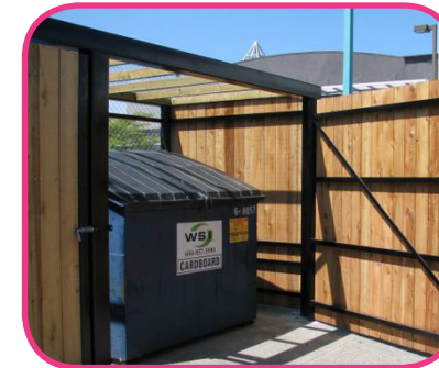
Fig. 183 - Garbage Enclosure, photo
