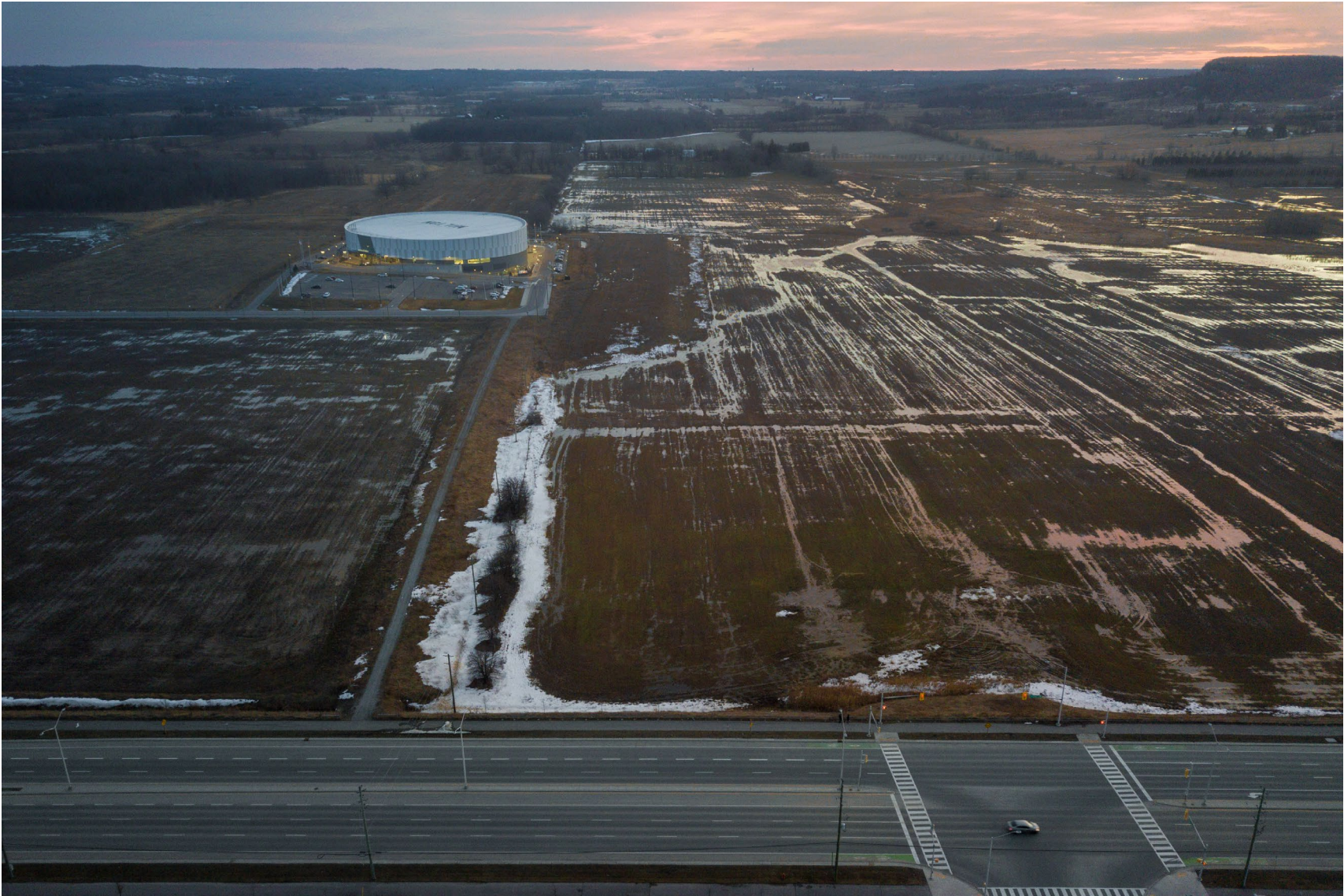
fig. 3 Aerial Photo of the Mattamy National Cycling Centre, Milton
