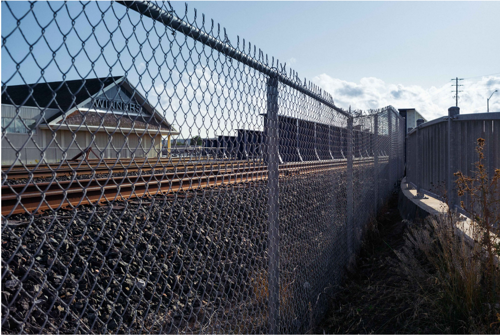
Junction between the rail and Main St. underpass fig. 32
