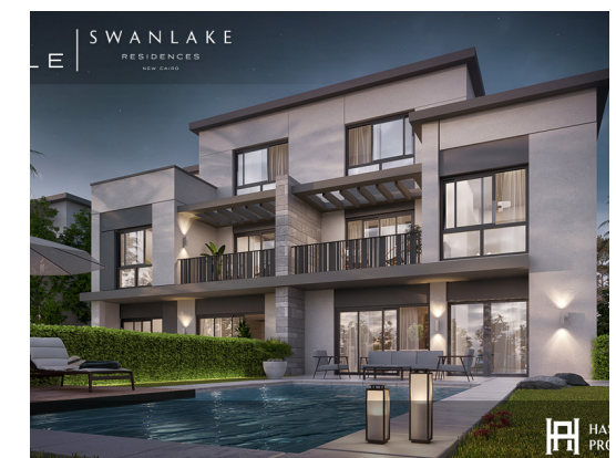
Figure 2.16: A House in Swan Lake Compound in New Cairo, a Second Generation Satellite City
