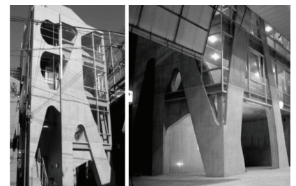
[figure 2.1.6] Akutagawa Riverside Building
