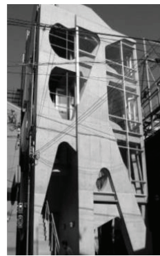
Akutagawa Riverside Building in Osaka, Japan
