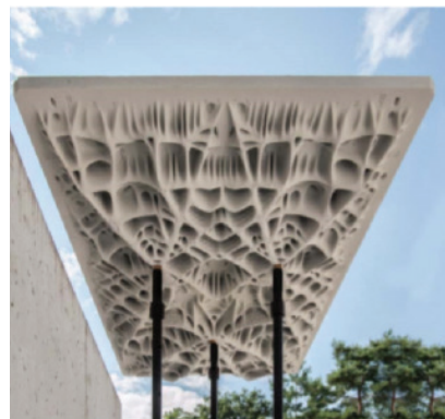
[figure 2.1.8] 3D-Printed Stay-in-Place Formwork by ETH Zurich
