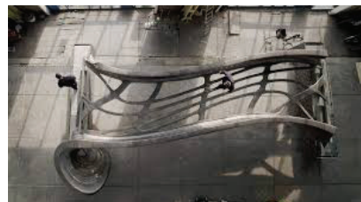
[figure 2.1.12] 3D Printed Bridge by MX3D
