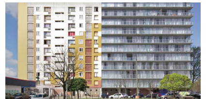
[figure 2.2.1] Before and After Construction of Exoskeleton Facade of Tour Bois le Pretre in Paris
