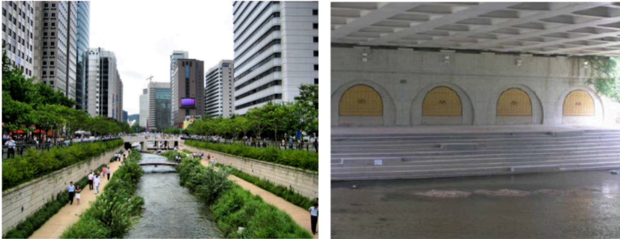
Figure 13. The Cheonggyecheon Stream: The right image depicts its naturalized stream design and the left image displays its stormwater overflow conduits (Green, 2014; Anzola, 2007)
