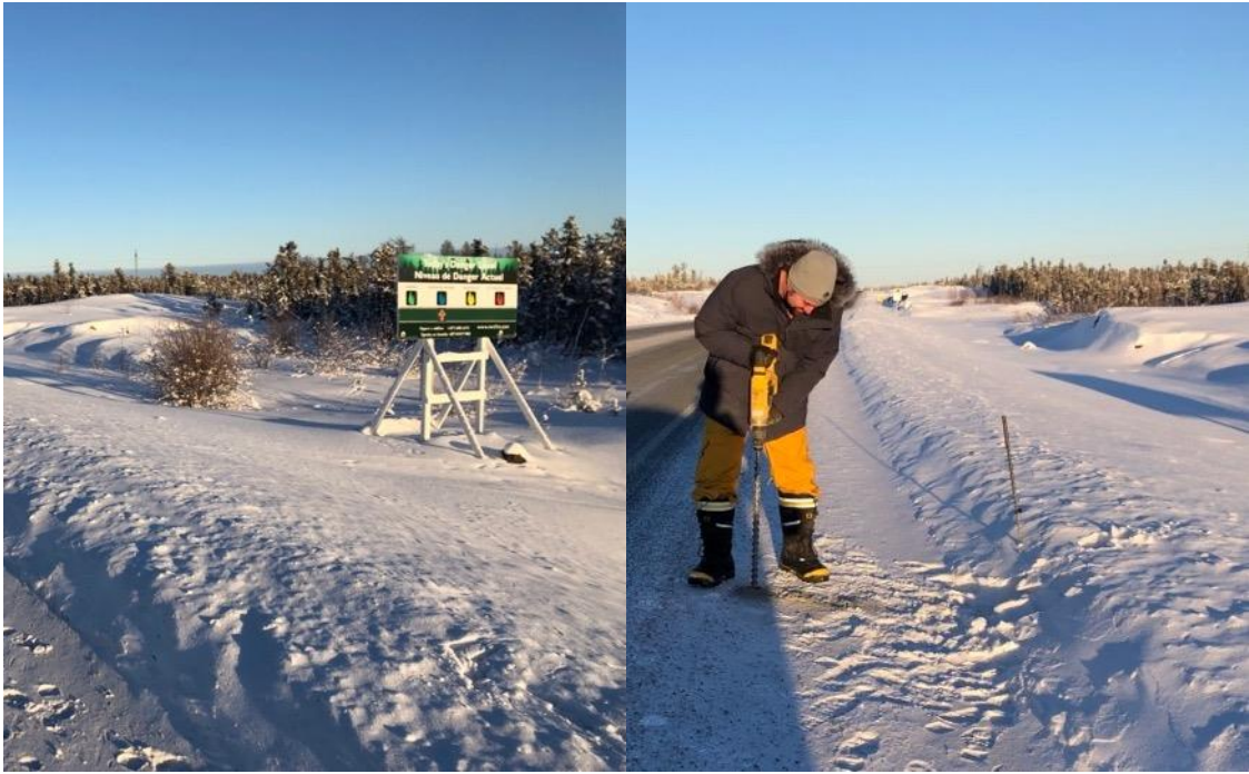
Thermistor string 3 location/installation
