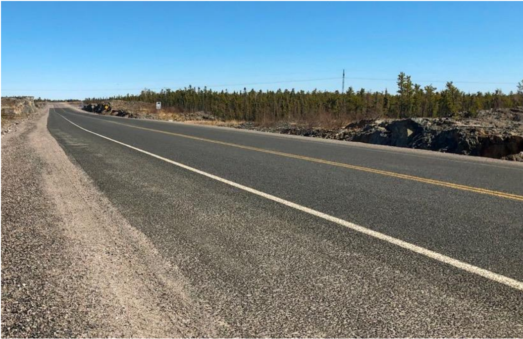
Chipseal section near sensors #3 and #4. Taken May 24, 2019.
