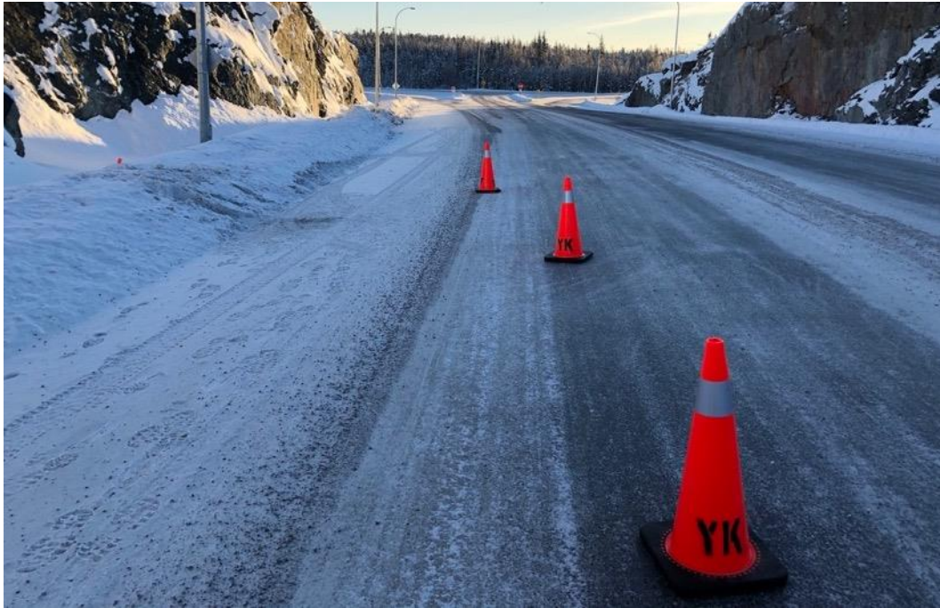
Asphalt section near sensors #1-#4. Taken January 18, 2019.
