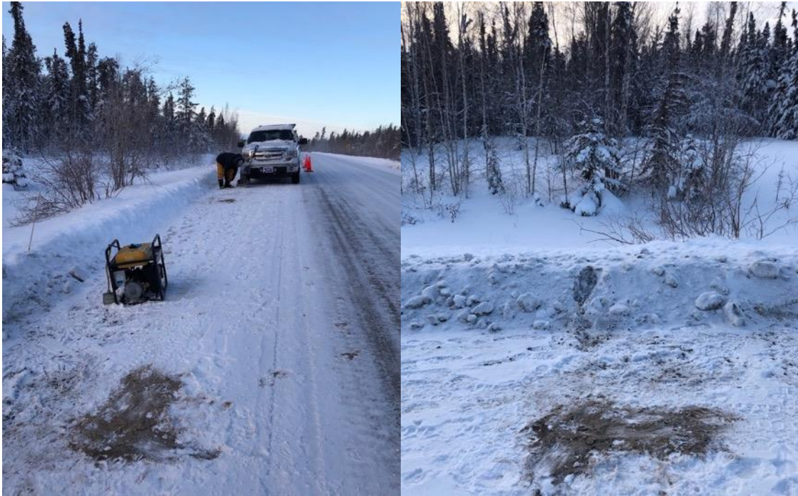
Thermistor string 9 location/installation
