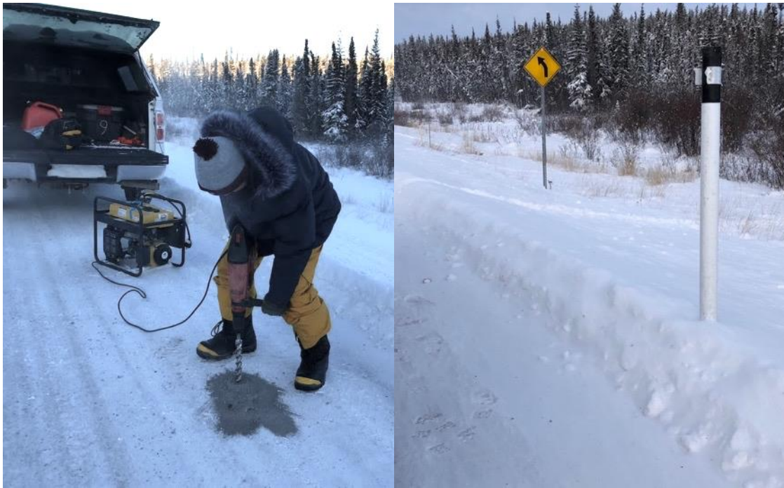
Thermistor string 5 location/installation
