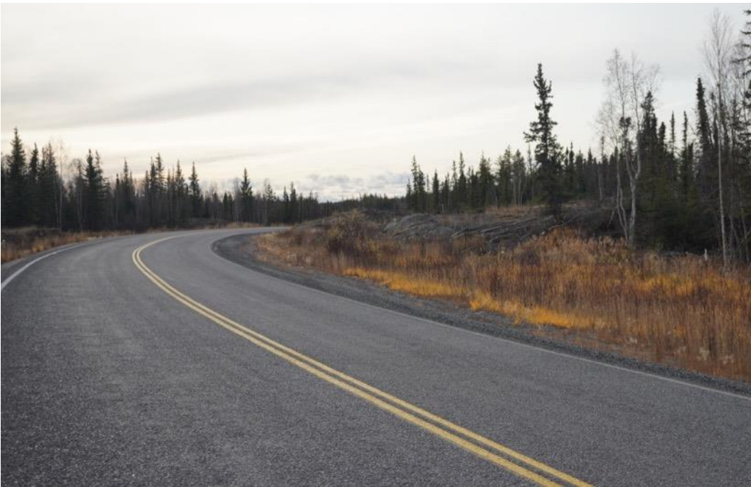
Chipseal section near sensors near sensors #3-#4 and Ptarmigan Mine. Taken October 7, 2019.
