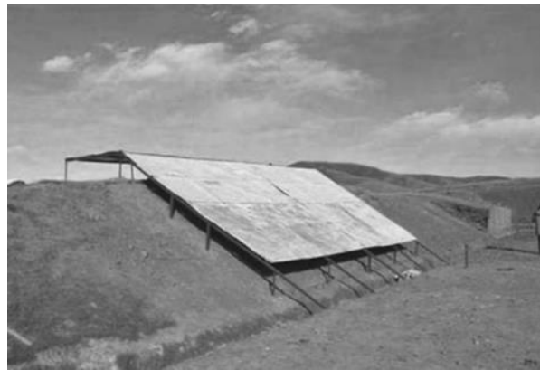
Figure 4.5. Shading panels installed along the Qinghai-Tibet Highway in China (Doré & Zubeck, 2009)
