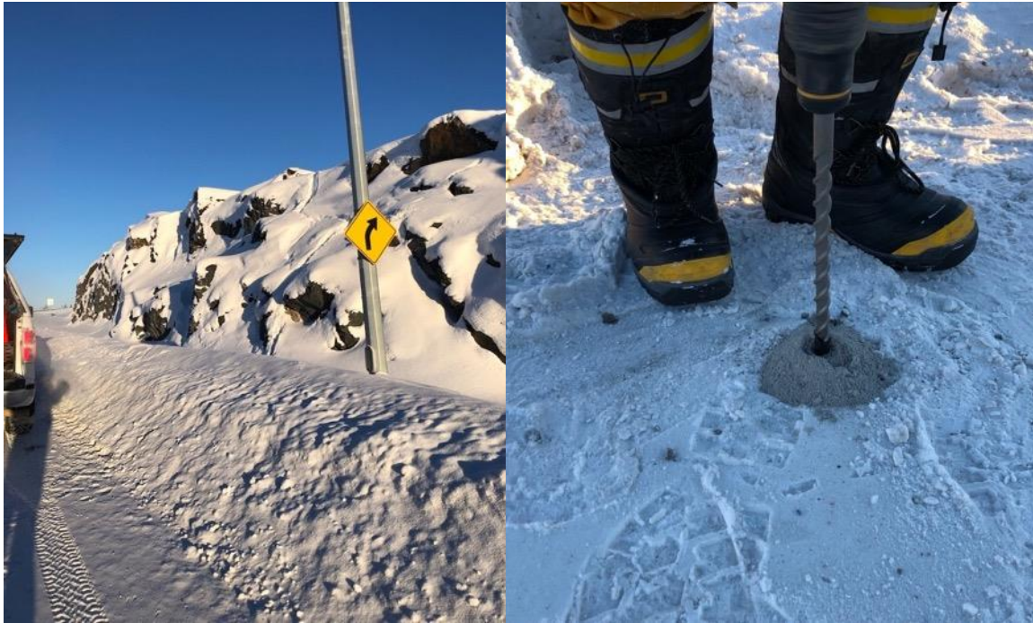
Thermistor string 1 location/installation
