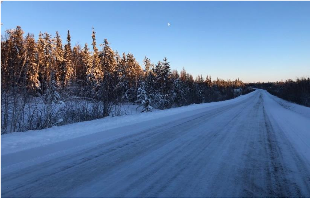
Chipseal section near sensors #5 and #6. Taken January 16, 2019.
