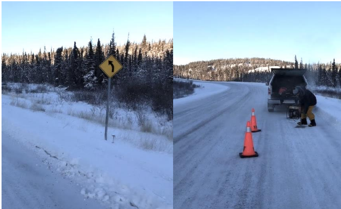
Thermistor string 6 location/installation
