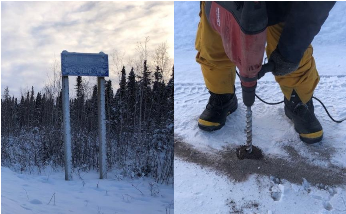
Thermistor string 10 location/installation
