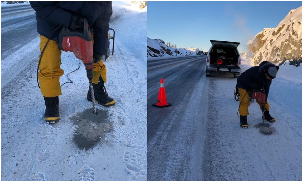
Thermistor string 2 location/installation
