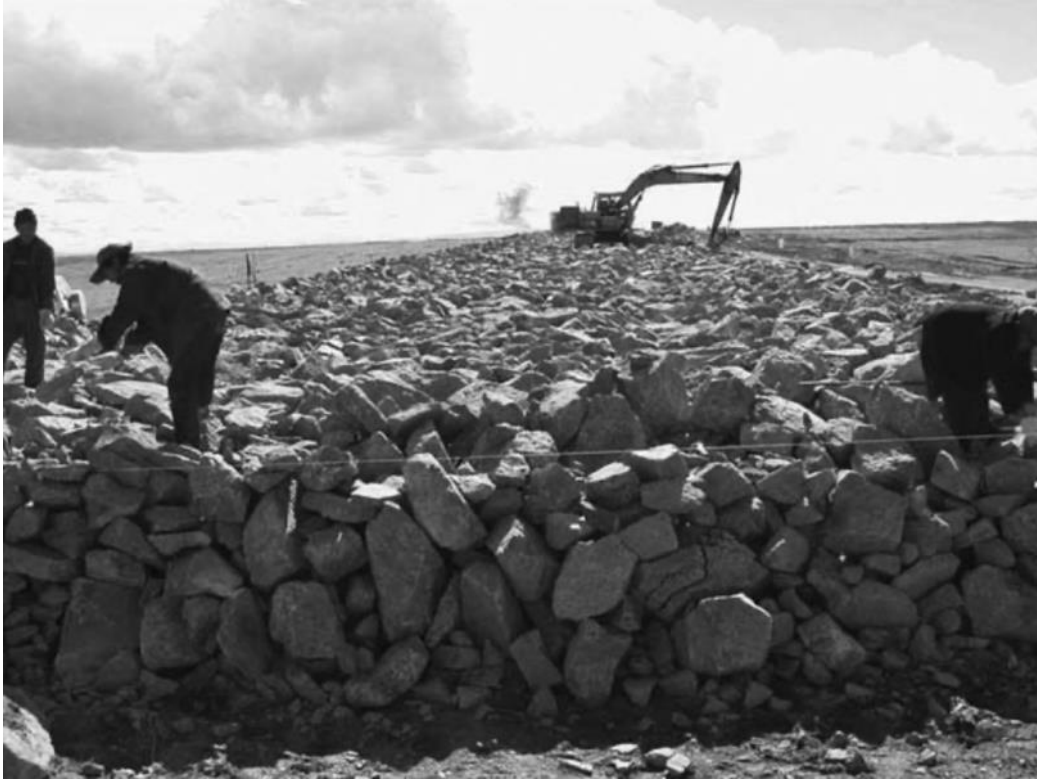
Figure 4.15. ACE installation along the QTH (Luo, Niu, Liu, Lin, & Yin, 2018).
