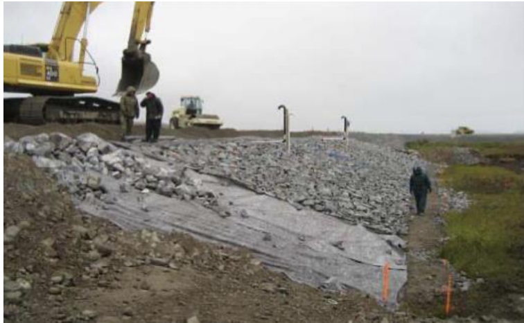
Figure 4.16. Geotextile being installed on side slope in Nunavik, Québec (Jørgensen & Doré, 2009).
