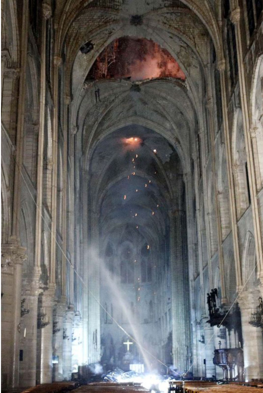
Figure 4.5 - Vault Collapse Notre-Dame - Photo by Amaury Blin
