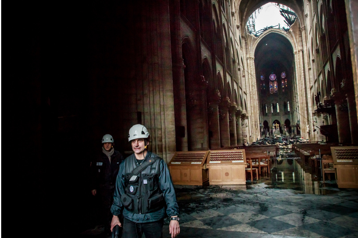
Figure 4.7 - Below collapsed vaults - Photo by Christophe Petit Tesson
