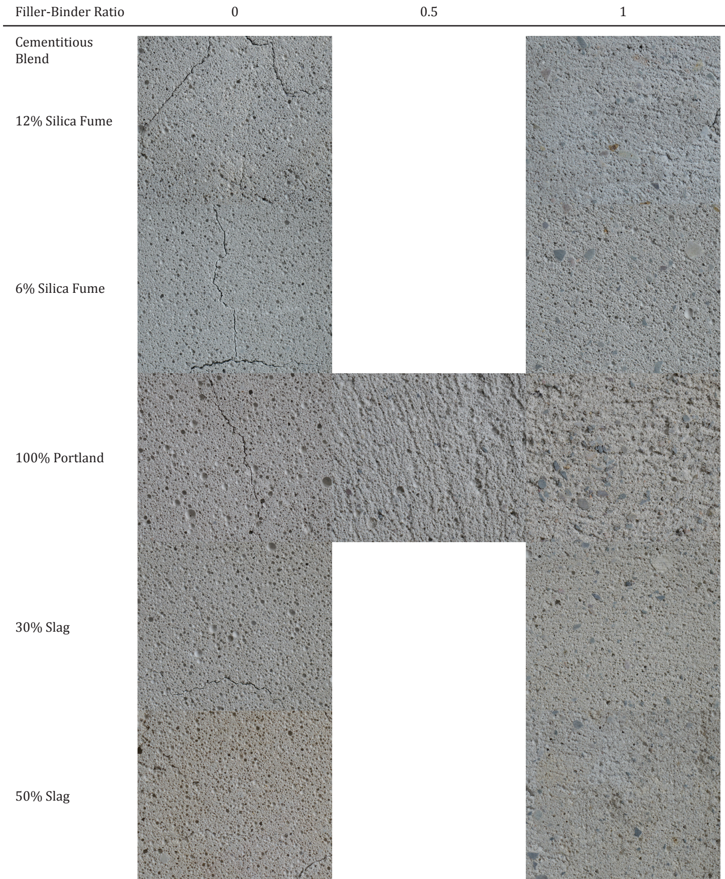
Figure 6.17.1a Foam concrete specimen sections at 1x magnification.
