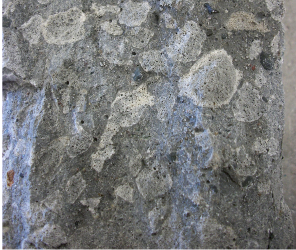
Figure E.2.1 FCA in wet-cast mix.
