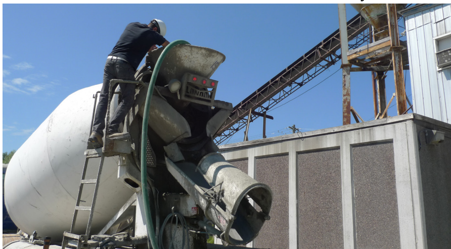
Figure S.6.1 Batching of low density foam concrete in the field. Producing good quality, neat cement foam concrete to a specification is relatively uncomplicated: the material is highly homogenous (no aggregate), and foam volumes are high, permitting a large margin of error in adding foam volume to achieve a particular density.
