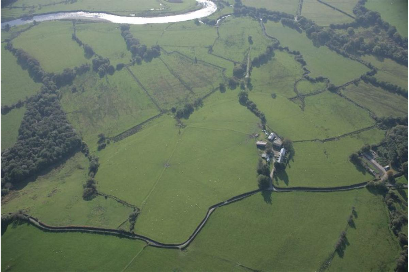
Figure 8. Pennal. An aerial view of the fort, its northwestern corner defined by the farmhouse, looking south to the confluence of the River Dyfi.
