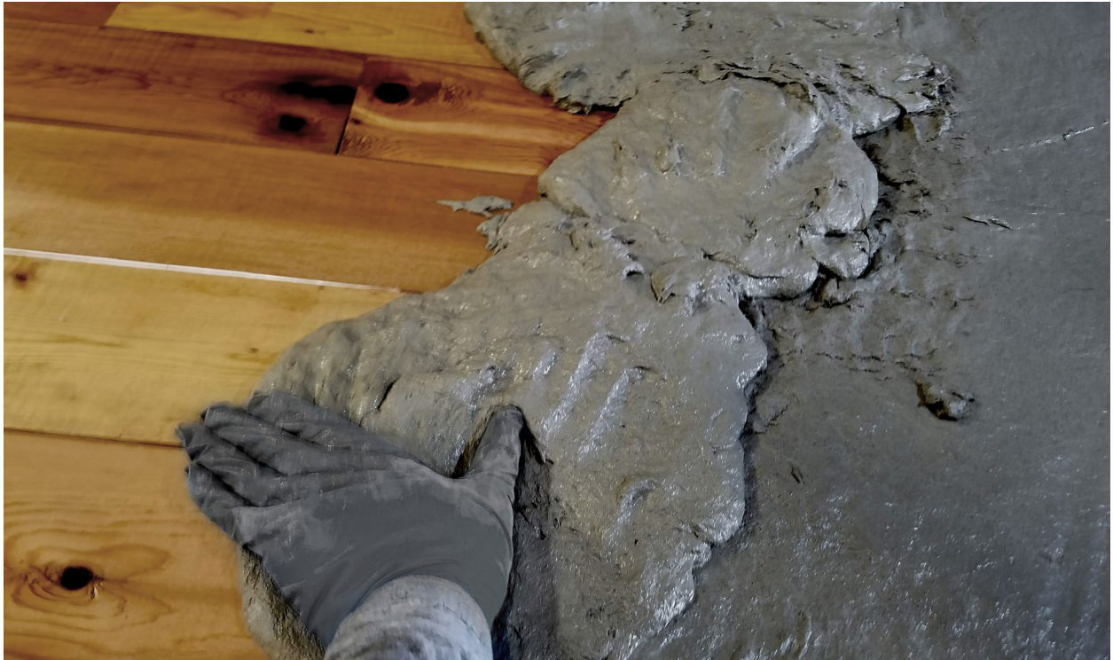
fig. 19 Initially hands flatten the viscous mix and blend the seams together
