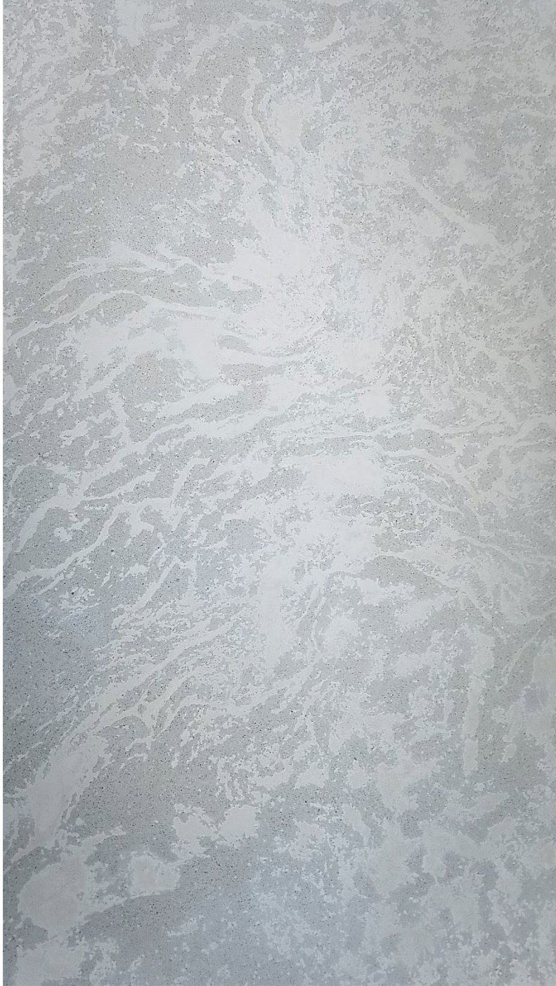
fig. 22 Irregular patterns filled with new ECC during finishing
