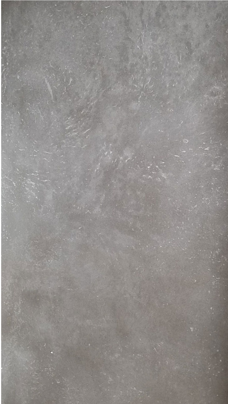
fig. 21 Irregular patterns from trowelling
