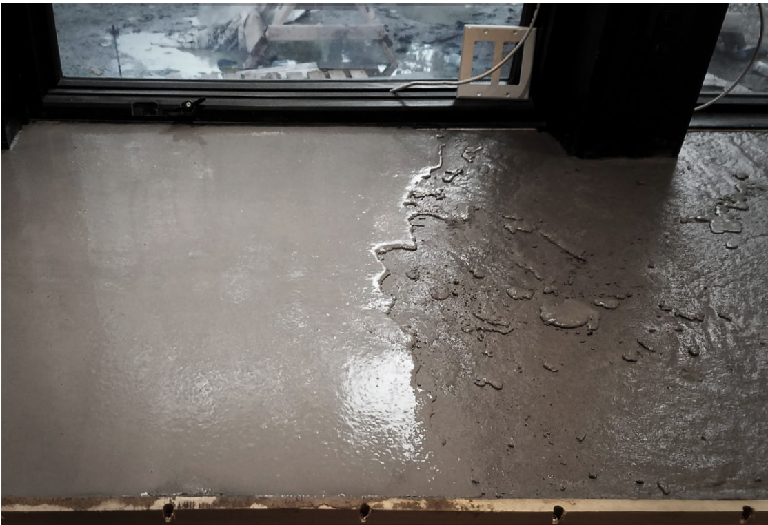
fig. 14 Fluid topping layer is applied over the already set bottom layer
