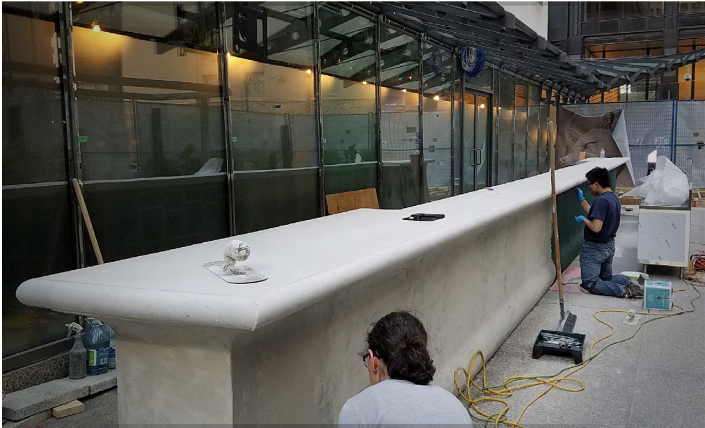
fig. 15 Casting 20-foot bar in sequence
