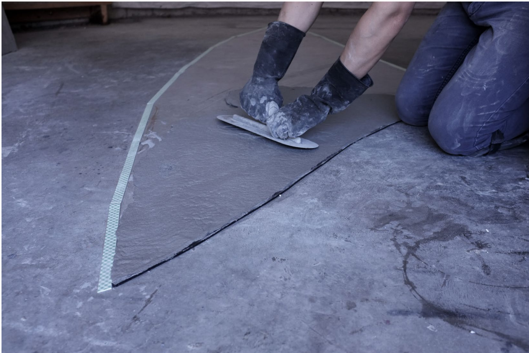
fig. 28 Trowelling ECC onto fabric to be draped
