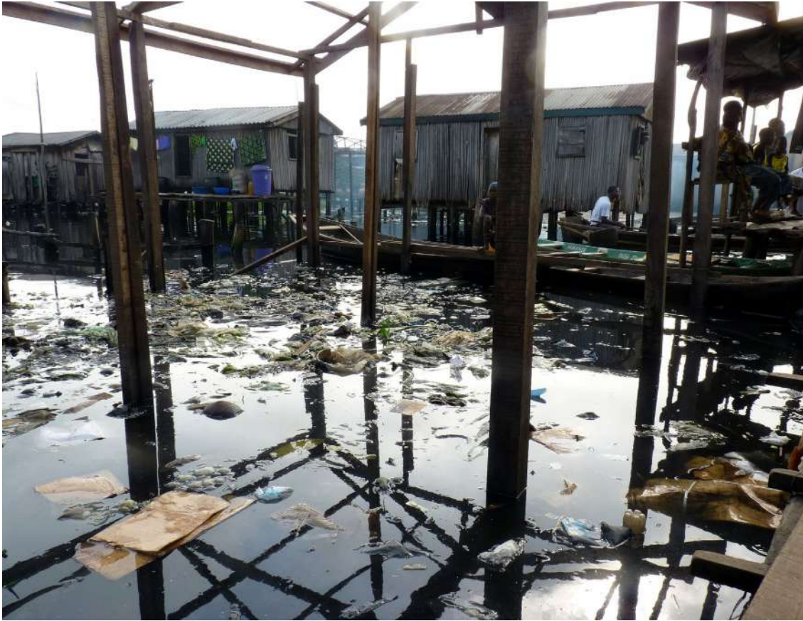
FIGURE 6.02 Typical flood conditions in Makoko
