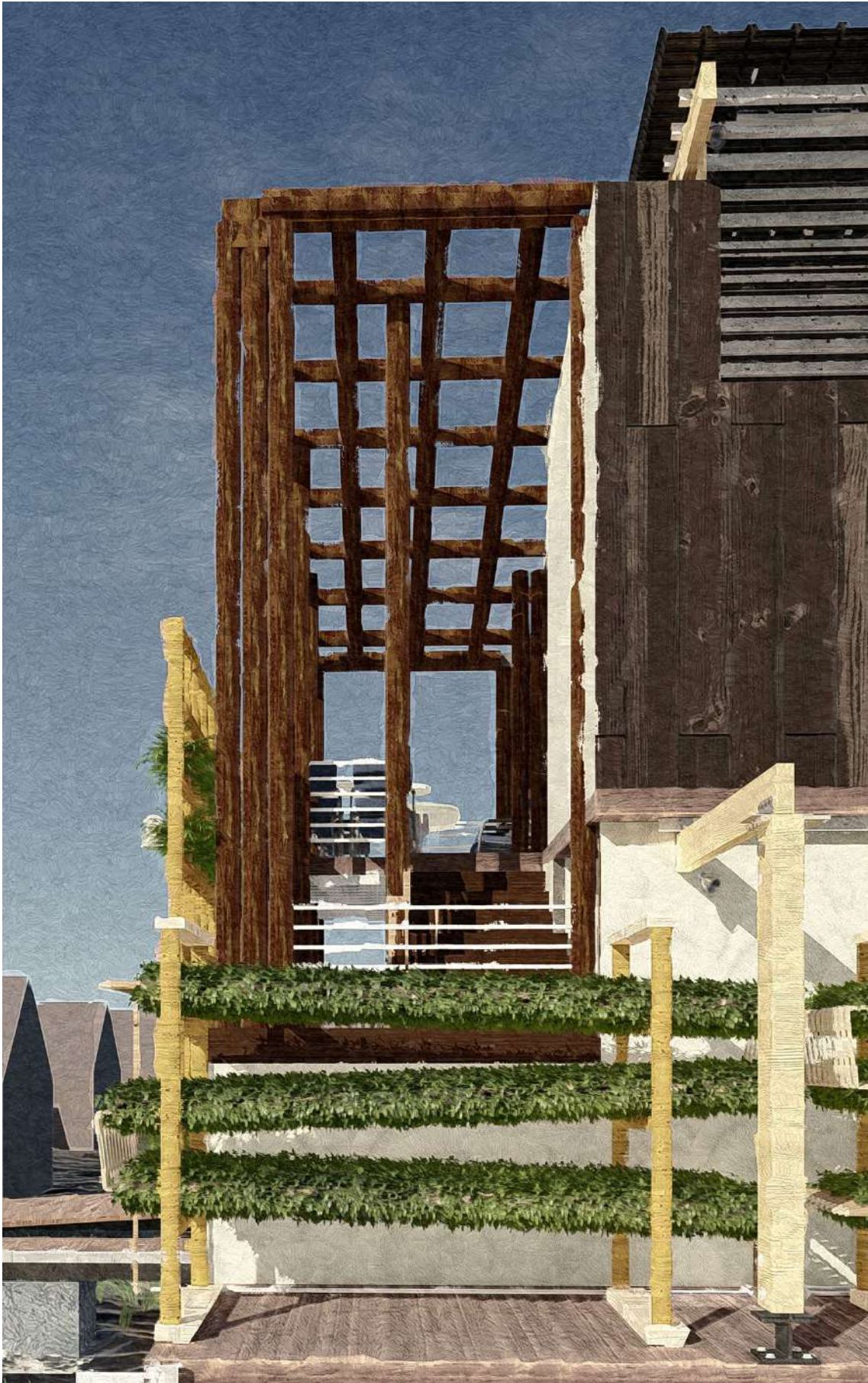
FIGURE 4.47 Bamboo structure on the East facade
