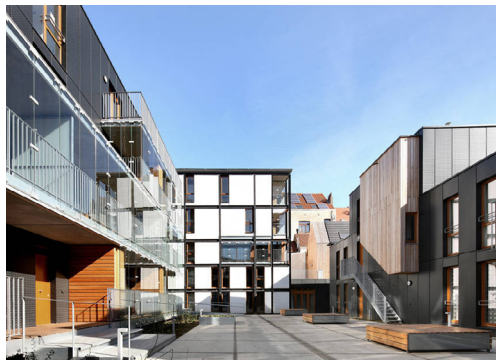
3.30 (Right) The transparency of the facades create a sense of porosity while the more solid elements define an edge which holds the courtyard in place as a central gathering space.
