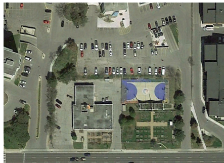
3.10 (Left) ESS is situated between the two residential towers and this provides a platform for social engagement between the towers
