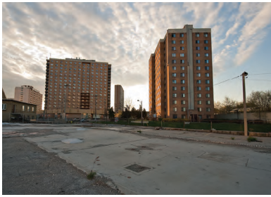
3.2 (Above) Empty parking lots surrounding the towers highlights the importance given to automobiles when they were initially built
