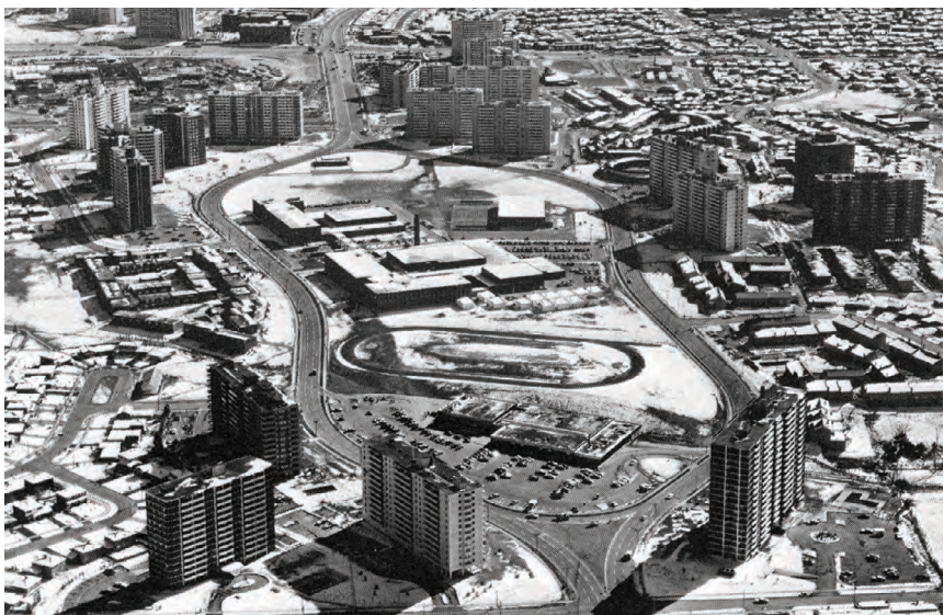
3.5 (Left) Aerial view of the urban fabric which clearly shows the 'tower in the park' design of the buildings and highlight the dominance on automobiles
