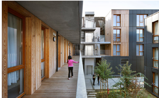
3.28 (Right) The balcony overlooking the courtyard provides a transitional space between the indoor and outdoor which can be used as social gathering spaces
