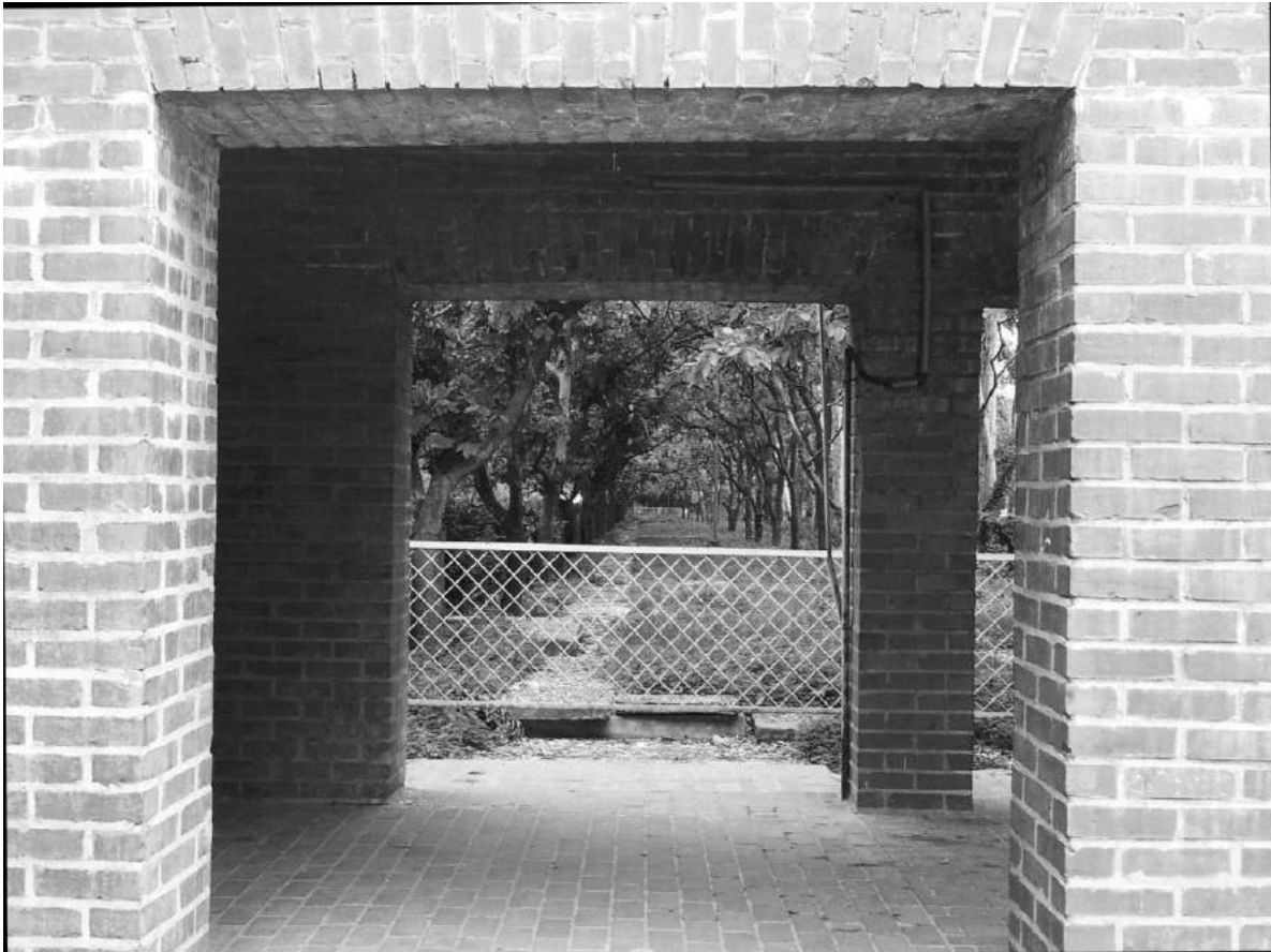
Figure 2.11 Passage to Entrance at Level 1, National Assembly Building, Dhaka
