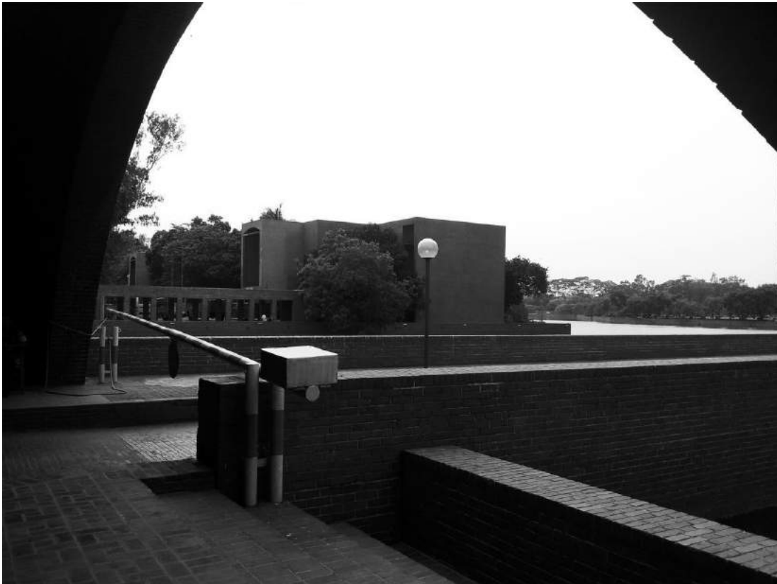
Figure 2.26 Passage to Entrance at Level 1, National Assembly Building, Dhaka
