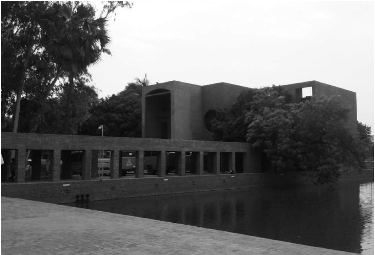
Figure 2.27 Passage to Entrance at Level 1, National Assembly Building, Dhaka
