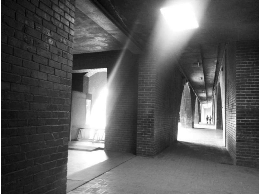
Figure 2.19 Passage to Entrance at Level 1, National Assembly Building, Dhaka
