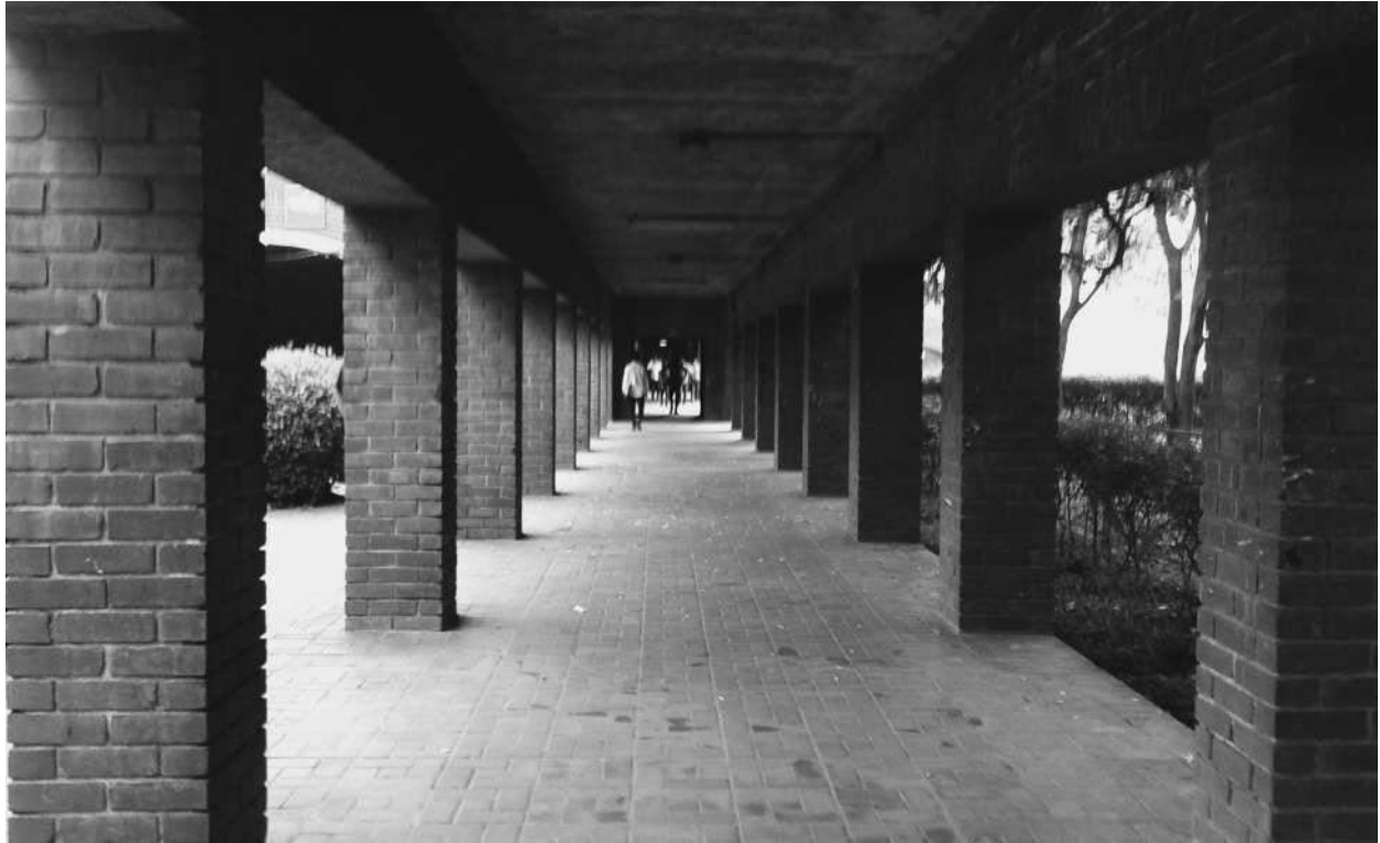
Figure 2.10 Passage to Entrance at Level 1, National Assembly Building, Dhaka
