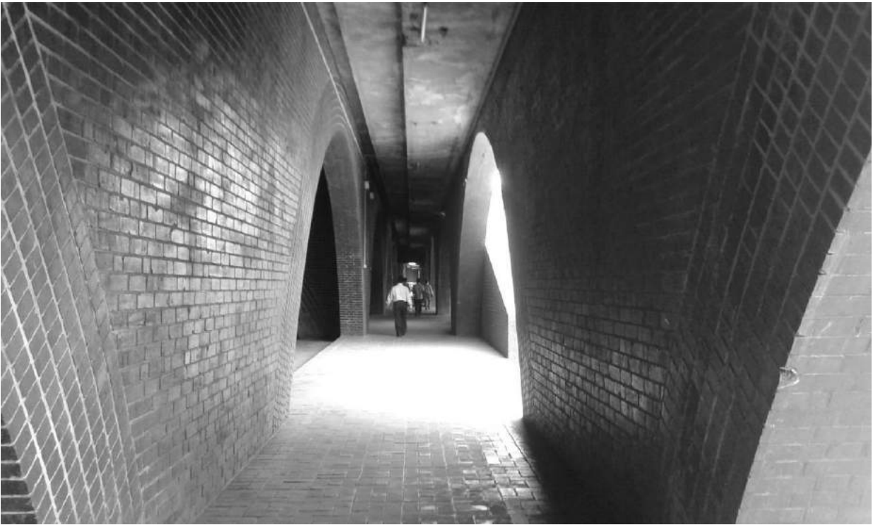
Figure 2.14 Passage to Entrance at Level 1, National Assembly Building, Dhaka
