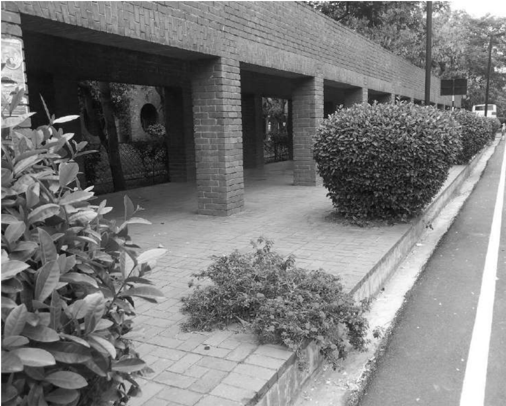
Figure 2.09 Passage to Entrance at Level 1, National Assembly Building, Dhaka
