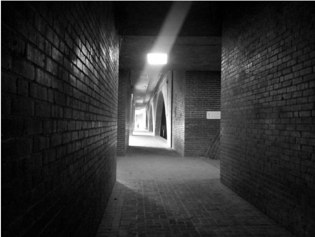
Figure 2.18 Passage to Entrance at Level 1, National Assembly Building, Dhaka
