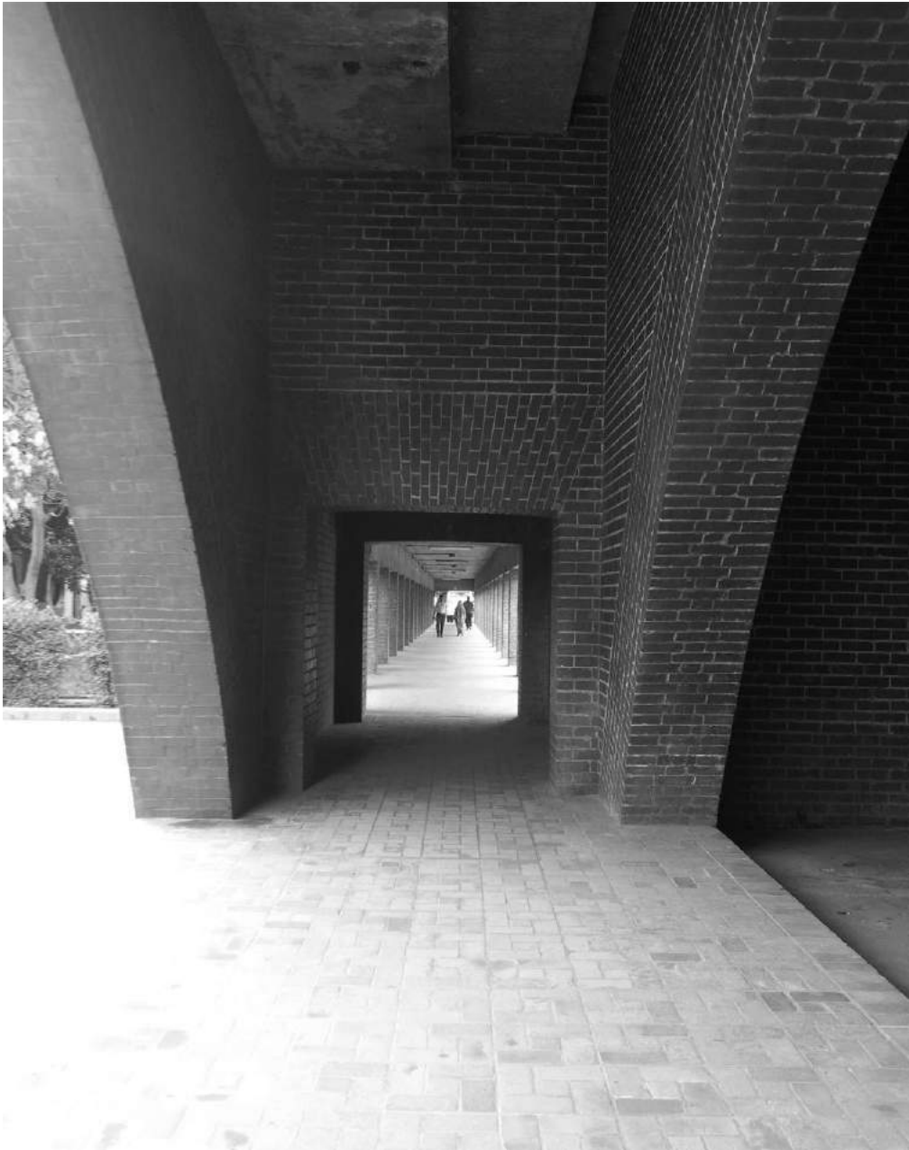
Figure 2.13 Passage to Entrance at Level 1, National Assembly Building, Dhaka
