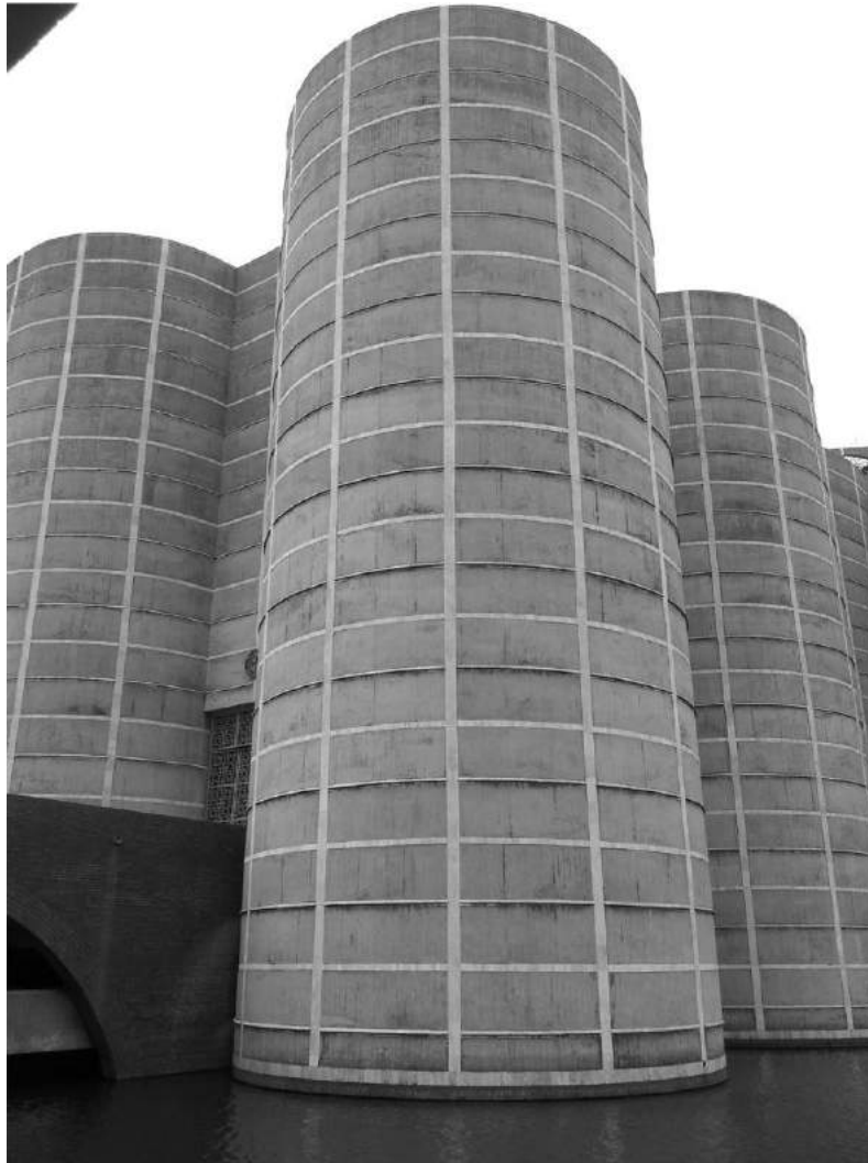
Figure 2.23 Passage to Entrance at Level 1, National Assembly Building, Dhaka
