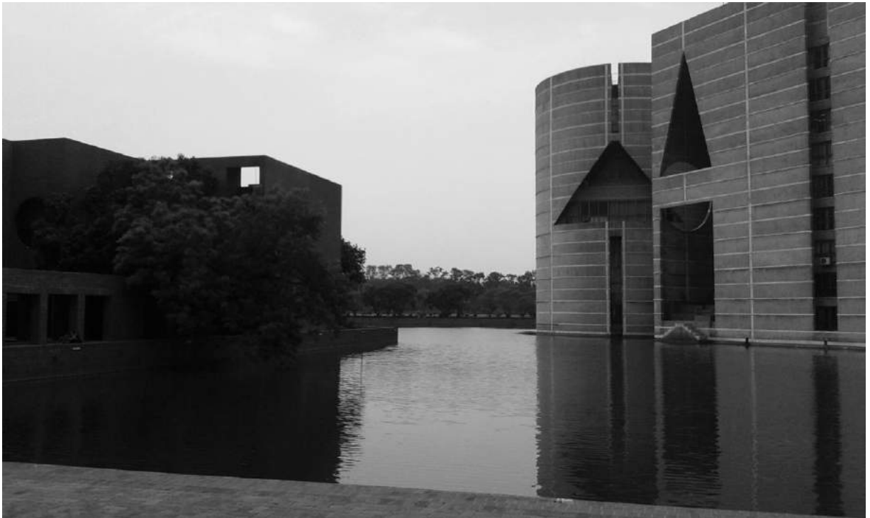
Figure 2.25 Passage to Entrance at Level 1, National Assembly Building, Dhaka
