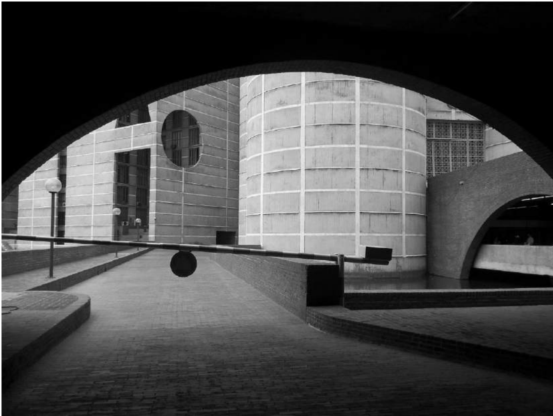
Figure 2.22 Passage to Entrance at Level 1, National Assembly Building, Dhaka
