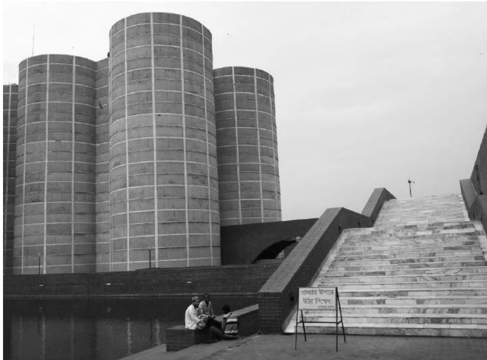
Figure 2.24 Passage to Entrance at Level 1, National Assembly Building, Dhaka
