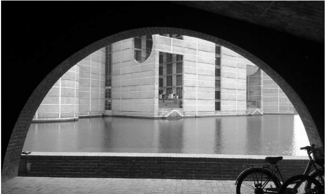
Figure 2.20 Passage to Entrance at Level 1, National Assembly Building, Dhaka
