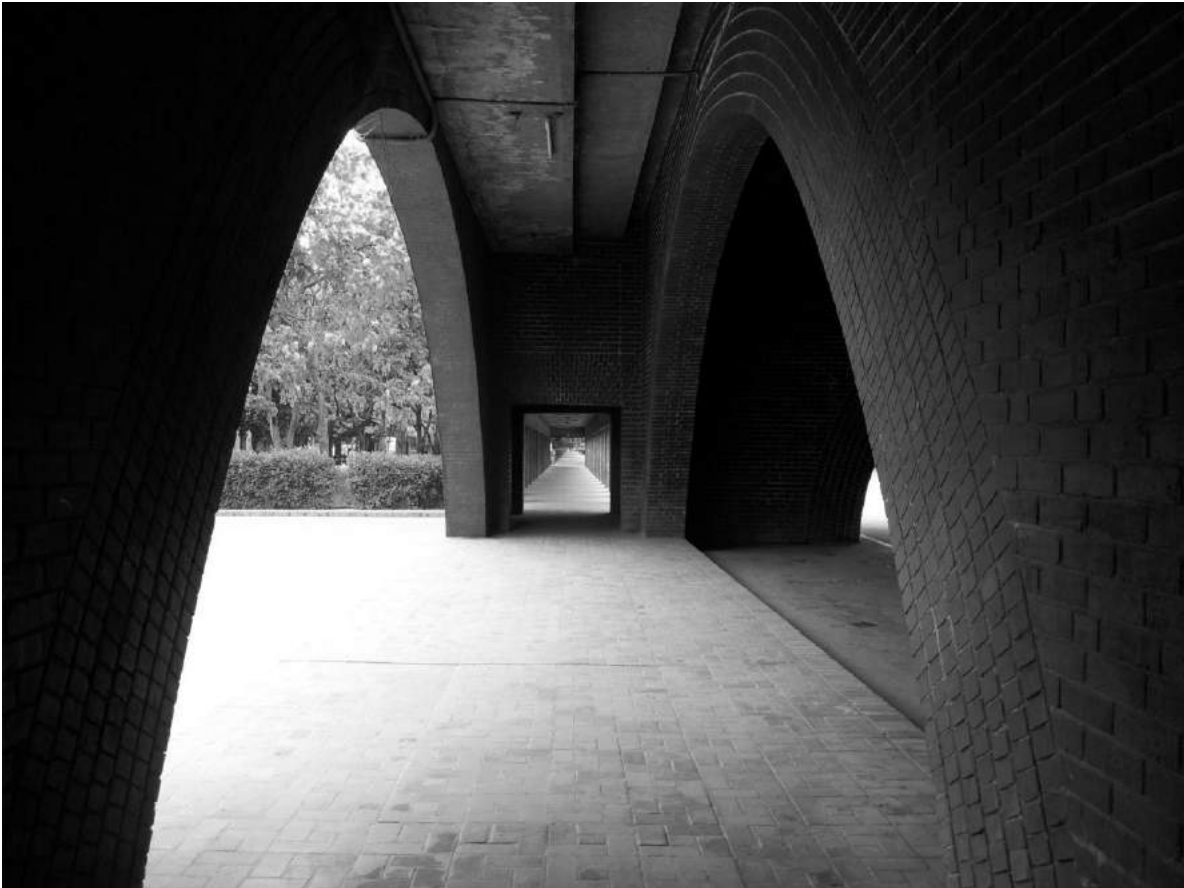
Figure 2.12 Passage to Entrance at Level 1, National Assembly Building, Dhaka
