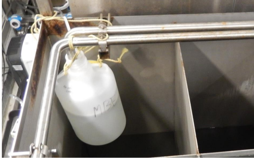
Figure 3-5. Filter effluent collection in Toronto R.C. Harris Water Treatment pilot plant clearwell during Seeding Protocol Validation Experiments.
