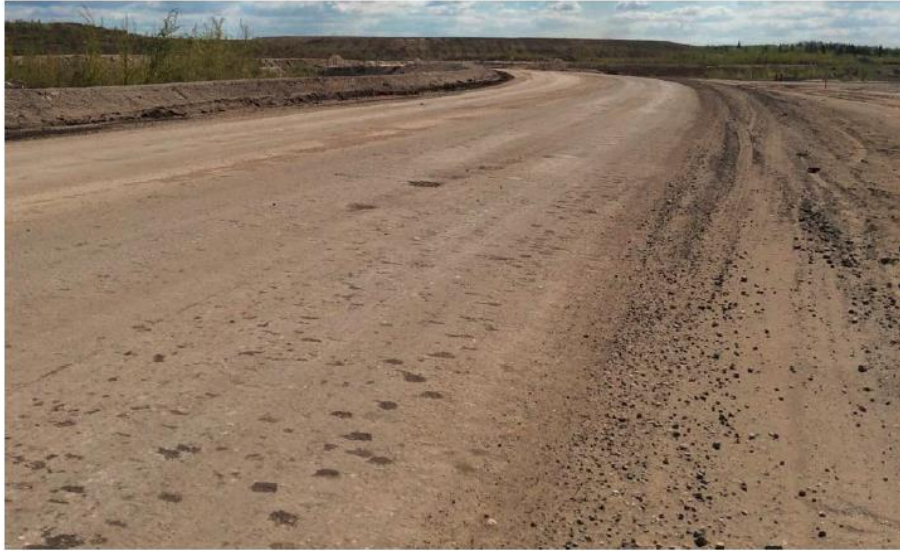
Figure 12 OPP2 Access Road (south-facing view)
