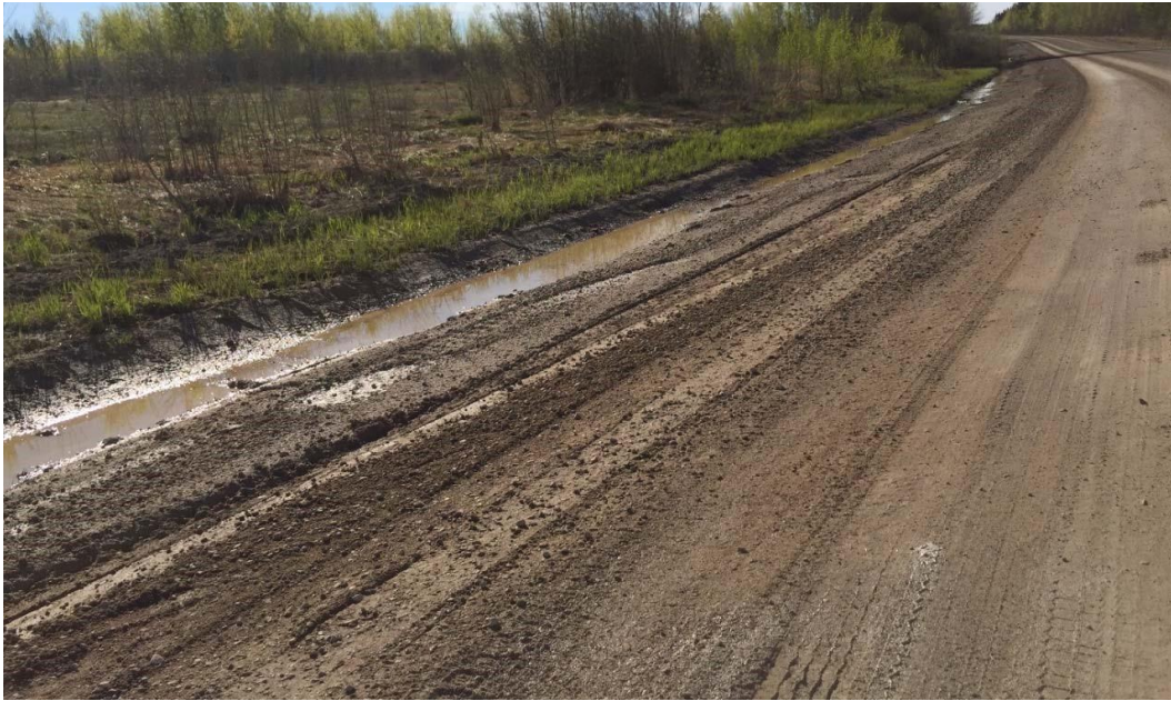
Figure 26 Water Pond on Canterra Road
