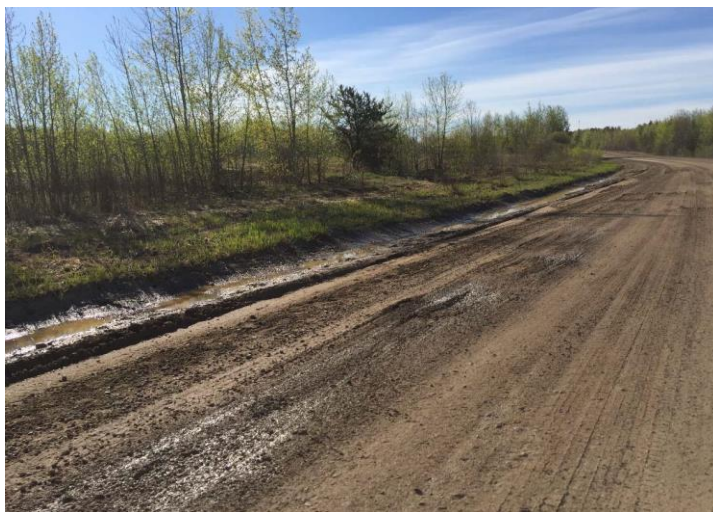
Figure 4 Soft Spots on Outside of Wheel Path
