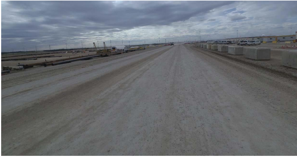
Figure 11 K2 Laydown Road (west-facing view)
