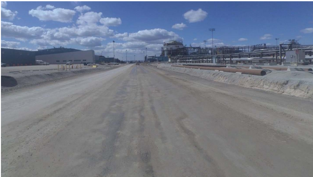
Figure 10 Control Room Road (west-facing view)
