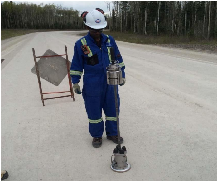
Figure 15 Light Weight Deflectometer (LWD) Test on MPAR Road
