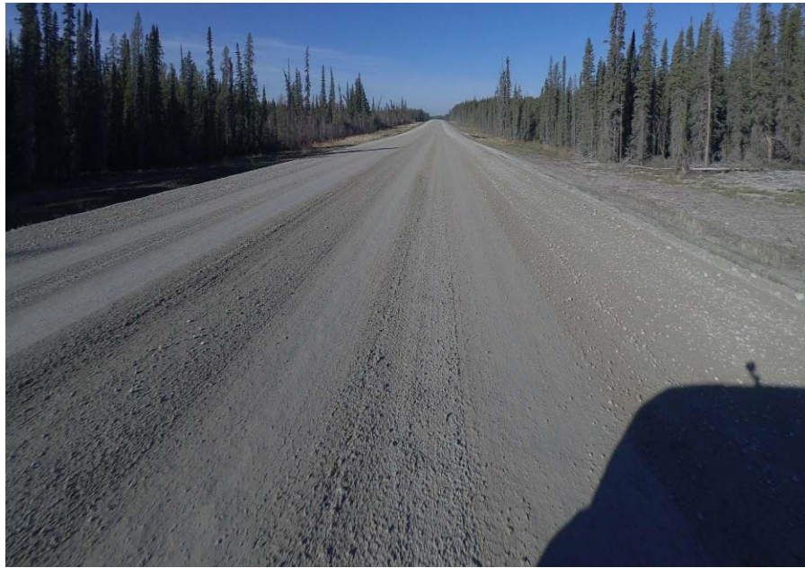
Figure 13 Main Plant Access Road (MPRP) Road
