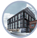
1554 Dundas St. W. Alto Rental Suites Condo Under Construction
