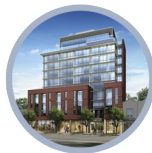
2055 Danforth Ave. Carmelina Condos Condo Under Construction
