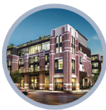
2000 Queen St. E. Bellefair Kew Beach Condo Under Construction
