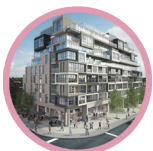
829 St. Clair Ave. W. Nest Condos Condo Pre-Construction
