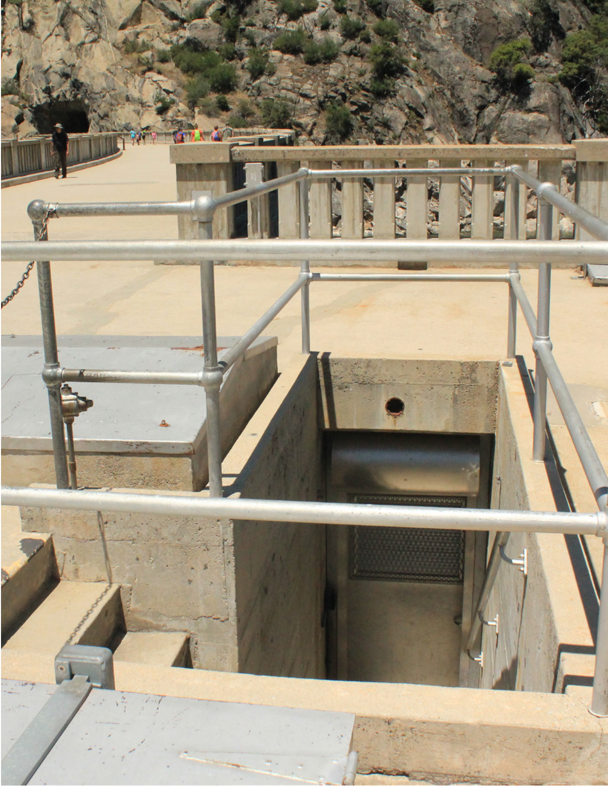
Figure 2.90 Access into the dam's innards.
