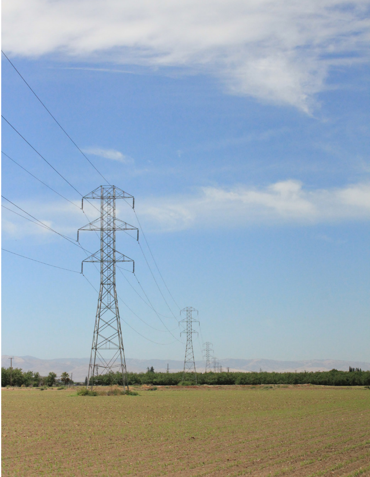
Figure 2.53 Power lines carrying Hetch Hetchy electricity straddling a hidden stretch of the San Joaquin pipeline, headed to San Francisco, with the Coastal Range in the distance.
