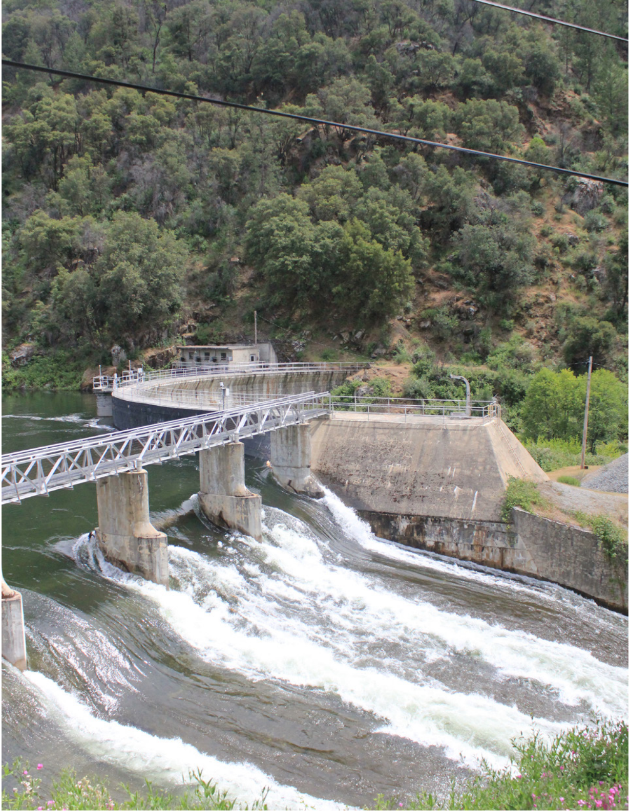
Figure 2.75 Early Intake Dam, Tuolumne River.
