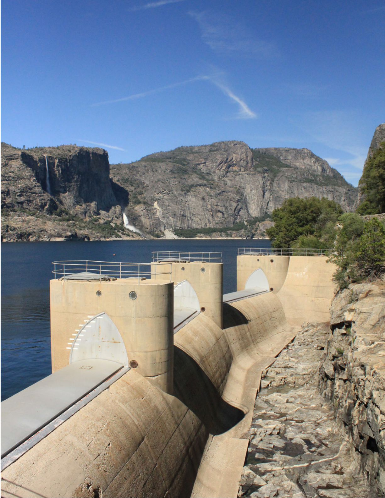
Figure 2.82 Rear of dam spillway and reservoir.
