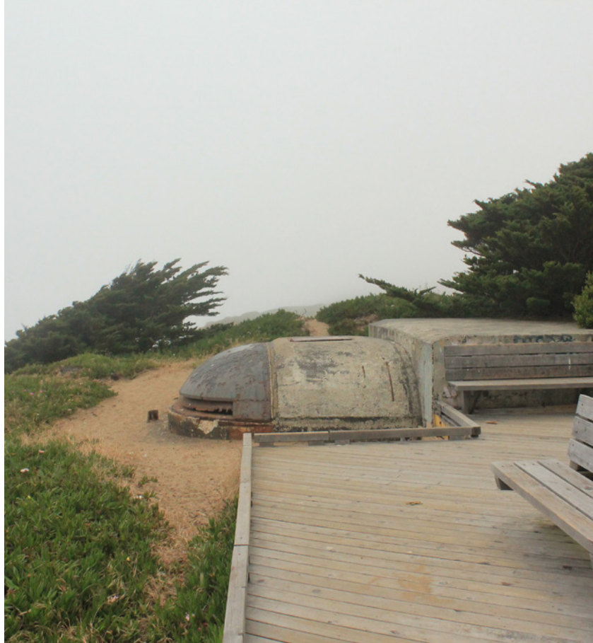
Figure 4.3 Boardwalks and bunkers at Fort Funston.
