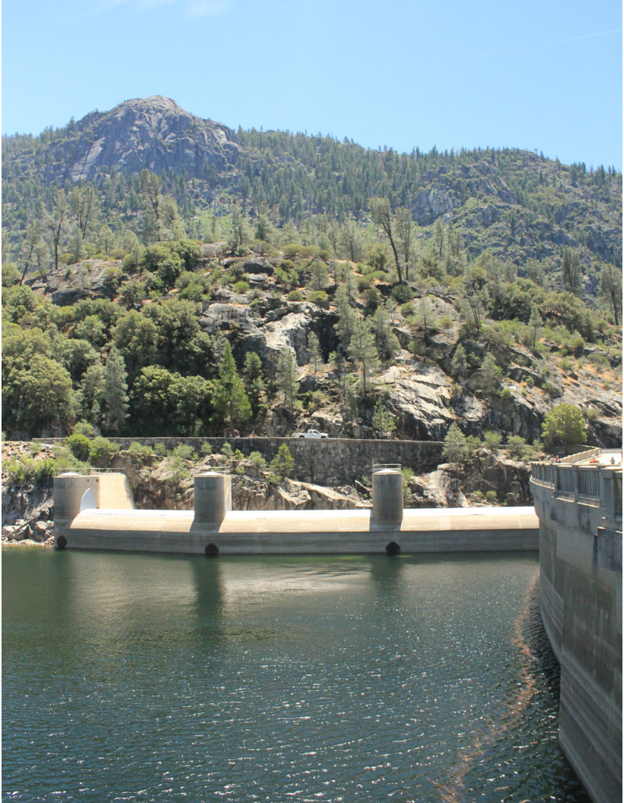
Figure 2.97 The opposite side of the spillway.
