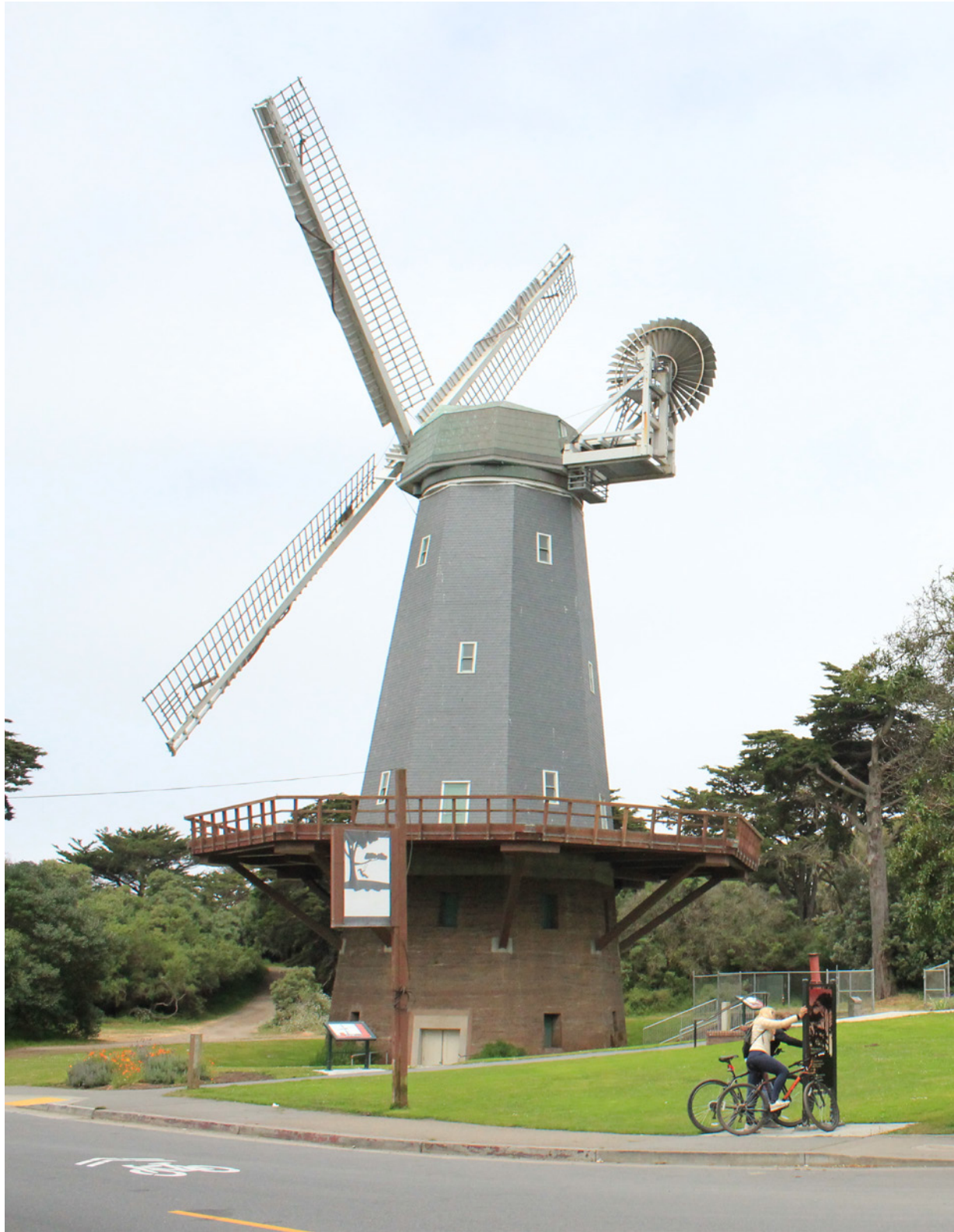
Figure 2.38 The Murphy Windmill was once used to irrigate the park with groundwater.
