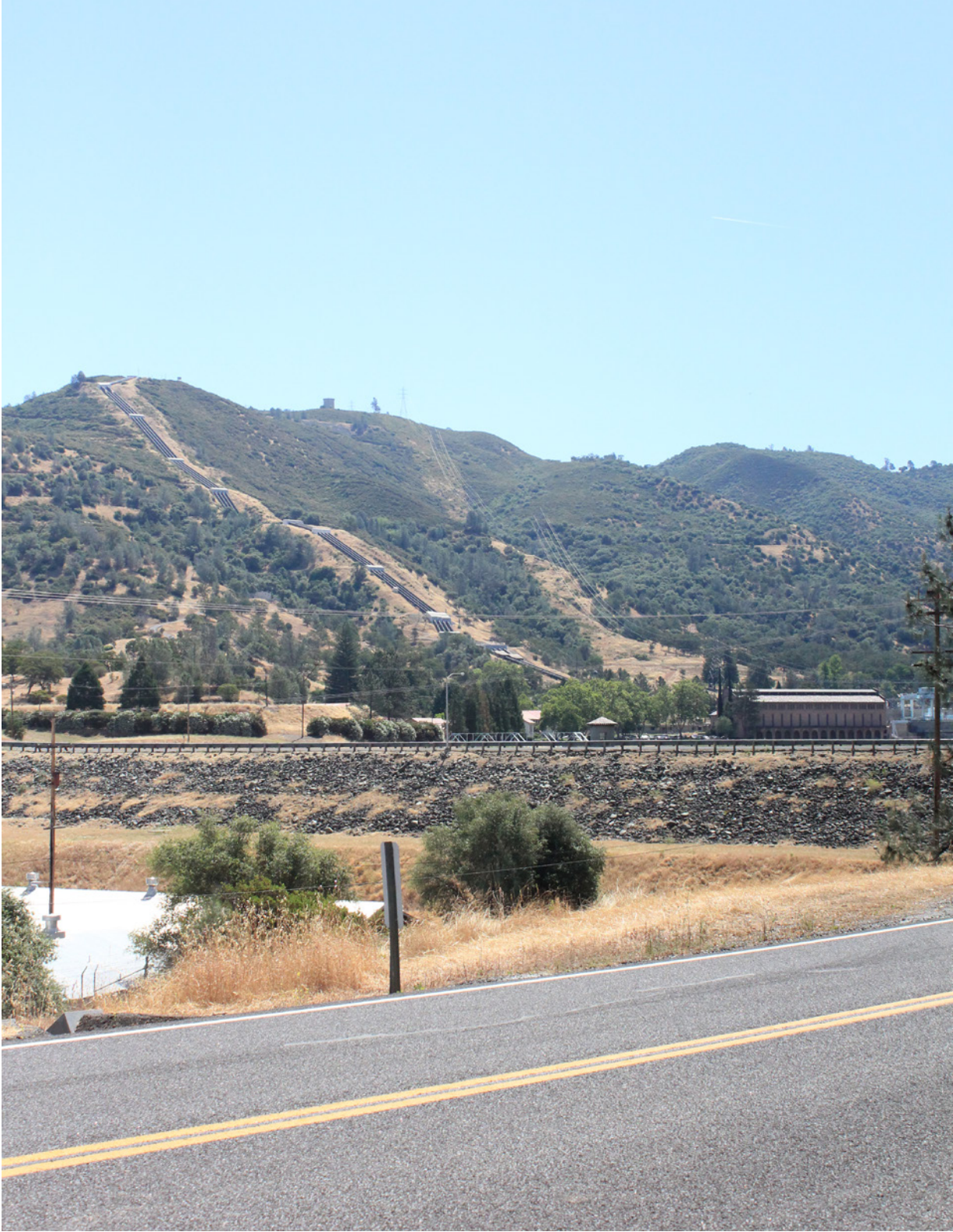
Figure 2.68 Moccasin, with pipeline cascade, and old and new power plants.
