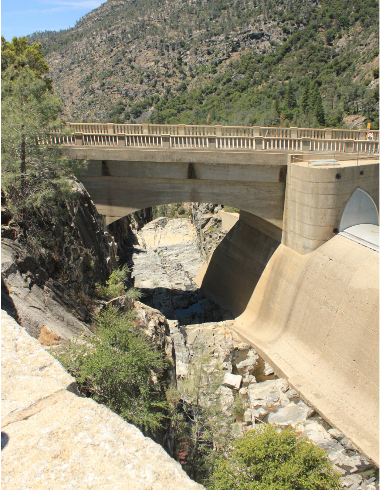
Figure 2.83 Dam spillway, looking downstream.
