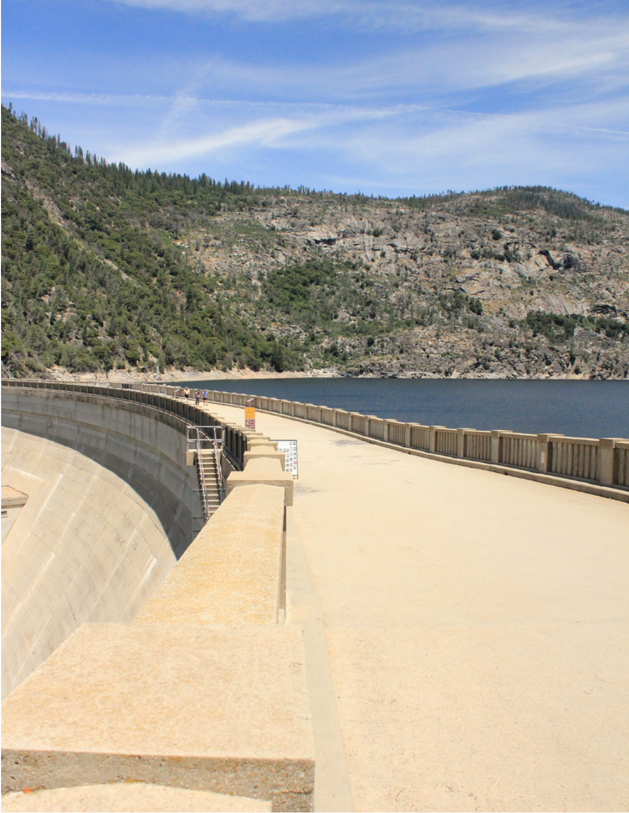
Figure 2.86 Walkway atop dam.
