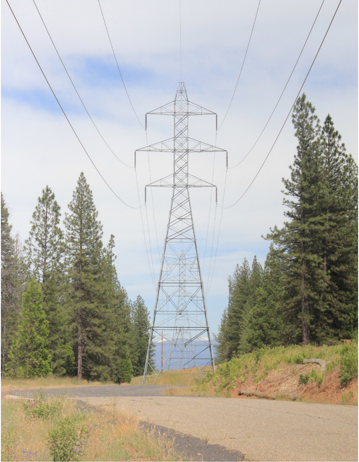
Figure 2.71 Hetch Hetchy power lines crossing over Statre Route 120.
