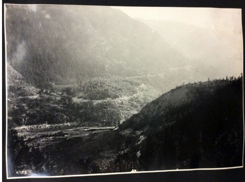
Figure 3.8 The site of O'Shaughnessy Dam at the west end of Hetch Hetchy Valley, prior to construction.
