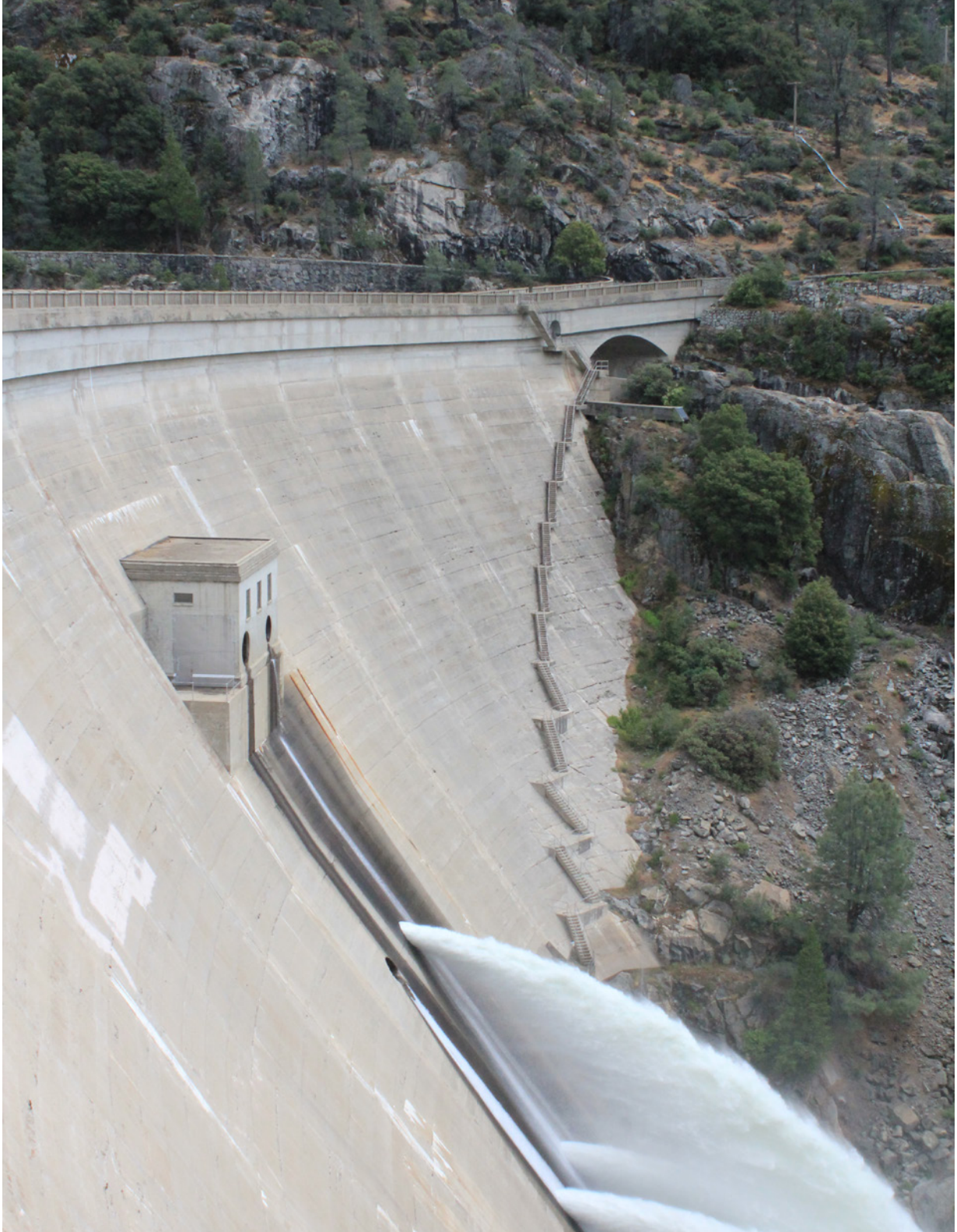
Figure 2.93 The front of the dam.
