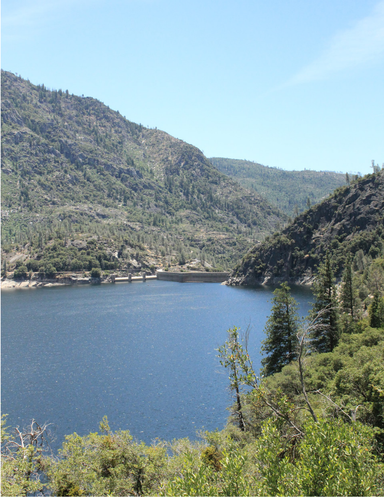
Figure 2.98 The dam and reservoir from above.
