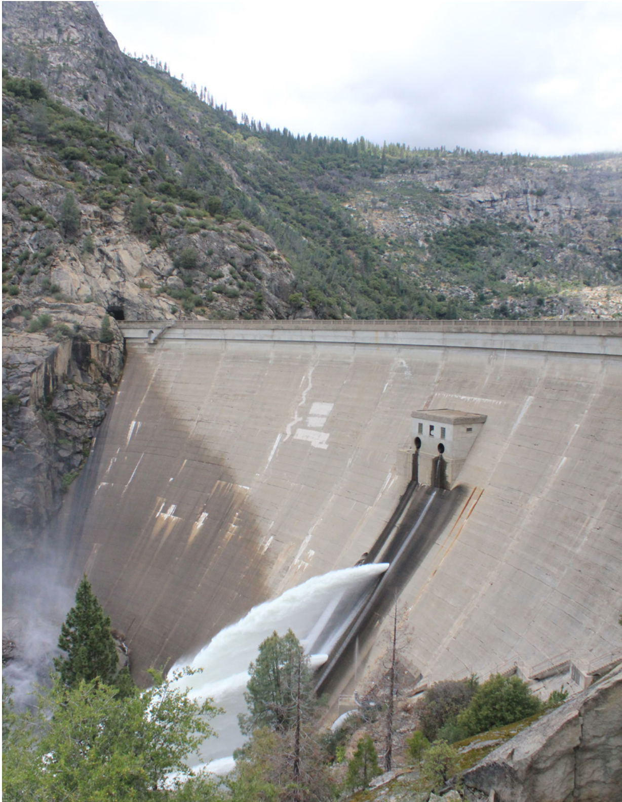
Figure 2.80 Front of O'Shaughnessy Dam during water release.
