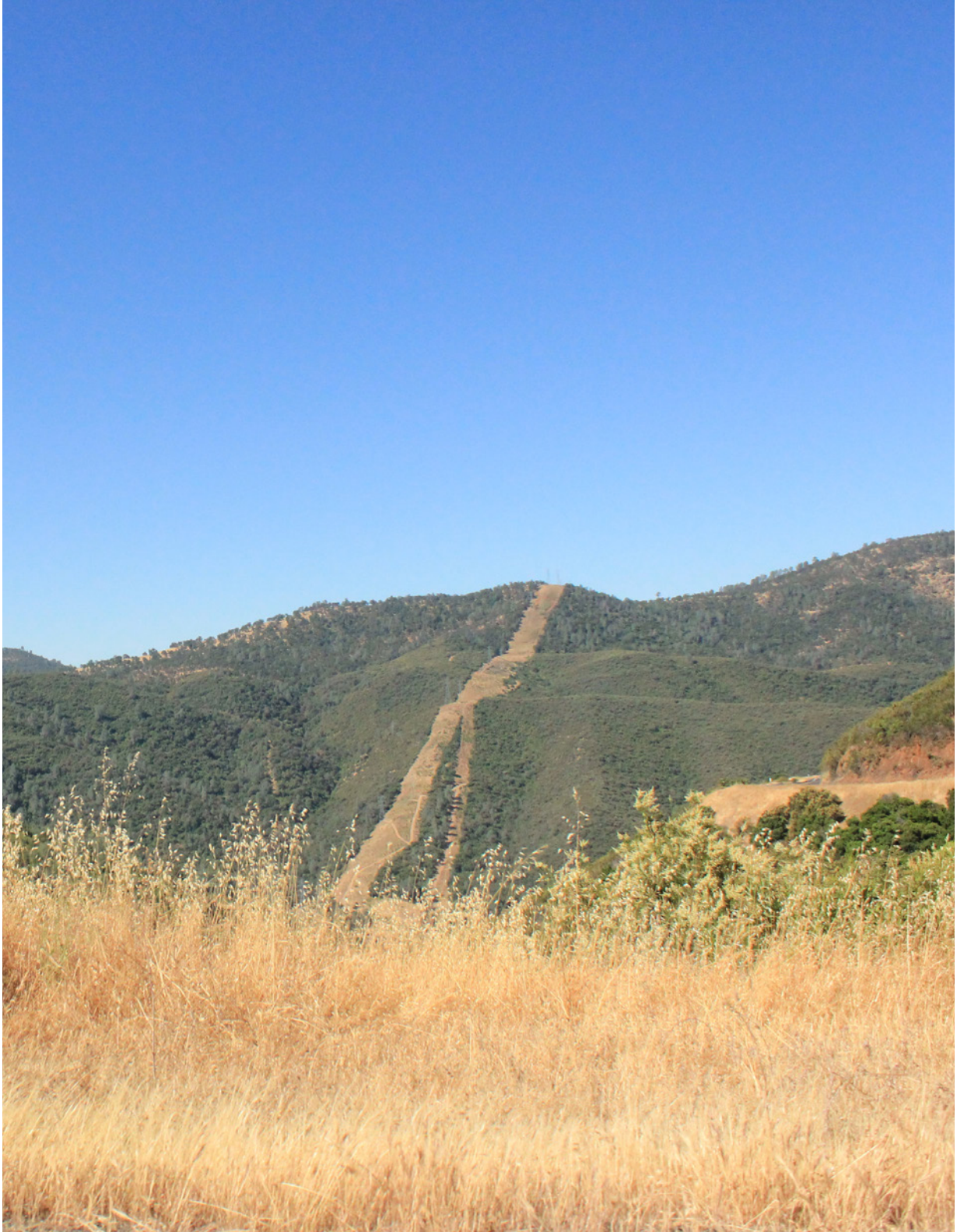
Figure 2.69 Power lines ascend out of Moccasin.
