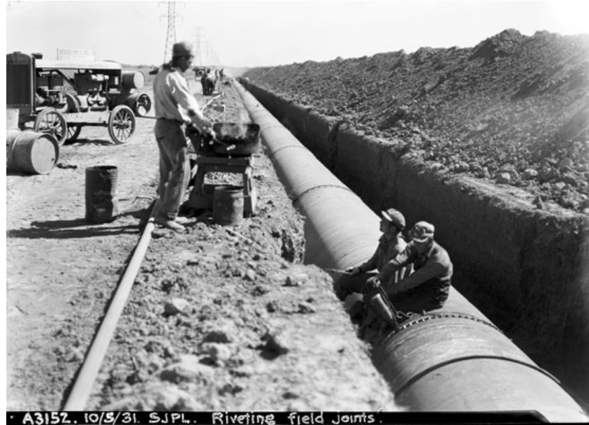
Figure 3.6 Building the San Joaquin Pipeline in 1931; in the background, pylons already carrying Hetch Hetchy power are visible.
