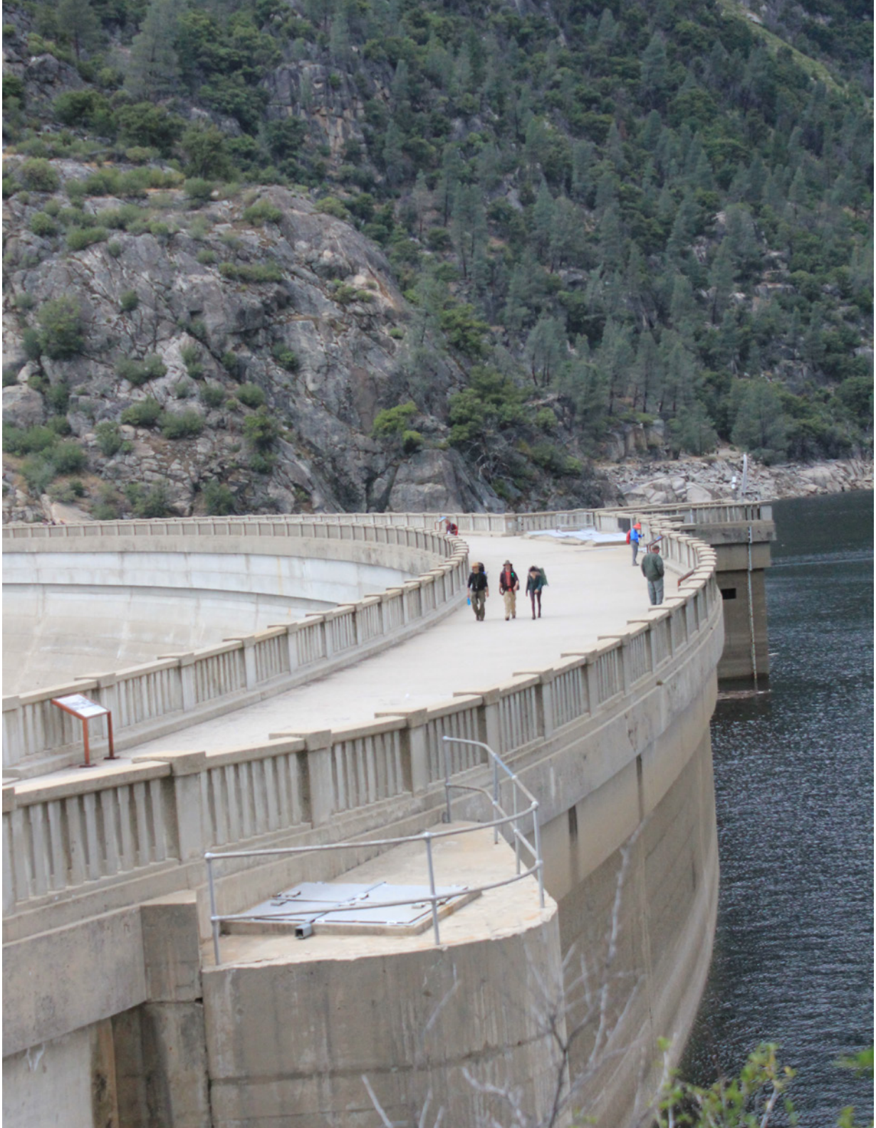
Figure 2.87 Top of dam.
