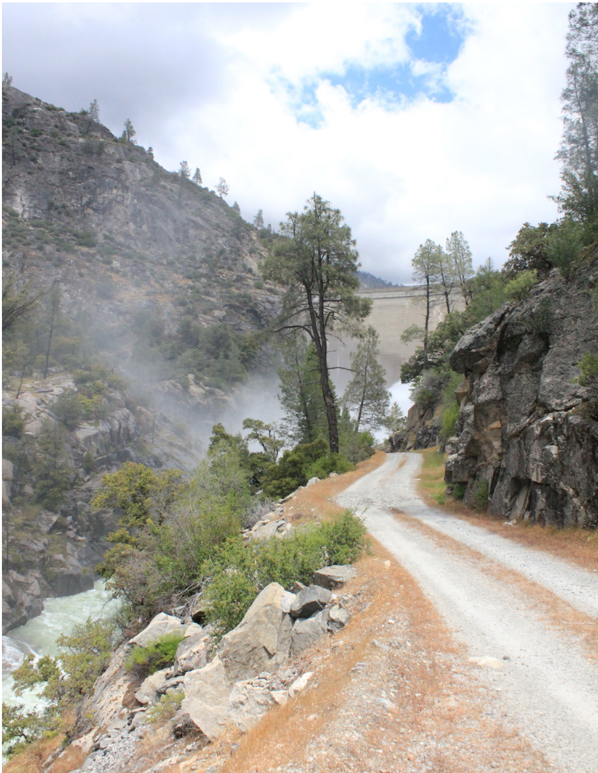
Figure 2.94 Approaching the dam from below, with the Tuolumne beside.
