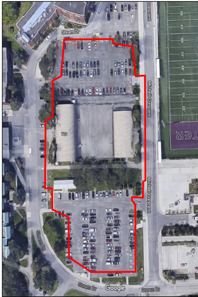
Figure 4.1. Project Site before Construction
