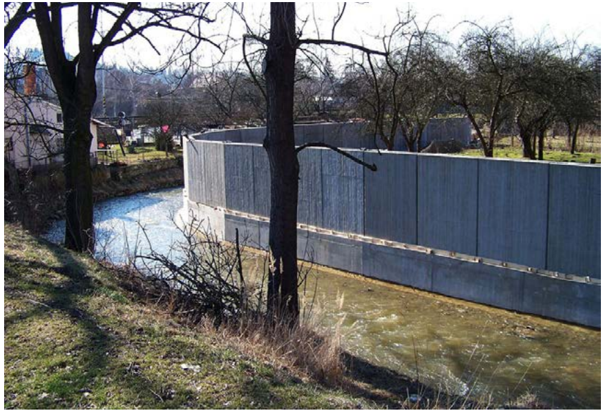
Fig.35 Flood Wall at Zruc nad Sazavou, Czech Republic
