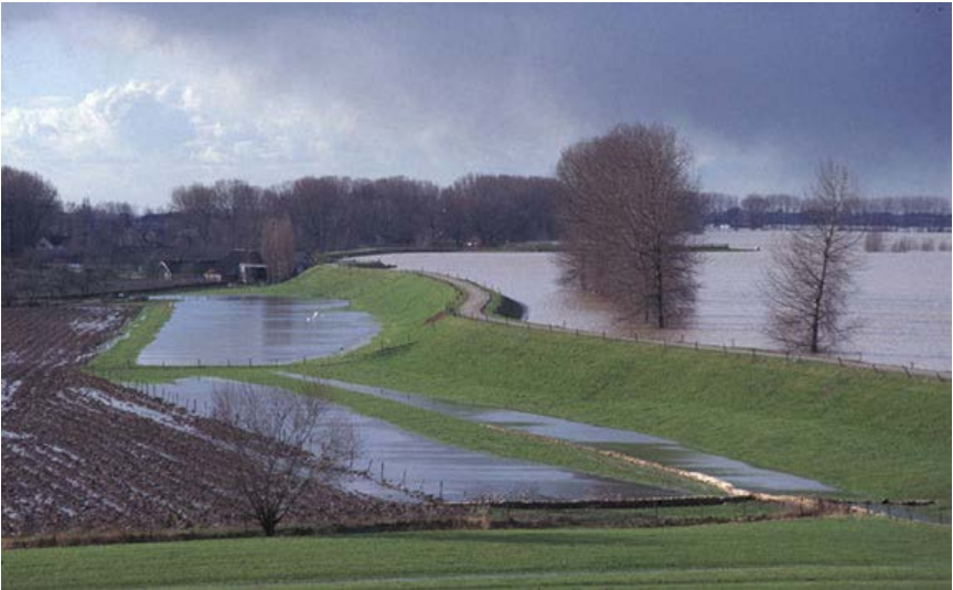
Fig.37 Dike at River Waal, the Netherlands
