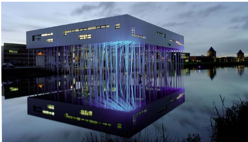
Fig.48 Aluminium Centrum , Abbink X De Haas Architectures Houten, the Netherlands
