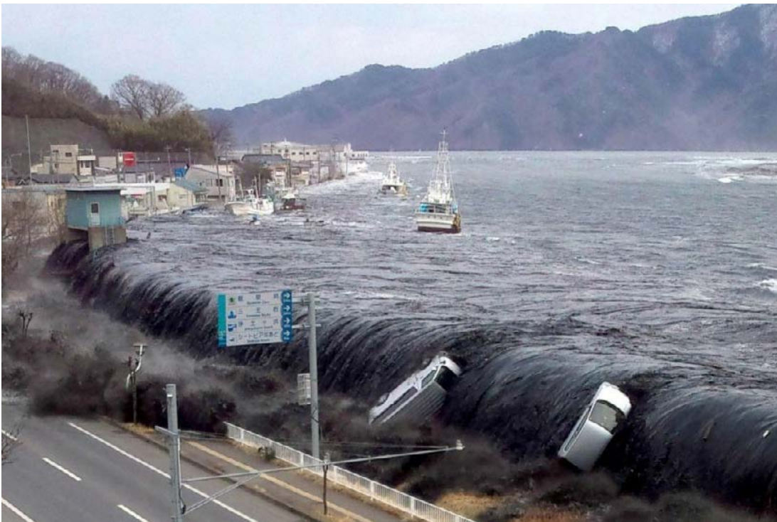
Fig.6 Breach of Flood Defence during the Japan 2011 Tohoku Tsunami
