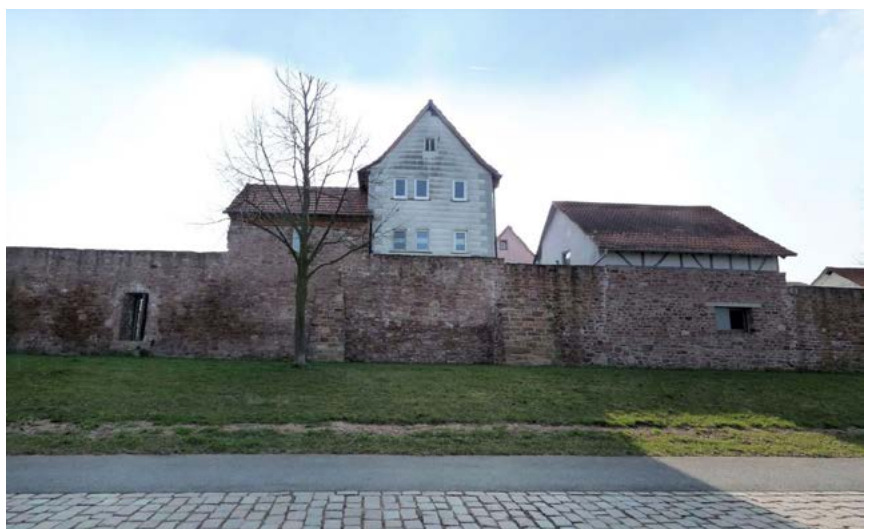
Fig.36 Integrated Flood Wall Worth am Main Germany
