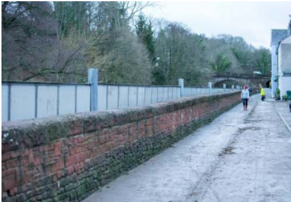
Fig.11 Flood Barrier at Cockermouth England, before and during flood event
