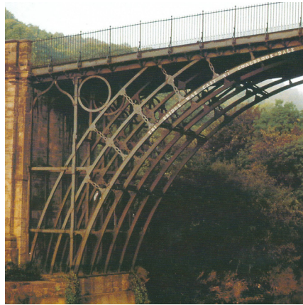
Fig. 23 The Iron-Bridge at Coalbrookdale Abraham Darby III, Built in 1777–1779
