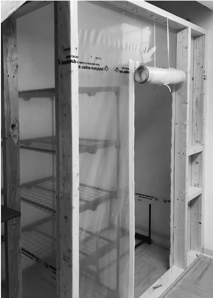
Fig.55 Completed Grow Chamber
