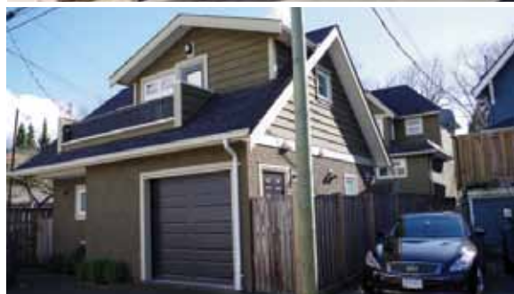
Figure 2.7.18: Existing Vancouver laneway houses
