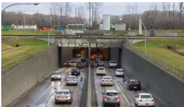
Figure 2.3.6: George Massey Tunnel. 1 Lane + 2 Alt.
