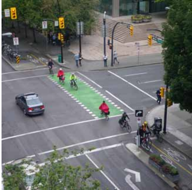
Figure 3.8.8: Fully seperated bike routes with well marked crossings and seperate bike traffic signals have made cycling a safe and viable option to an increasing number of residents.
