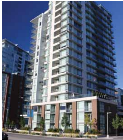
Figure 2.6.27: Condo tower & podium
