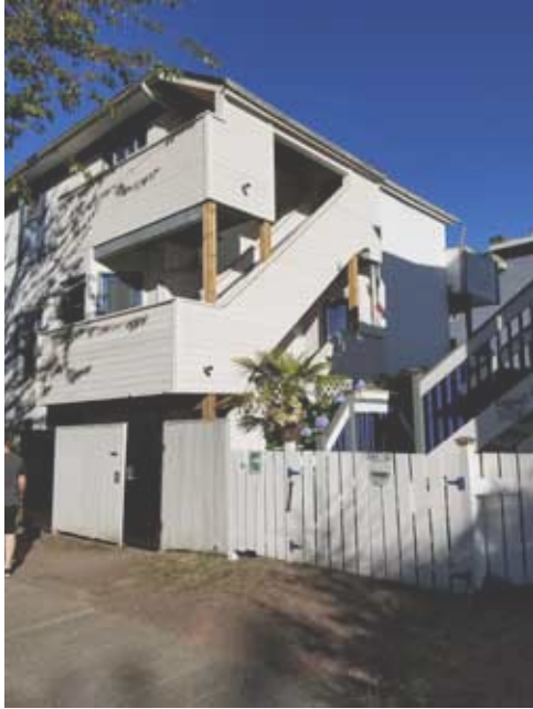
Figure 2.8.9: Exterior Stairs for upper unit entry.
