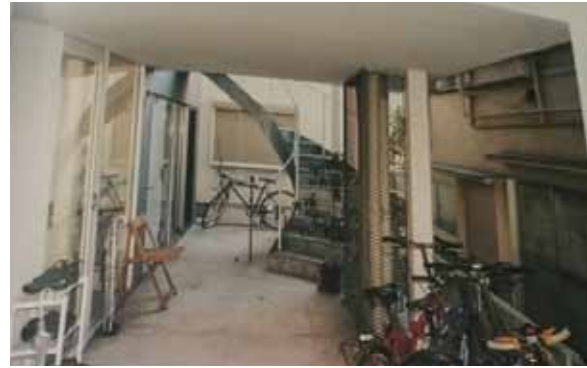
Figure 3.3.6: Yokohama Apartment. Access path.
