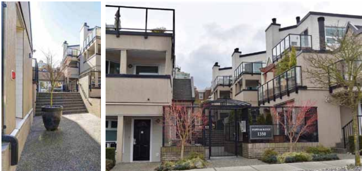
Figure 2.6.22: Pepper Ridge, Fairview, Vancouver. A common multiplex type with central exterior entry.
