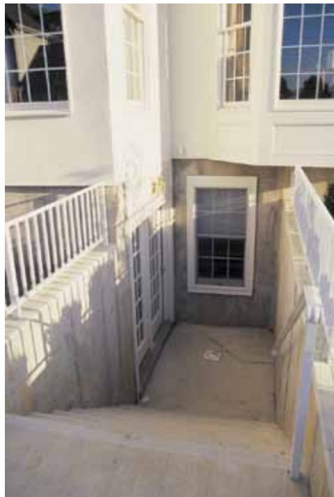
Figure 2.8.10: Concrete stairwells to access new basement units from exterior.
