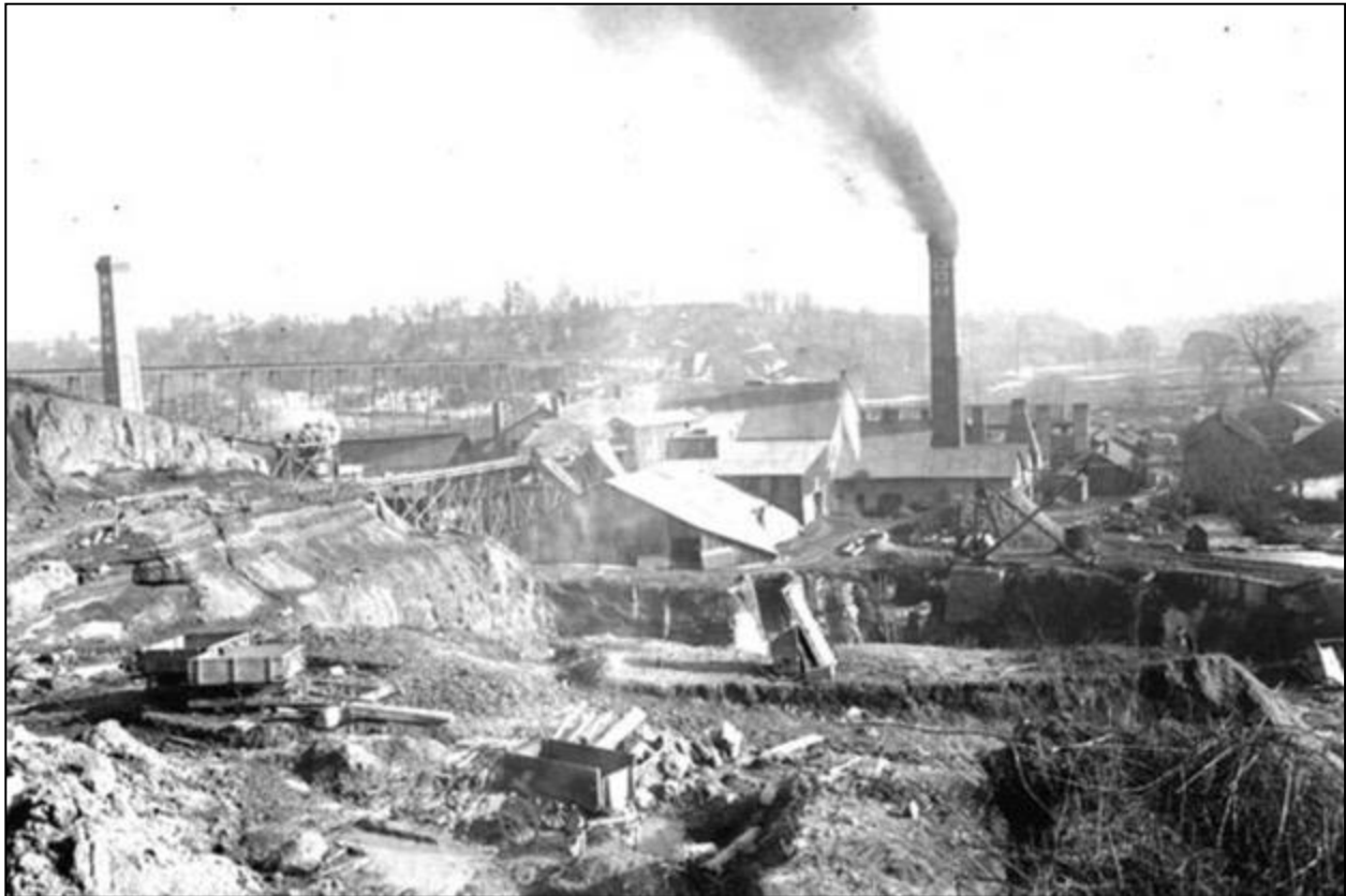
Figure 8: Don Valley Brick Works – Quarry, Pit and Buildings Pre-Adaptation
