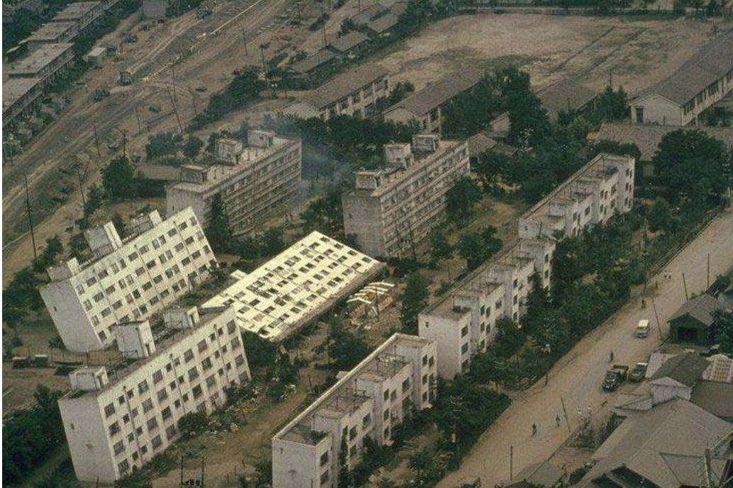
Figure 3.9: 1964 Niigata earthquake caused widespread liquefaction in Niigata, Japan, destroying many buildings (Hays 1981).
