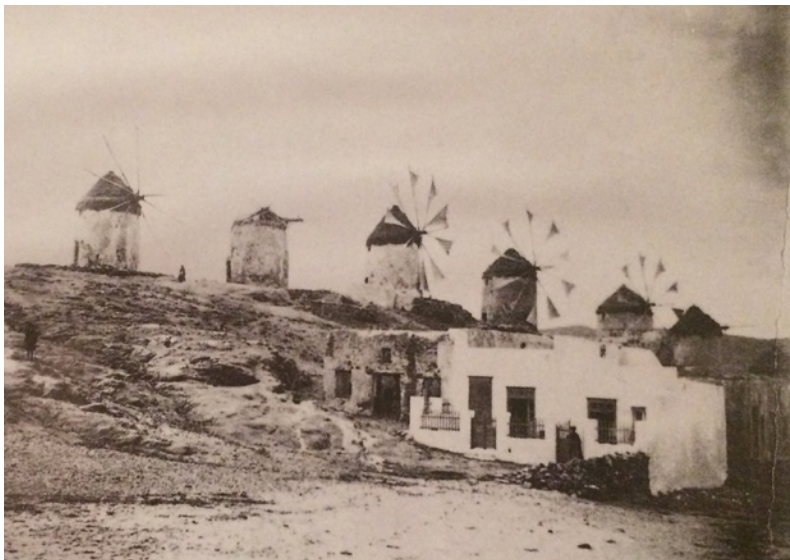
4.1 Buildings' Poor Condition before Tourism's Emergence in Mykonos (1885)
