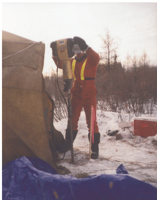
FIGURE 4.8: Steve Berg using a jackhammer to advance the Waterloo Profiler.
