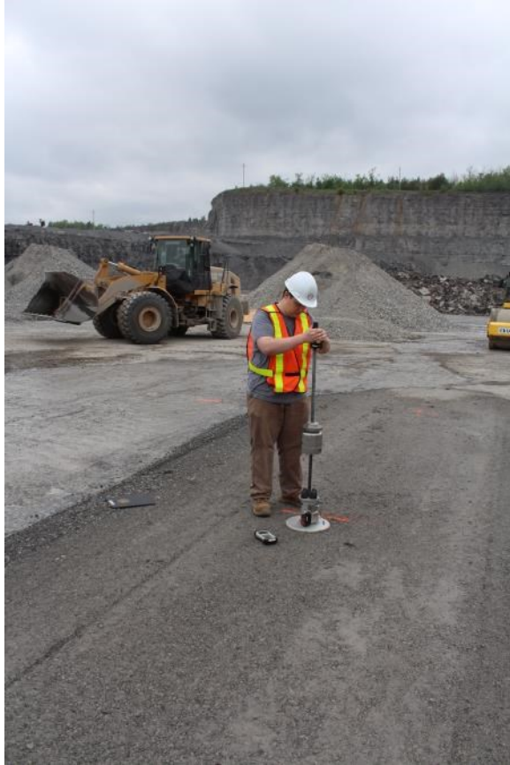
Figure 4-9. Lightweight deflectometer testing in progress at Quarry 1
