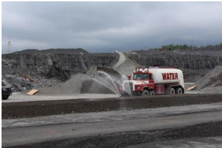
Figure 4-5. Addition of water to a test pad under compaction at Quarry 1
