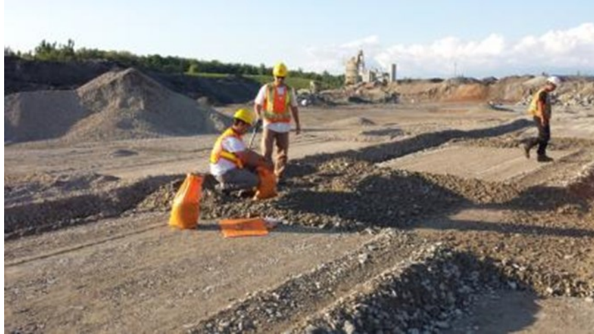
Figure 4-8. Sampling at a test pad at Quarry 2
