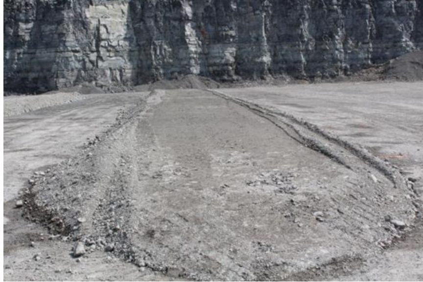
Figure 4-1. Example of a test pad constructed at Quarry 1
