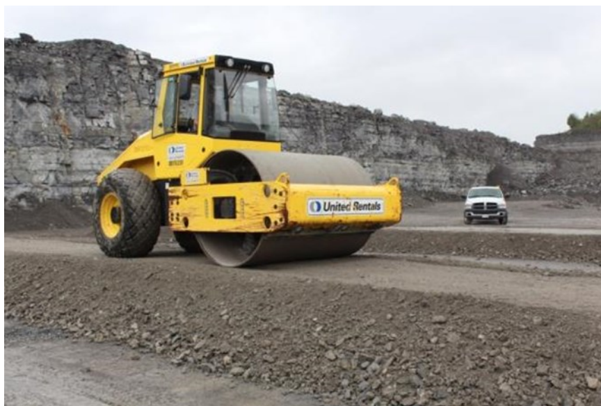
Figure 4-2. Test pad at Quarry 1 undergoing vibratory compaction
