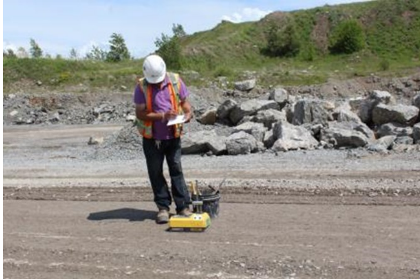
Figure 4-4. Nuclear densometer testing in progress at Quarry 2
