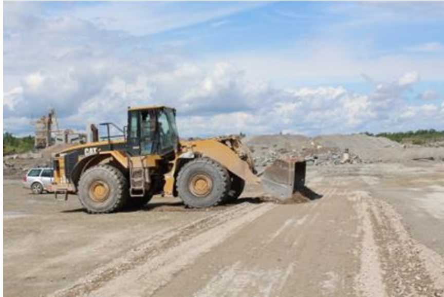
Figure 4-6. Test pad sampling at Quarry 2 using a front-end loader
