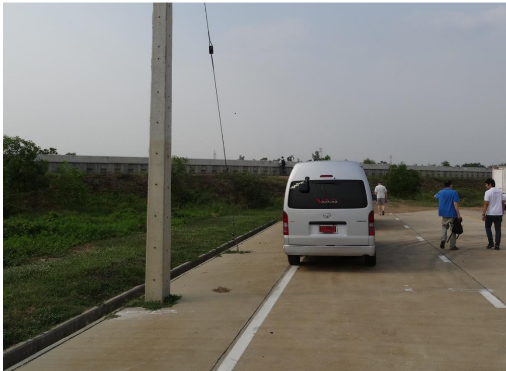
Figure VIII: Industrial Sector Adaptation to Flooding. This industrial estate has built an approximately 2.0m earthen berm topped with an approximately 1.0m concrete wall. The estate also improved its pumping capacity. The 2011 flood line is visible approximately 2.5m up the power pole.
