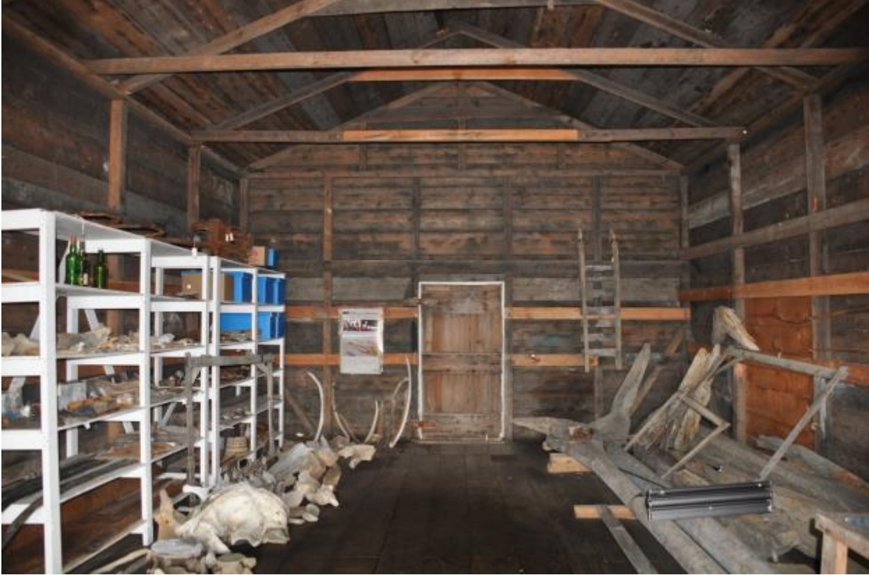
Figure 12: Photograph showing interior of the main section of the Bone Shed where Alikomiak and Tatamigana were hanged. At the time of the hangings, the portable gallows would have been built under the joists. The platform of the gallows would have held the prisoners and hangman, and required a sturdy overhead beam (the roof joist in this case) and enough clearance to allow the body to hang. 145 Rumour has it, that when the RCMP left the Island in 1965, they cut down the beam from which Alikomiak and Tatamigana were hanged, and burnt it. 146 The walls of the bone shed began to splay outward due to the lack of support, and the gap in the beam was repaired, not fully replaced a number of years ago. This photograph clearly shows the new wood used to repair the beam. Photographs of all the buildings on Herschel Island are taken every year to document their condition. This photograph was taken in summer 2015. Photo courtesy of Brent Riley Historic Sites and Restoration Planner, Government of Yukon Tourism and Culture, Cultural Services Branch and used with permission.
