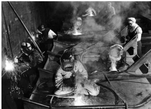
Figure 2: World War 2 welding application of shielded metal arc welding (SMAW) process [4]
