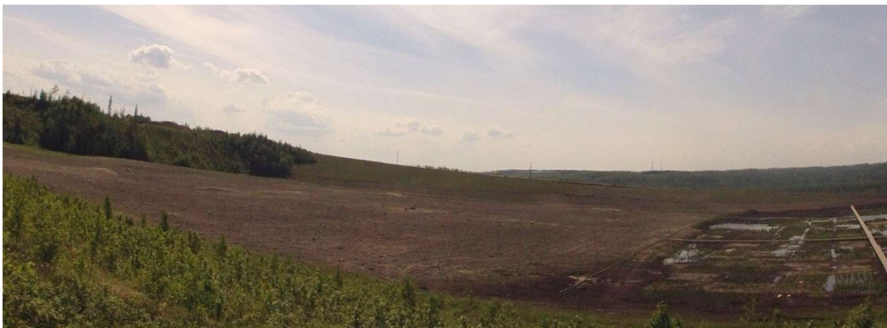
Figure 1 – 3 Photo (2014) of the Nikanotee Fen watershed. The constructed upland sloping towards the fen. Note that the wide-angled lens used exaggerates the true slope of the upland (2% grade).
