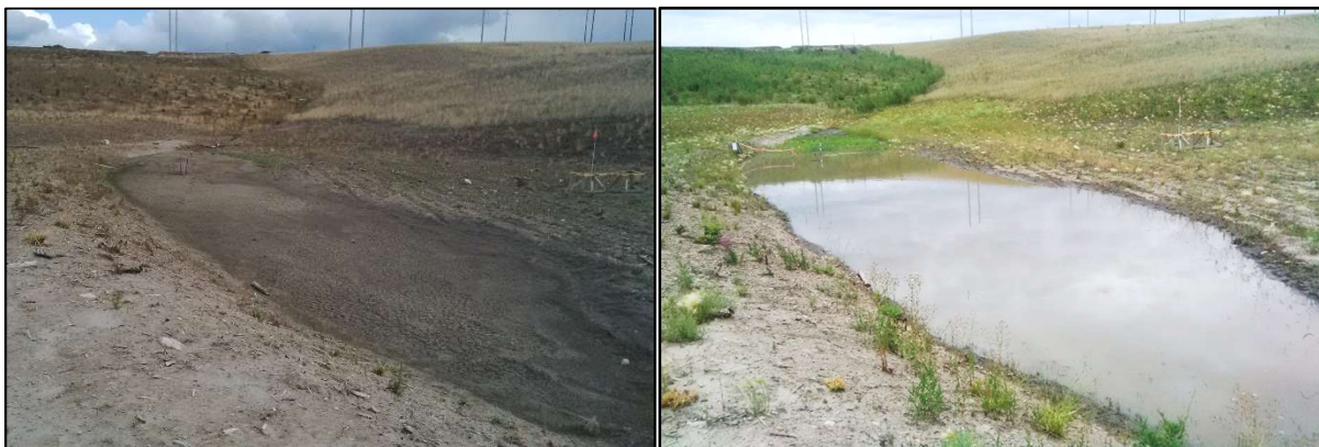
Figure 3 – 3 East recharge basin empty (left) and full shortly after a large rain event (right).
