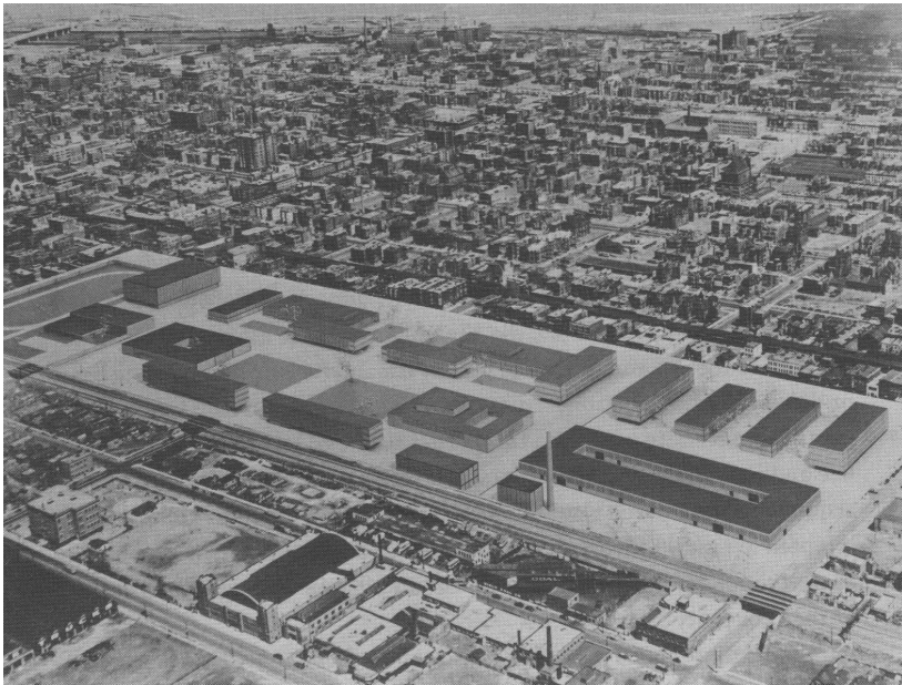
fig. 3.15 Aerial view of IIT Campus in relation to surrounding city context
