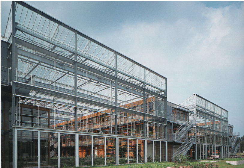
fig. 4.119 Greenhouse structures forming atria between laboratories and educational buildings, Institute for Forestry and Nature Research in Wageningen University
