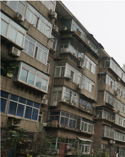
fig. 4.121 Loggia enclosed by sliding glass windows in danwei housing
