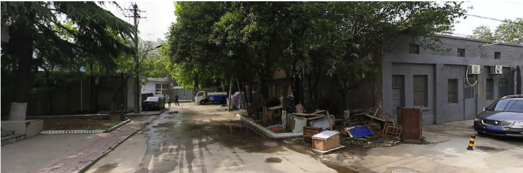
fig. 4.68 View south towards the dead end of Jiaoxue East Road showing the neglected state of single-storey printing company buildings to the right
