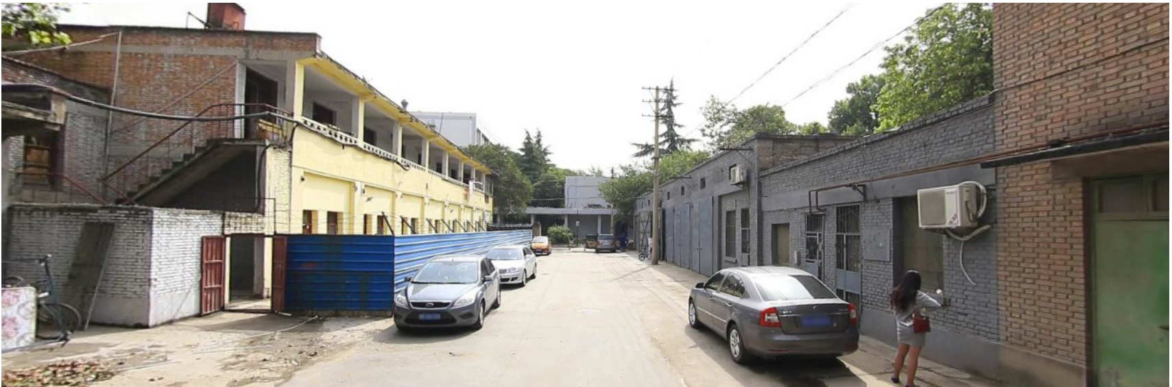
fig. 4.70 View east of low-density buildings in the printing company laneway
