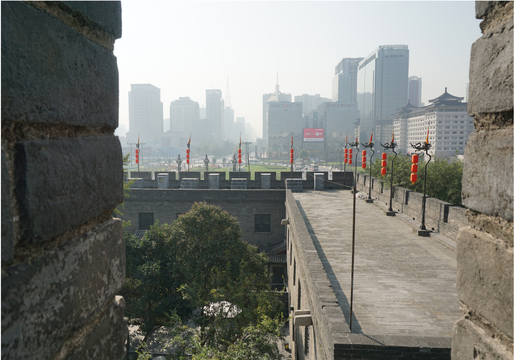
fig. 4.12 View of the outer city skyline from within the inner city wall
