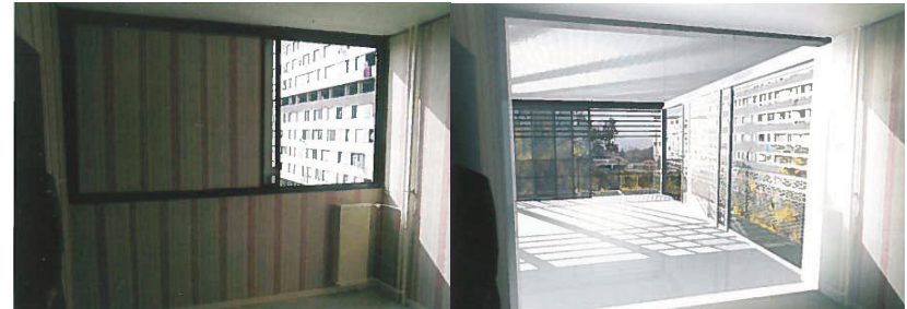
fig. 1.10 Loggia used by Lacaton & Vassal to extend living spaces in existing social housing
