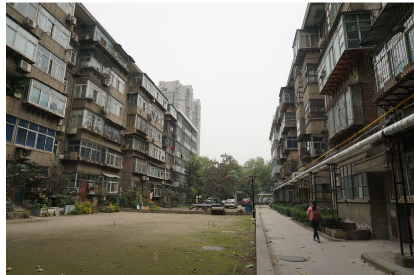
fig. 4.22 Socialist-era employee housing inside the Jiaotong University hospital danwei with un-insulated enclosed loggia extending from the exterior wall
