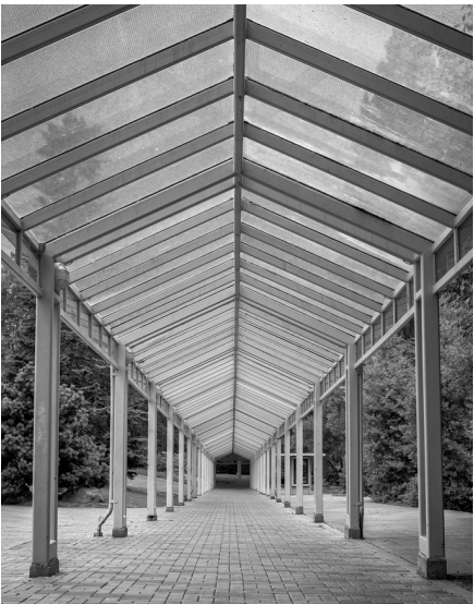
fig. 4.122 Covered walkway in the Seattle Center
