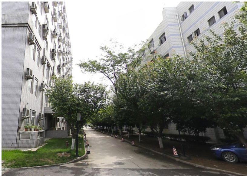
fig. 4.62 View east of tree-lined road between the medical library to the left and finance teaching building to the right
