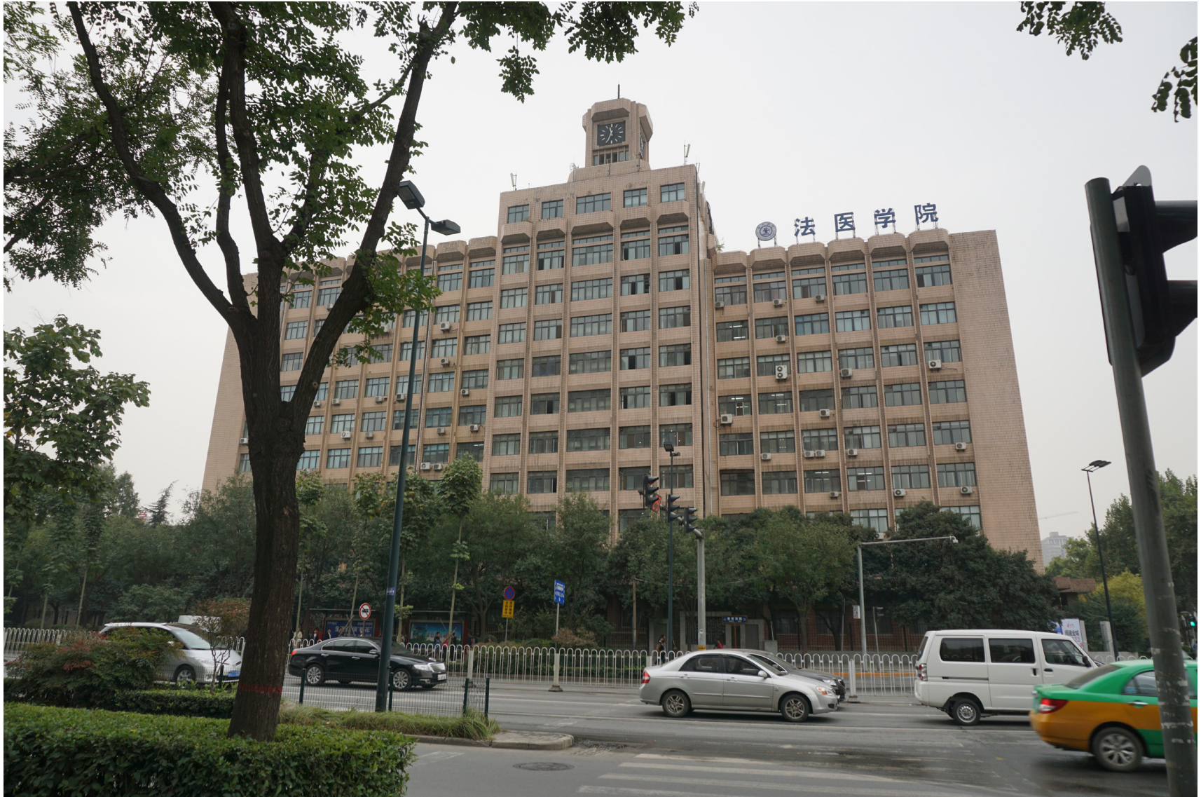
fig. 4.48 View from Yanta West Road of the forensic medicine building with clock tower in the northwest corner of the campus danwei
