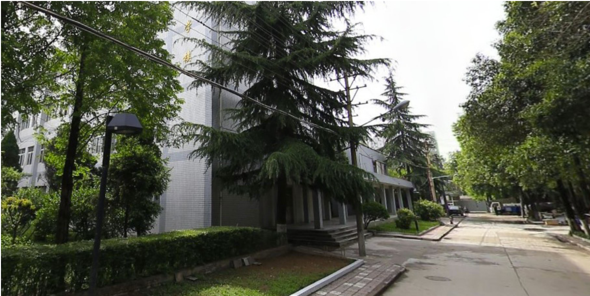
fig. 4.67 View south along Jiaoxue East Road of pharmacy teaching and training building
