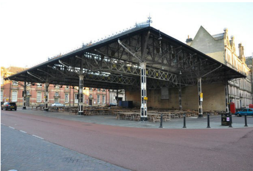
fig. 4.118 Use of the large spanning roof in Preston Covered Market, Lancashire, U.K.
