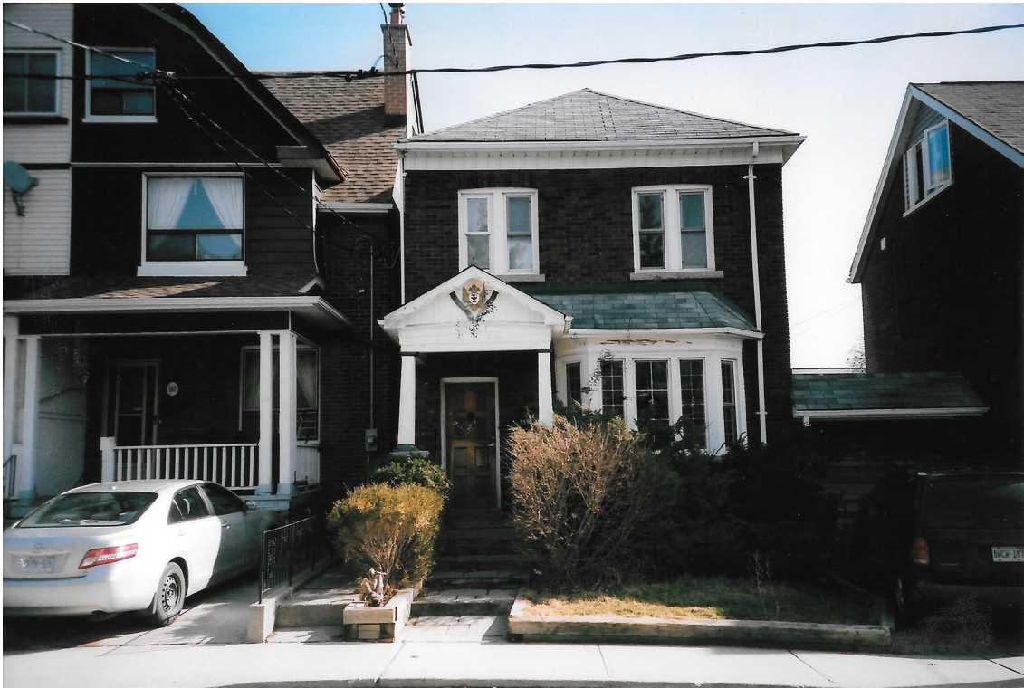
fig. 2.63. Entry 1.55 196 Manning | 196 Manning Ave. | Defunct | 2005
