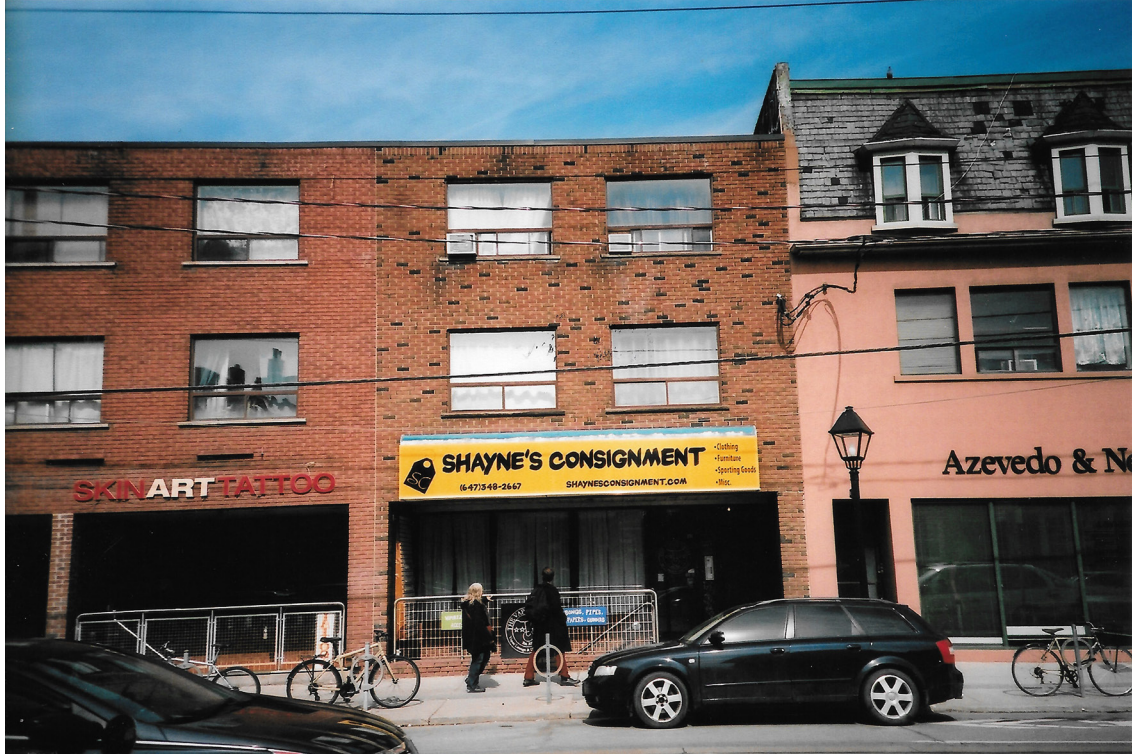
fig. 2.60. Entry 1.52 Faith / Void | 894 College St. | Operational | 2015-
