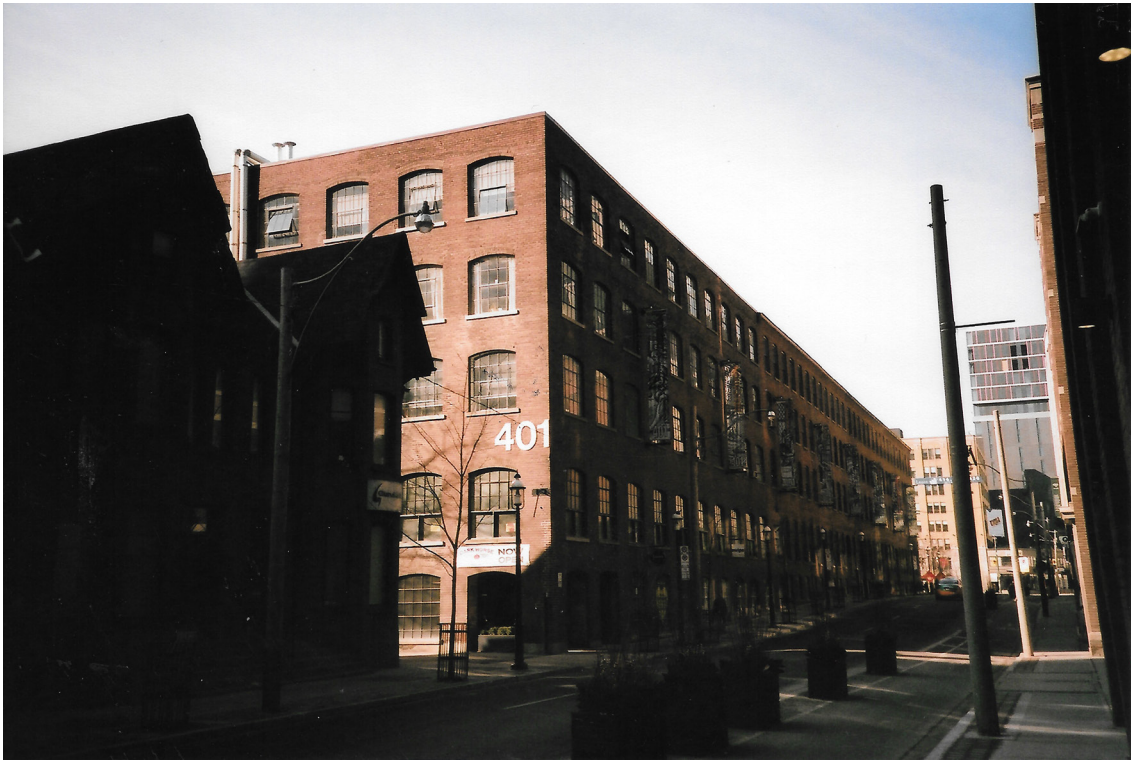
fig. 2.41. Entry 1.35 401 Richmond | 401 Richmond St. W. | Operational | 1994-
