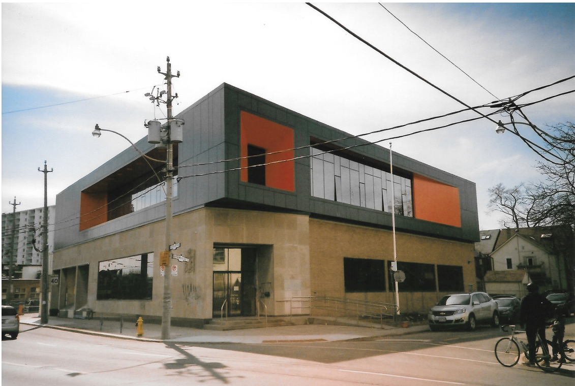
fig. 2.15. Entry 1.10 Common Cause | 772 Dovercourt Rd. | Operational | 2007-
