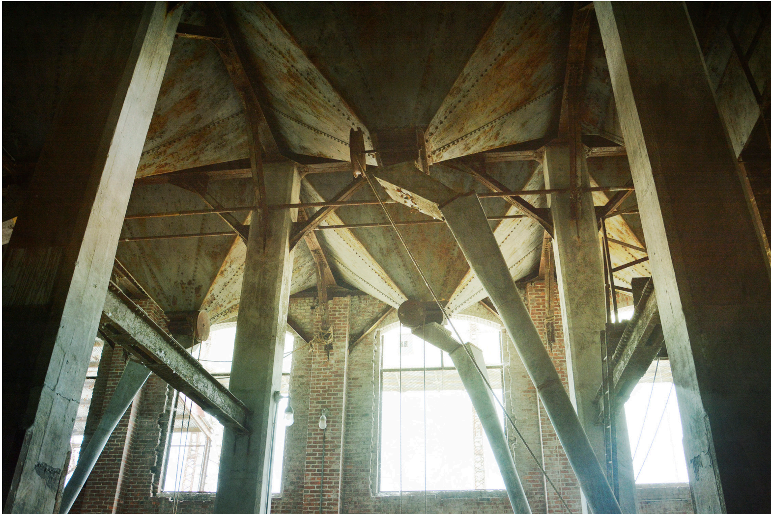
Figure 2.73: Interior of the steel grain elevator
