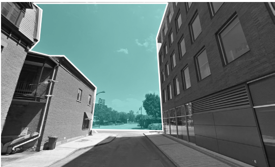
Figure 3.55: View to the silo complex from Rue Prince
