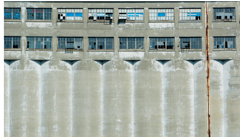
Figure 2.48: Silo No. 5 concrete facade
