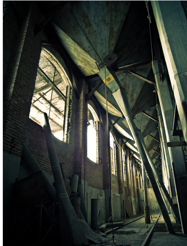
Figure 1.1: Image from the ground floor of the steel grain elevator in the Silo No. 5 complex
