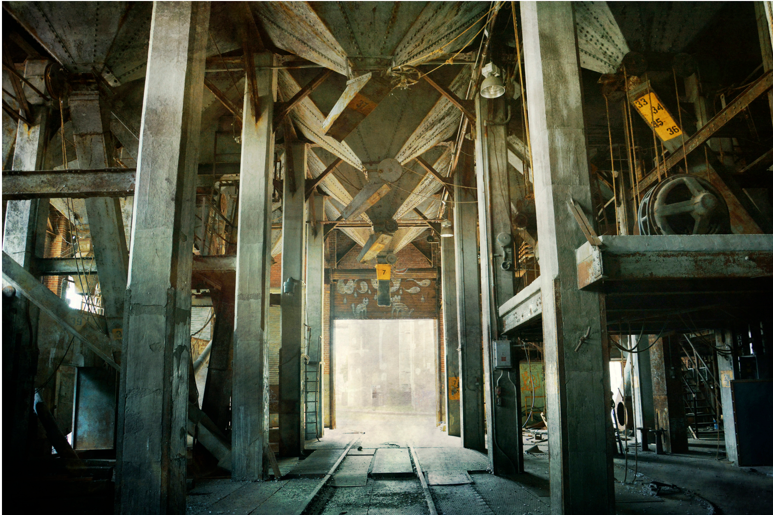
Figure 2.74: Interior of the steel grain elevator
