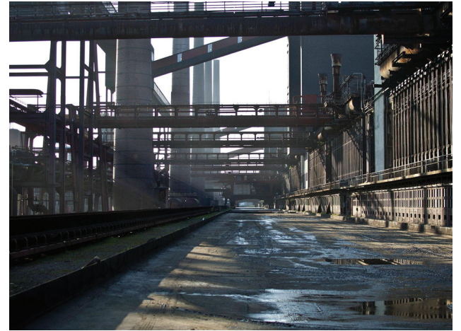
Figure 1.4: Steel mill in the Ruhr area, Germany
