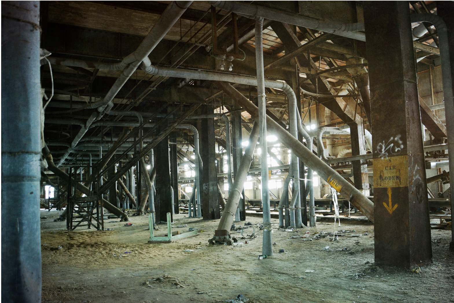
Figure 2.81: The interior of the upper galleries in Elevator B
