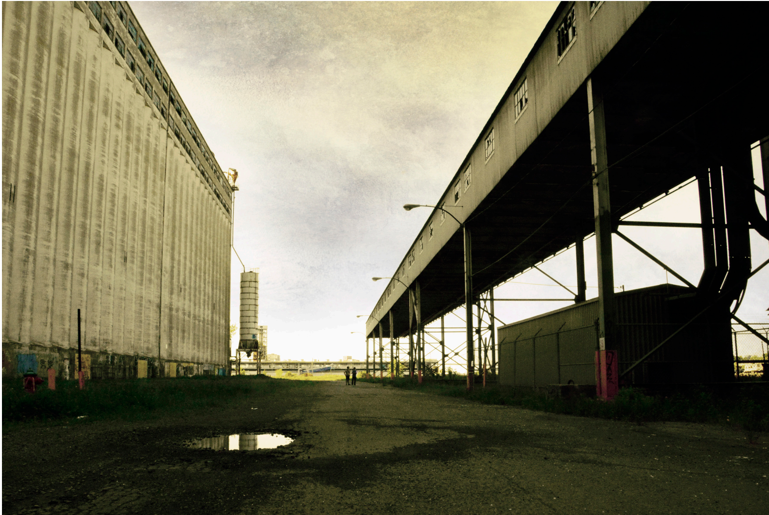
Figure 2.72: View from inside the complex, looking the opposite way
