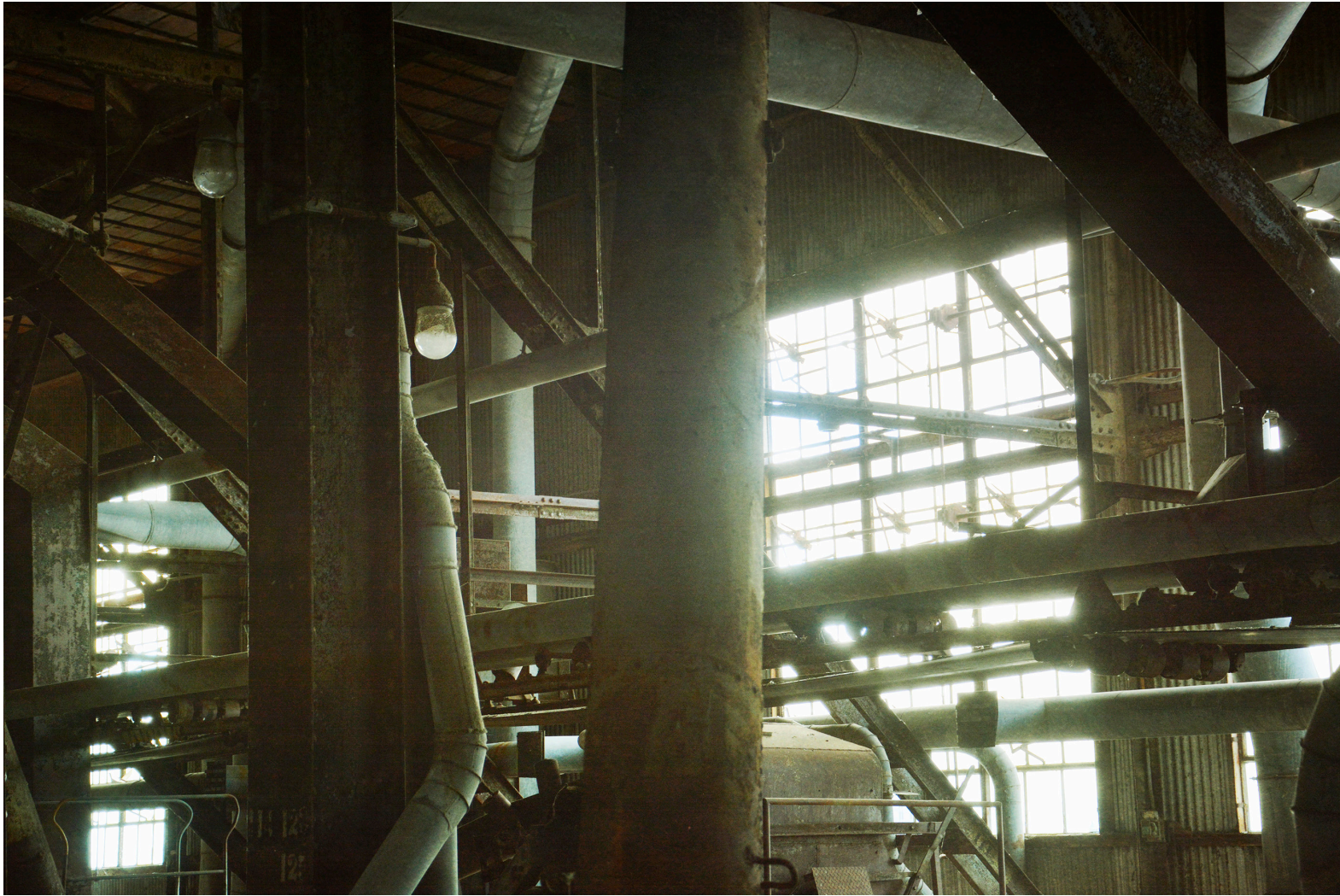
Figure 2.80: The interior of the upper galleries in Elevator B
