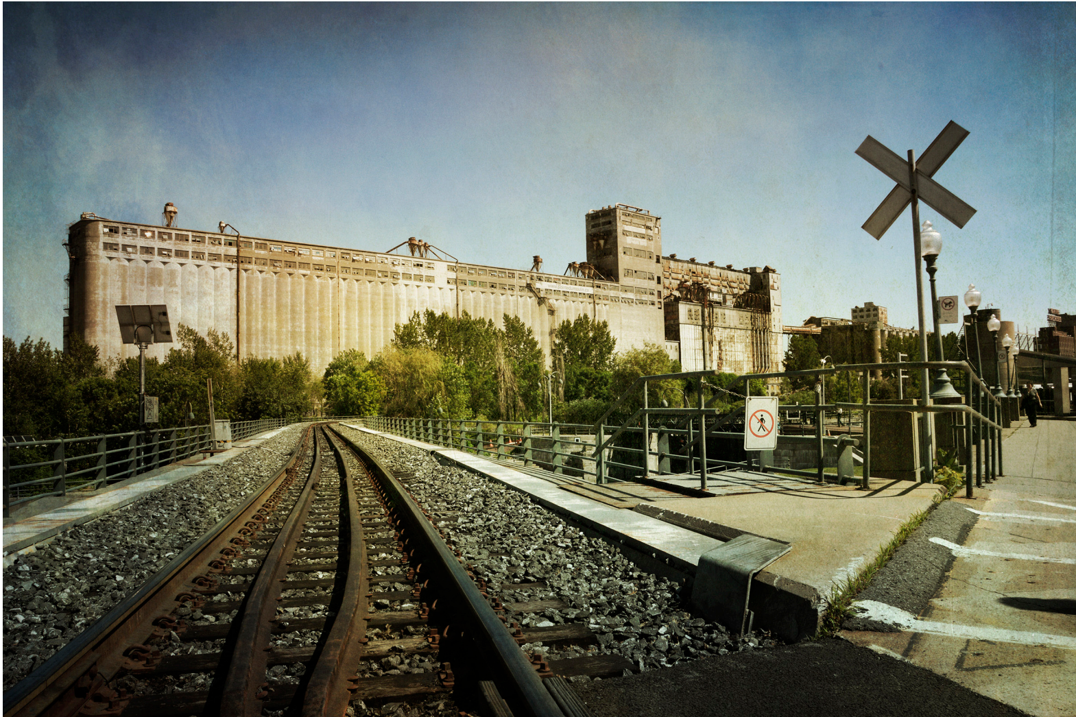
Figure 2.67: Walking along the train tracks towards the site
