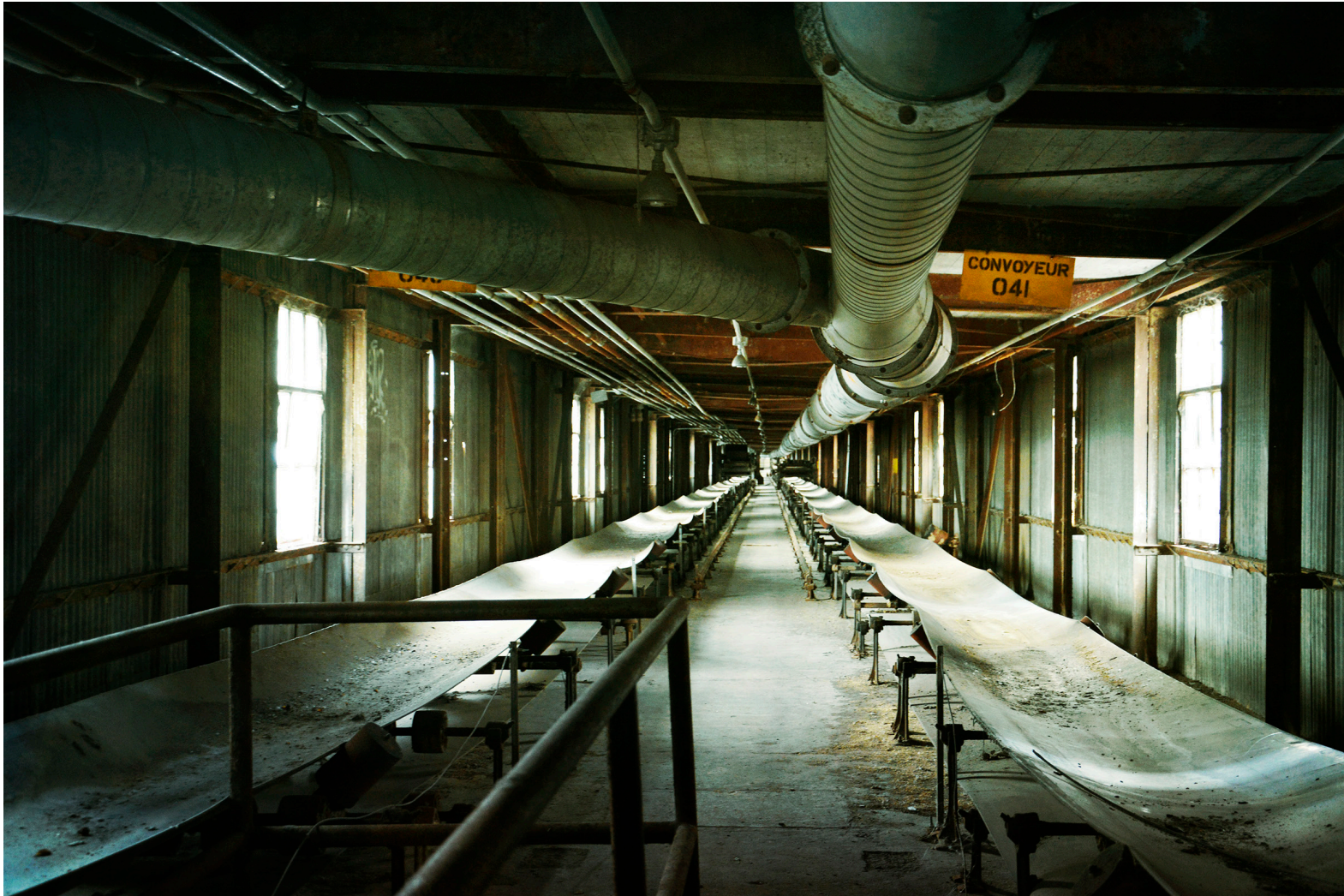
Figure 2.75: The interior of the elevated conveyor galleries
