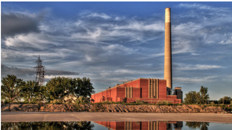
Figure 3.37: Exterior of the Power Plant
