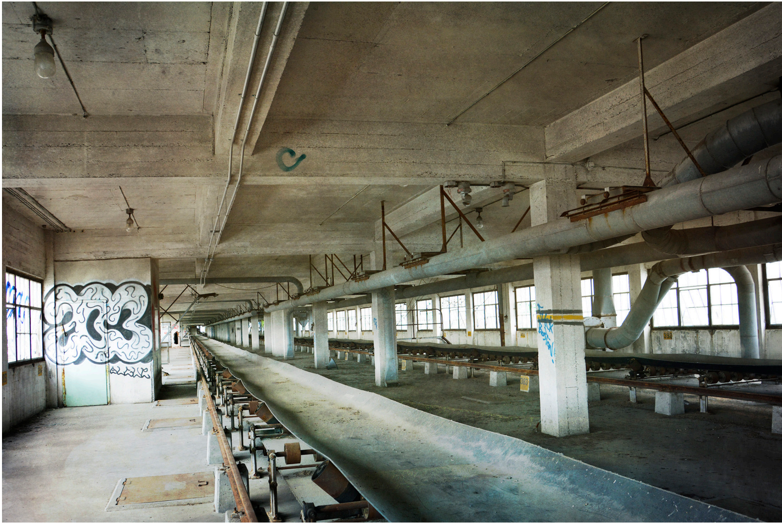
Figure 2.78: Interior of the upper galleries
