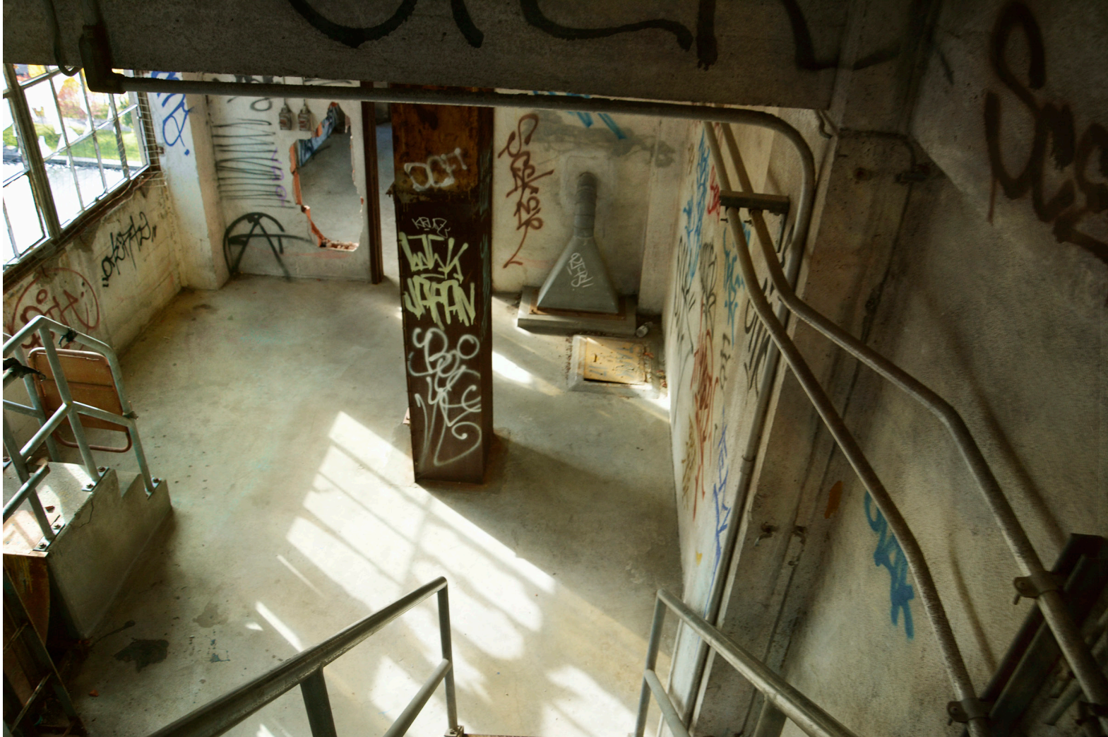
Figure 2.77: Interior of the tower
