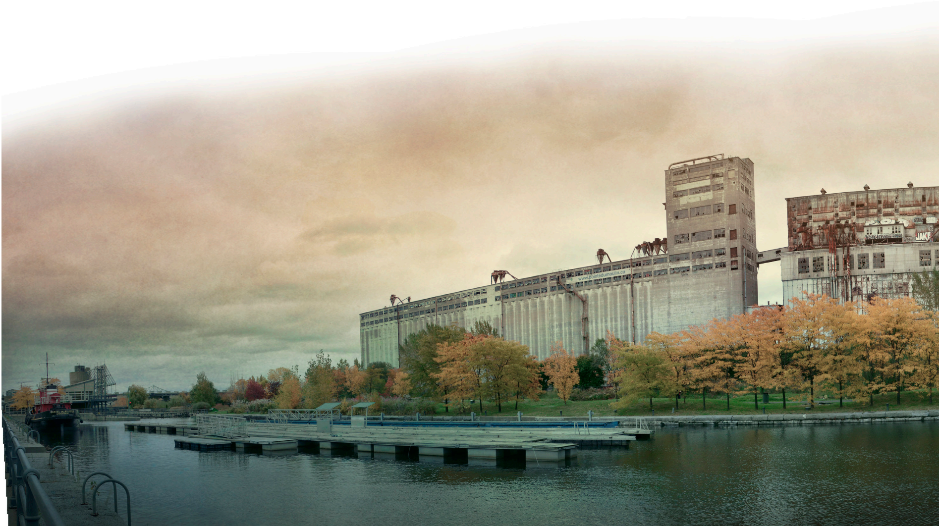
Figure 2.66: Panorama of Silo No. 5 and its surroundings
