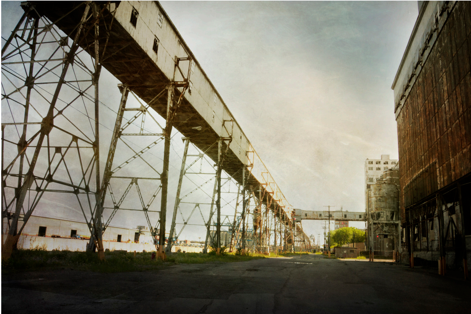
Figure 2.71: View from inside the complex, walking along the elevated conveyor galleries
