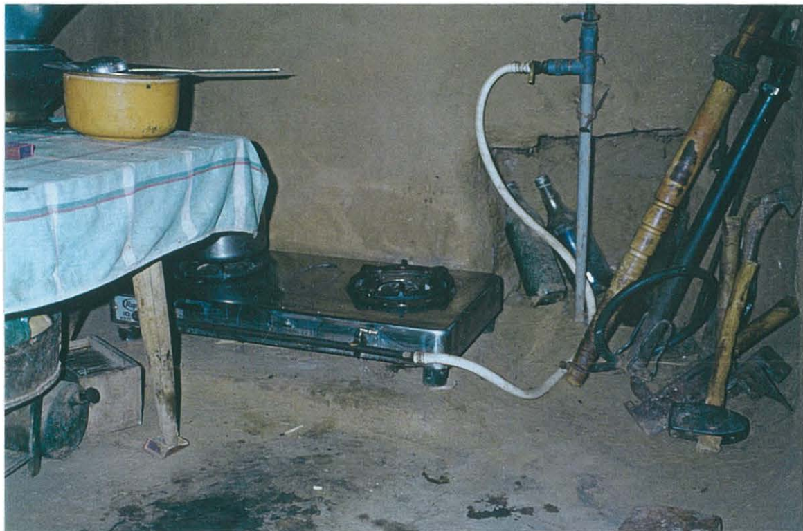
Figure 6.13 - Biogas Stove
