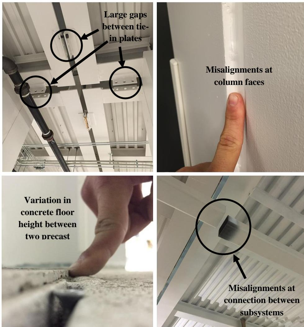
**Figure 5: Dimensional variability challenges faced in a modular construction project.**
