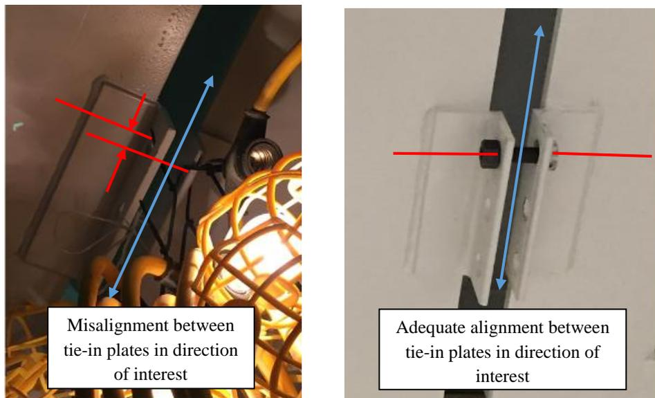
**Figure 67: Depiction of misalignment of tie-in plates (left), and adequate alignment (right). Red arrows indicate deviation associated with misalignment, while blue arrows indicate direction of interest.**
