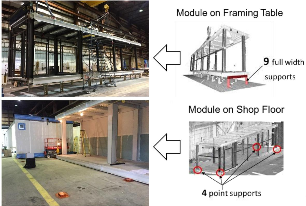
**Figure 45: Temporary support conditions for the module. Top left and right: module sitting on the BLUCO® framing table. Bottom left and right: cribbing on the shop floor.**
