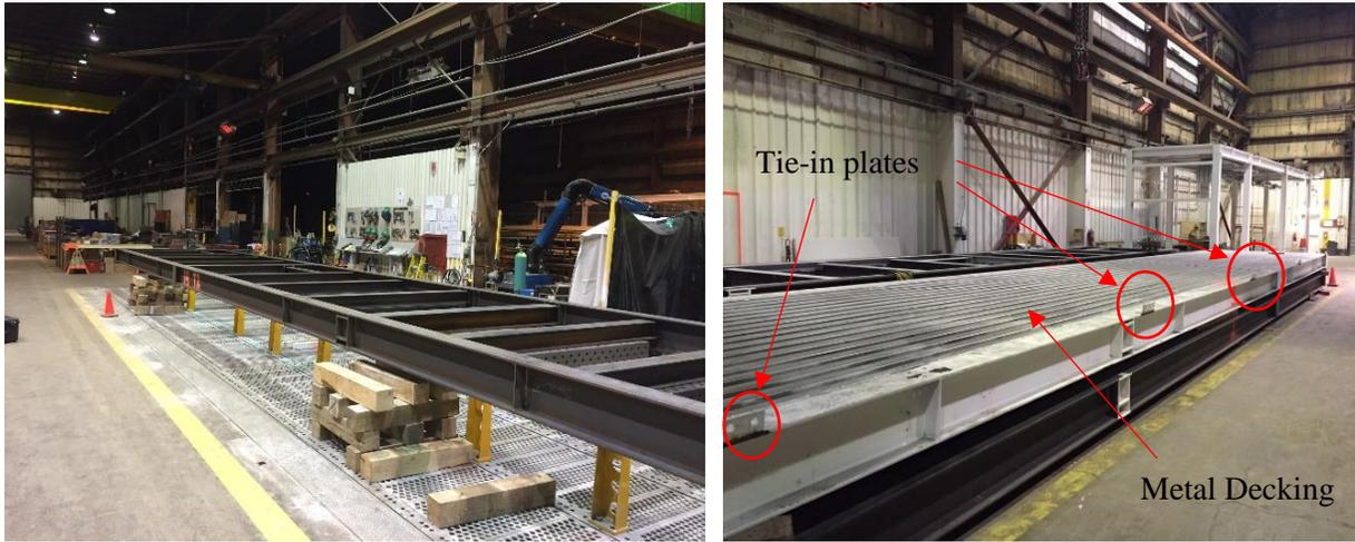
Figure 36: Left: Standardized roof frame on framing table. Right: Installed corrugated metal decking and tie-in plates.
