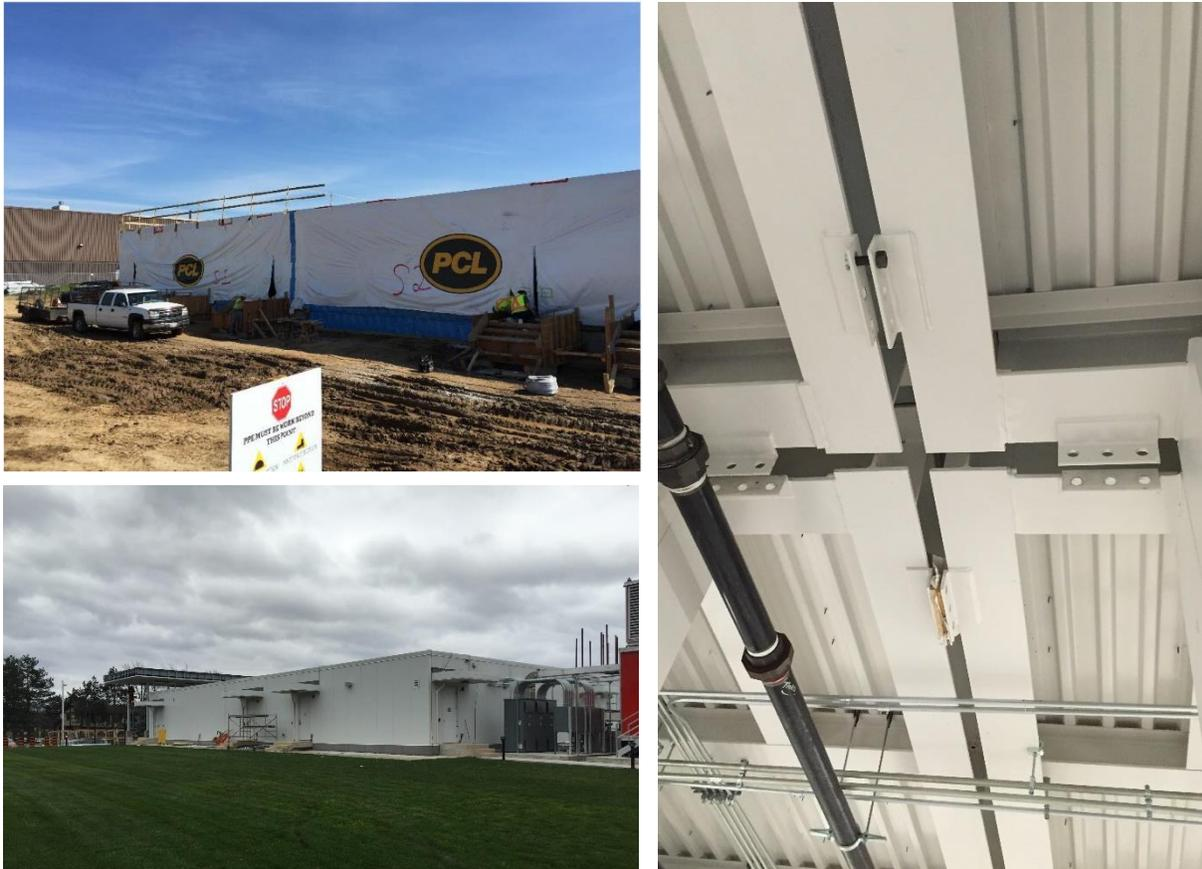
**Figure 55: Examining the dimensional variability associated with erection loads. Top left: project site, where modules are first brought into rough alignment, and then subsequently connected together at the tie-in plates. Bottom left: project site after completion of all construction activities. Right: demonstration of the amount of large gaps between modules at tie-in plate locations as the result of the accumulation of dimensional variability.**
