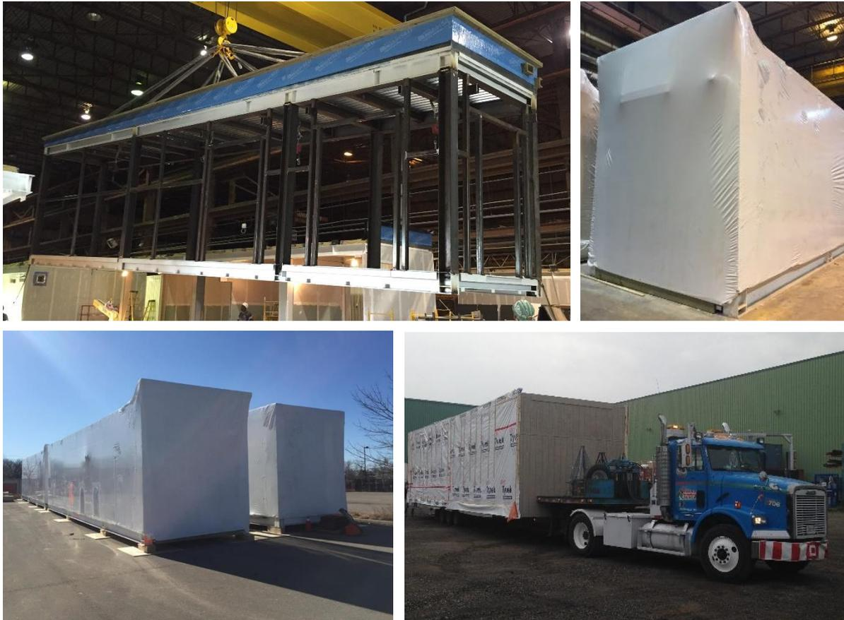
**Figure 52: Analysis of the effects of different load conditions. Top left: module being lifted by a crane during the fabrication of the module. Top right: module before transportation. Bottom left: module after transportation to a temporary storage facility. Bottom right: truck used to transport modules to and from the shop, temporary storage and the project site.**
