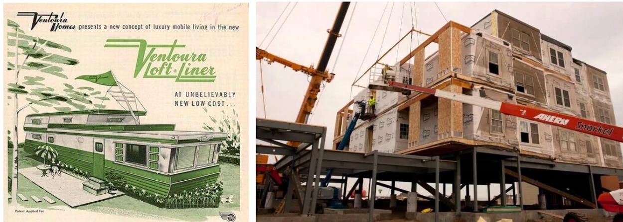
**Figure 1: Example of 1960's prefabricated construction: single-wide mobile manufactured house (left). Example of a modern modular construction project: modular apartment building (right). (Catpal 2013, Champion 2013)**
