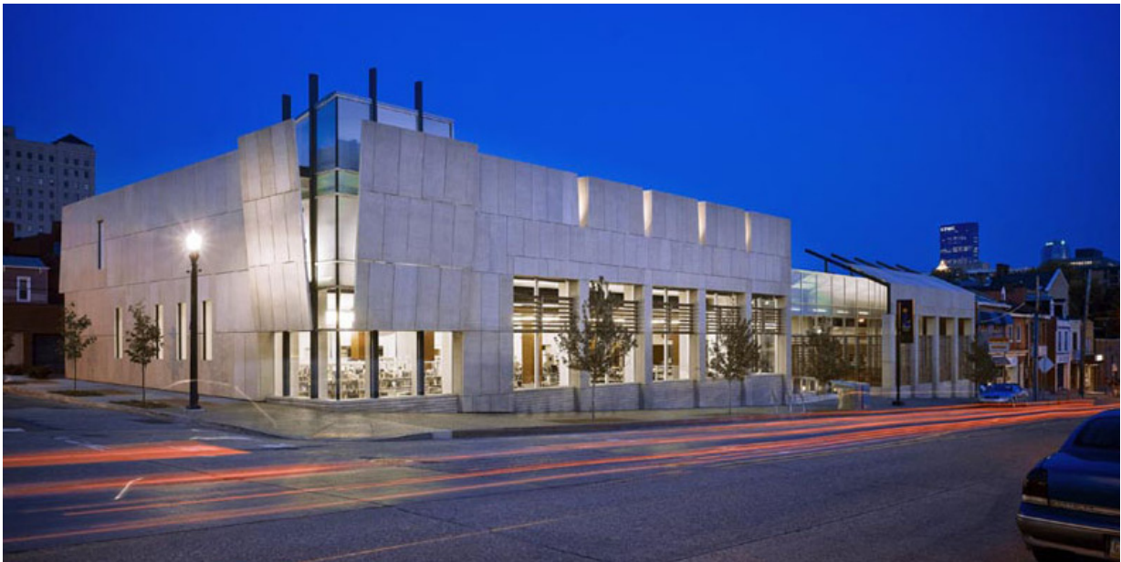
Fig. 1.4 - The new Allegheny Branch of the Carnegie Library of Pittsburgh network was built in 2009 to replace the original Carnegie Library that had been in operation since 1890.
