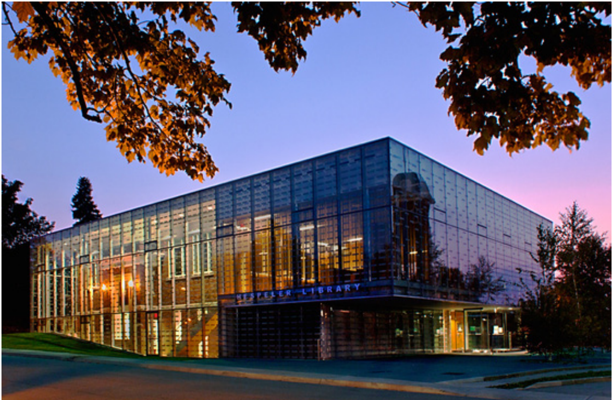
Fig. 5.3.2 - The Hespeler Public Library expansion project created a very innovative solution to the problem of space facing Carnegie Libraries around the world by enclosing the original library within a new building shell.
