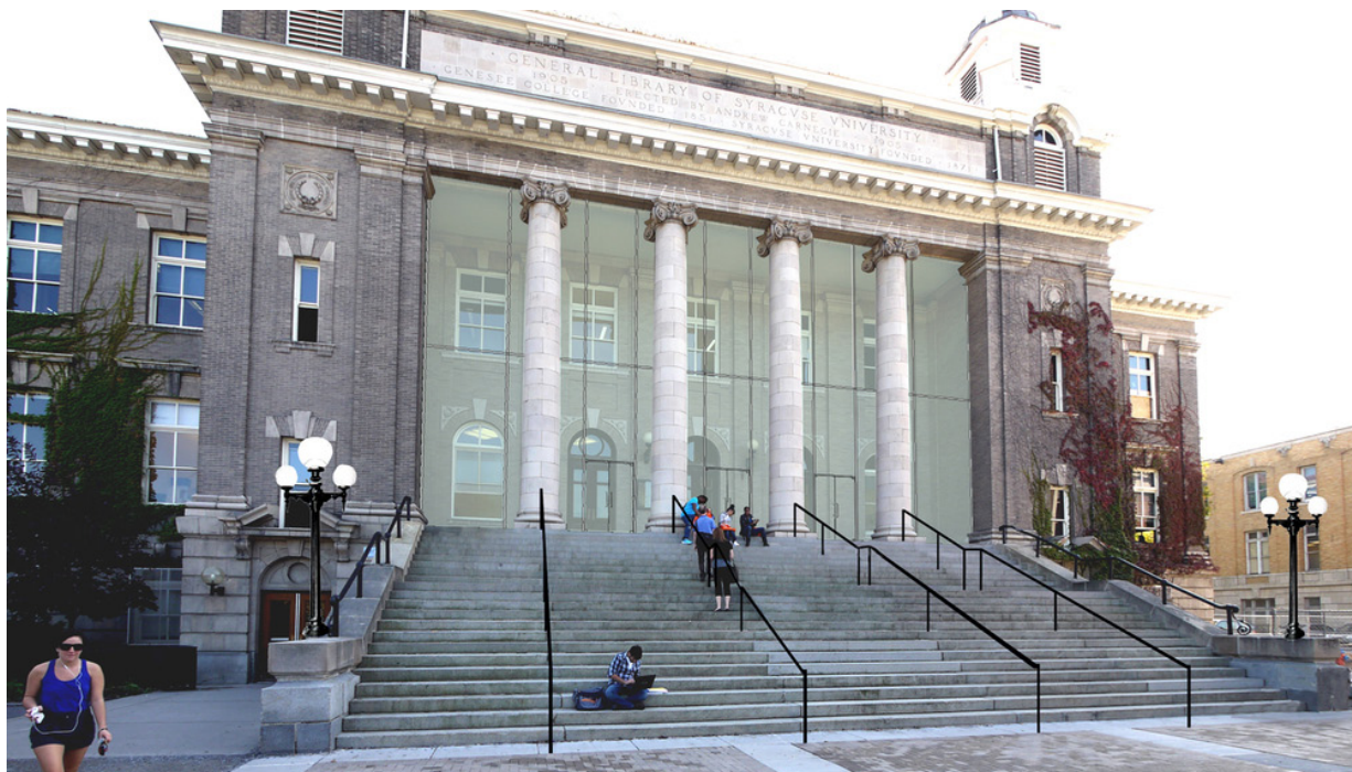
Fig. 5.6.2 – The newly restored façade of the University of Syracuse Carnegie Library with its newly enclosed portico as an entrance vestibule.
