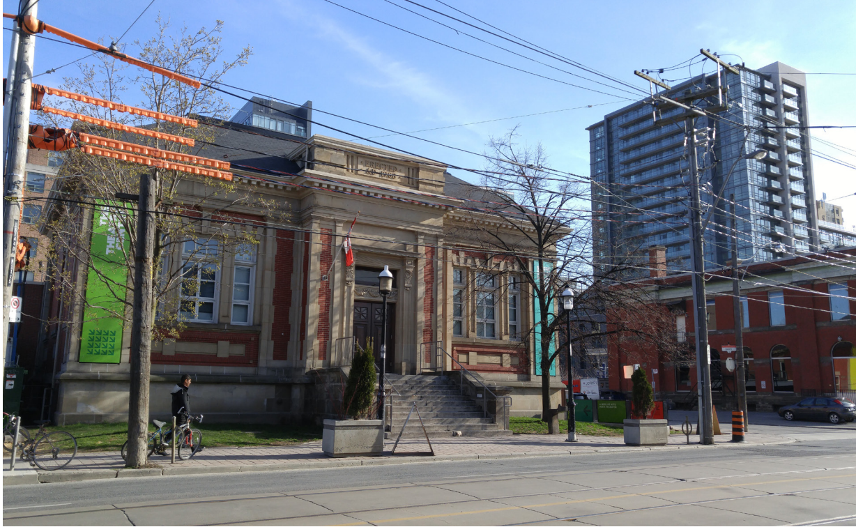
Fig. 7.1.7 - The former Queen and Lisgar Branch Library, currently in use by The Theatre Company as a performance space, sits in the rapidly developing neighborhood of West Queen West in Toronto.
