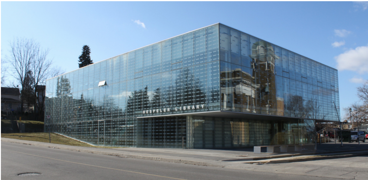
Fig. 2.5 - The Hespeler Public Library in Cambridge, Ontario used a unique strategy to facilitate its own revitalization by designing a glass building around their original Carnegie Library, doubling the usable space of the library while completely preserving the architectural integrity of the original building.
