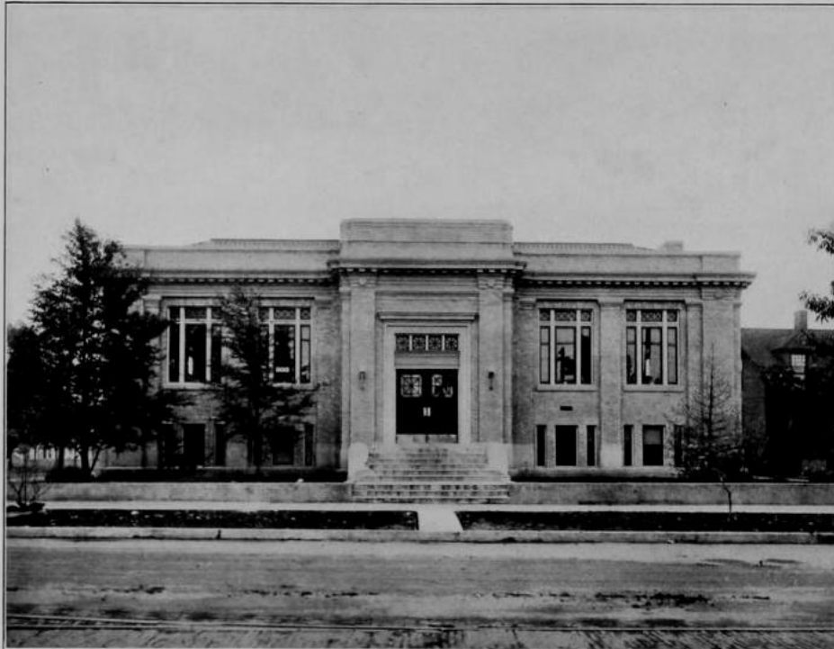
Salem Public Library, Salem, Oregon George M. Post, Architect
