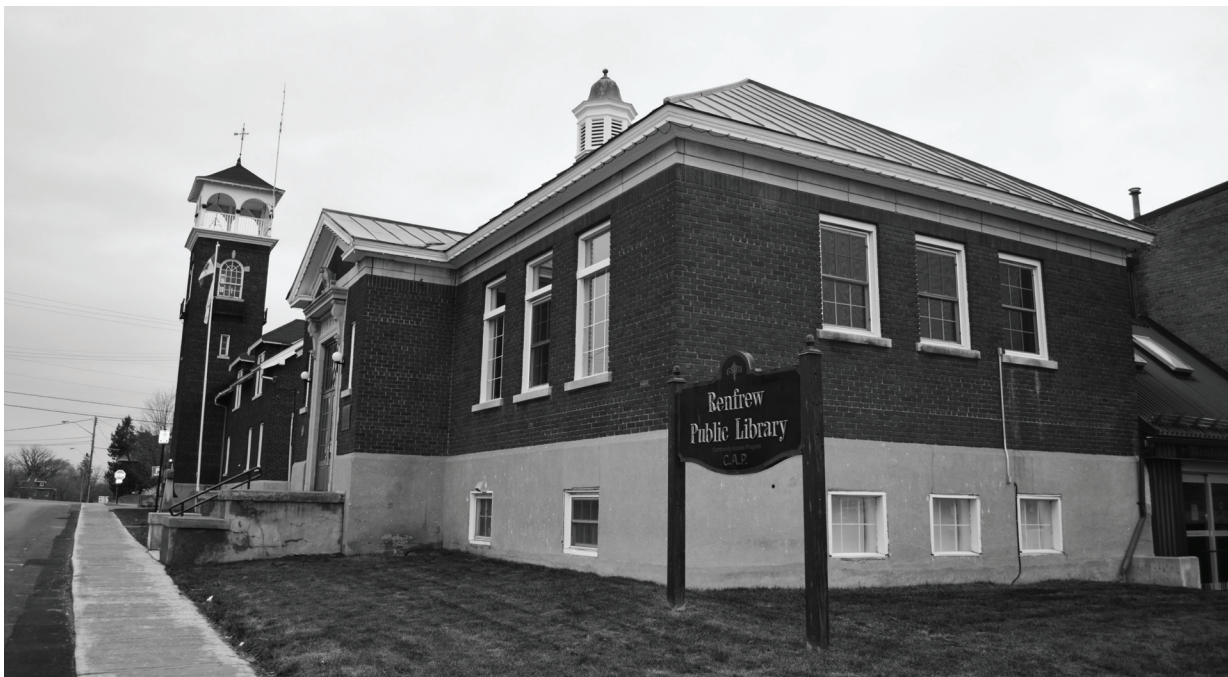
Fig. 4.1.1 - The Renfrew Public Library's site is a perfect example of the type of prominent site Carnegie preferred communities to select as it is located next to the fire station (left) and city hall (not pictured) at the exact center of the town.
