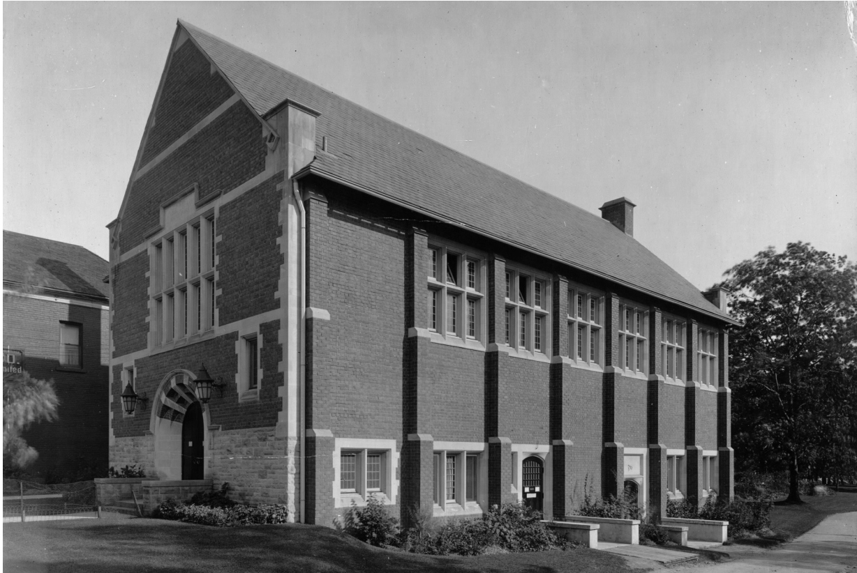
Fig. 5.1.1 - The original Beaches Branch of the Toronto Public Library after it was completed in 1916.
