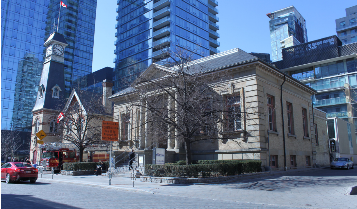
Fig. 2.4 - The Yorkville Public Library, one of Toronto's most prominent operating Carnegie Libraries, placed a subtle addition on the back of the building to facilitate digital technology integration while allowing for the original portion of the library to continue to house books and reading spaces.
