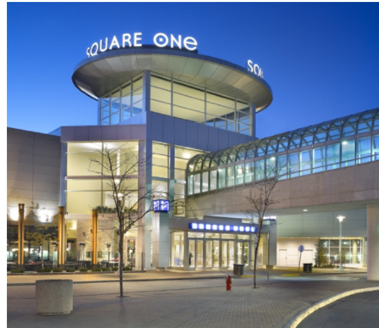
Figure 3.29 Square One SE entrance with bridge to parking structure
