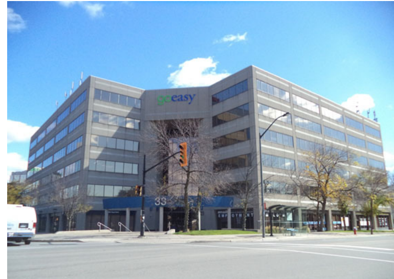
Figure 4.17 1977 Office Building at 33 City Centre Drive
