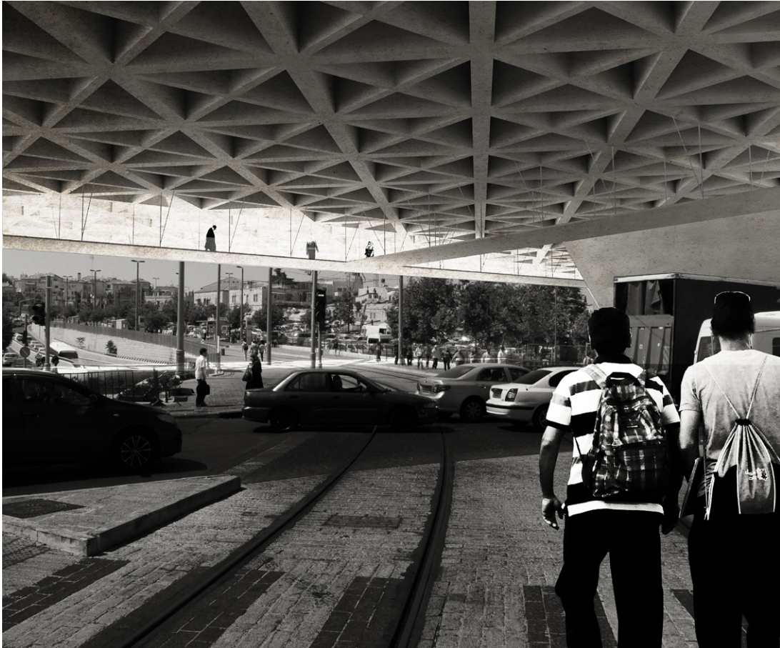
Fig. 3.55 Image depicting the roof passing over Road 60, and the system of overhead walkways suspended from it.
