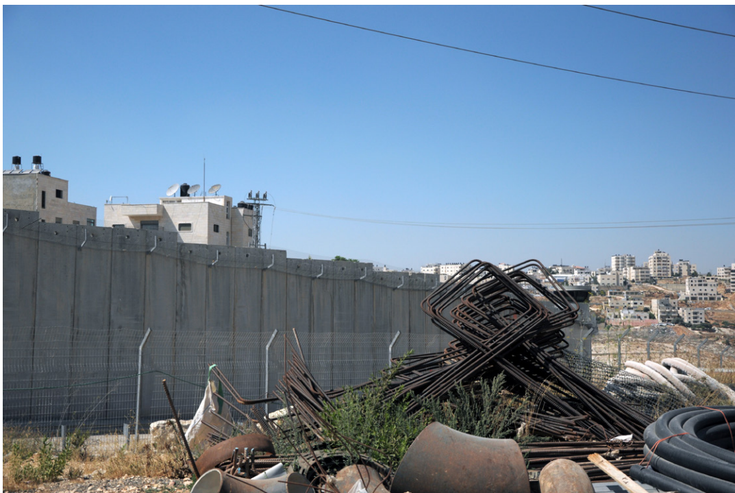
Fig. 1.11 View of the Separation Wall from a construction site in Neve Ya'akov, a suburban development in north - east Jerusalem, . The community of Ar - Ram can be seen behind the wall. Photo taken by the author.
