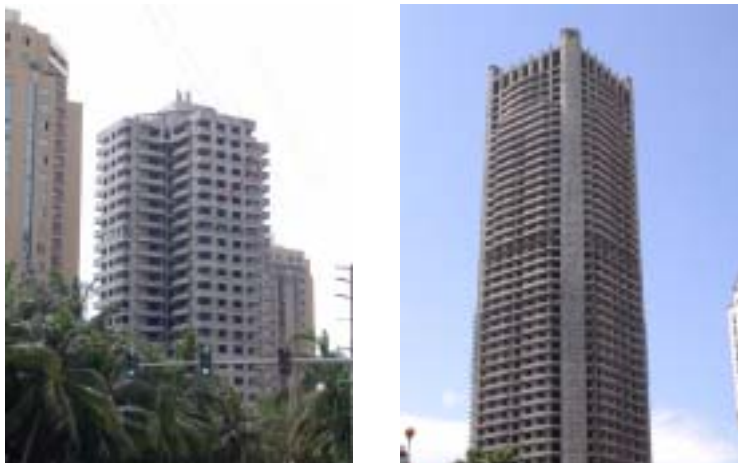
Figure 4-4 Unfinished and abandoned housing in Haikou (Photographs taken by the author, left: 07/02/2005, right: 07/16/2005)
