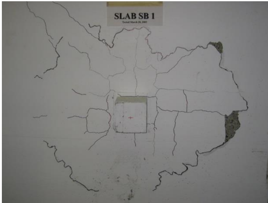
Fig. 5.14. Ultimate load cracking pattern at the bottom of the slab SB1: Test results (scanned from Adetifa and Polak 2005).
