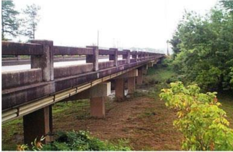
Figure A.3. Straight, RC T-Beam Bridge
