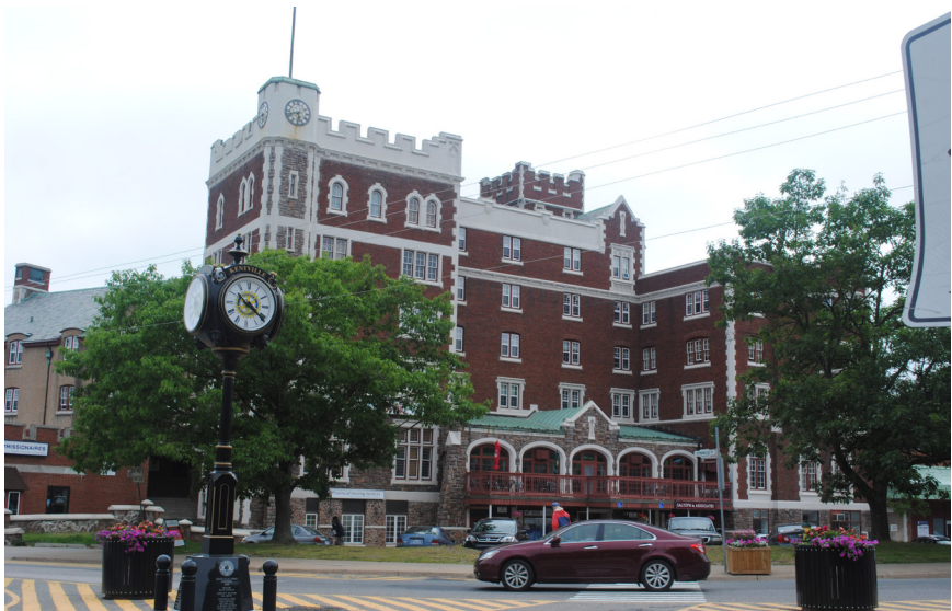
Fig. 3.1.12 - The Cornwallis Inn, formerly a railway hotel, is now apartments
