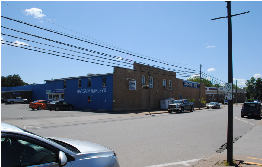
Fig. 4.3.3 - Commercial Street retail
