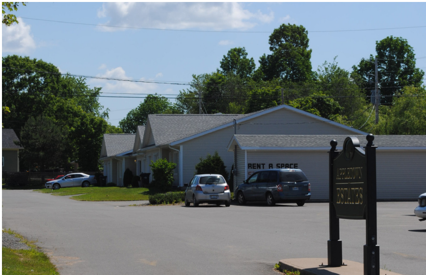
Fig. 4.3.2 - Small-scale apartment buildings off Commercial Street
