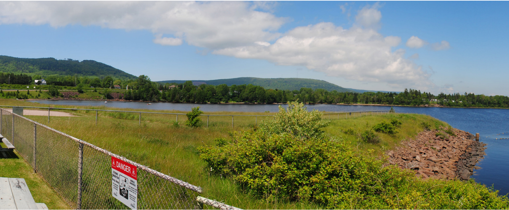
Fig. 2.2.1 - View upstream at Annapolis Tidal Generating Station
