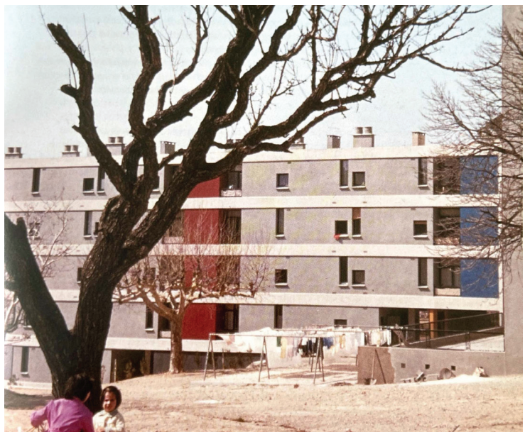
La Viste project (700 low rent dwellings), in Marseilles' suburbs, 1959, CWJ.
