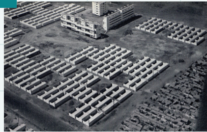
\ Muslim housing for Moroccan workers coming from rural areas \ 64 m 2 units, following the 8 m x 8 m grid
