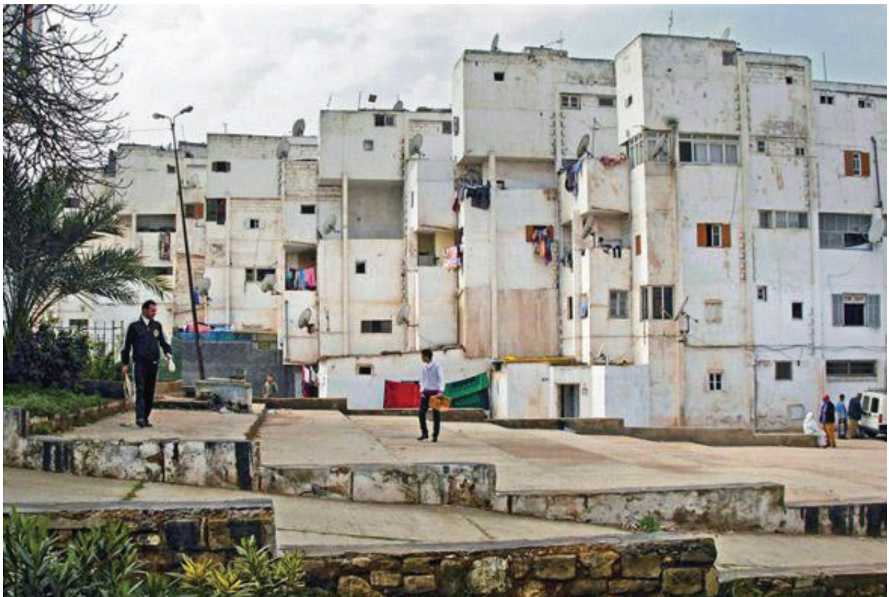
NOW: The Habitat Marocain in Sidi Othmane building, Sidi Othmane, Casablanca, 2013. Similarly to the outcome of the HCB, inhabitants of HMSO have closed-up the balconies and filled up the space underneath those with additional rooms as their needs in space evolved. Photograph: Marion von Osten
