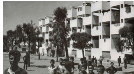
Figure 32 The Honeycomb building in the 1980s.
