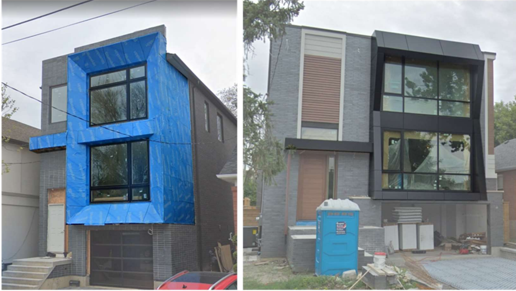
Figure 28: Recent Residential Construction Projects in Toronto, Ontario with Aluminum Exterior Panel Systems (photos obtained from Google Maps)
